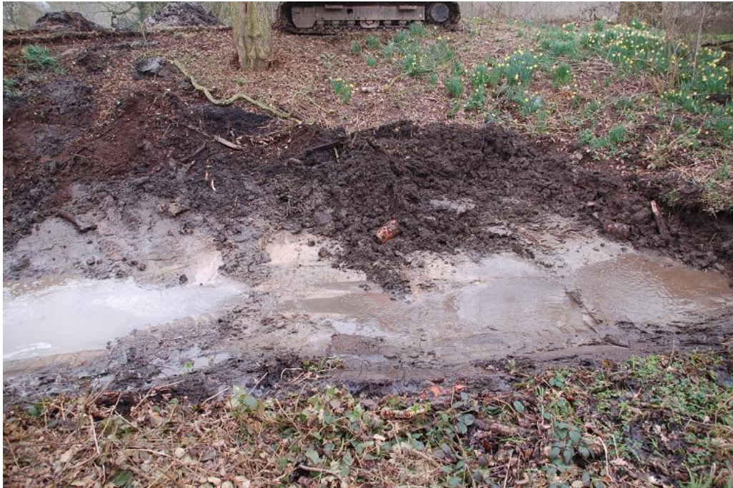
Plate 1 Excavation of pond 1 illustrating presence of modern drainage pipe
