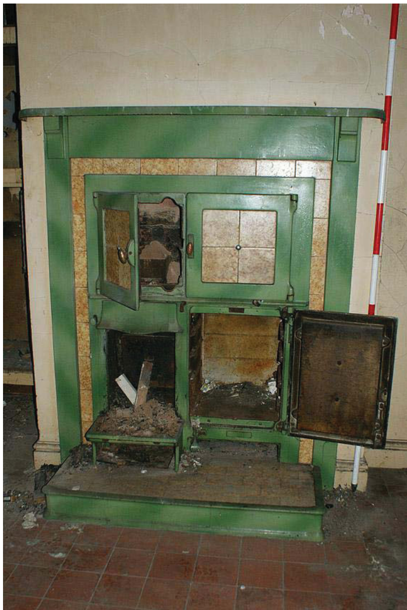
Plate 34: Triplex Grate, C Pattern, within 2 nd floor flat
