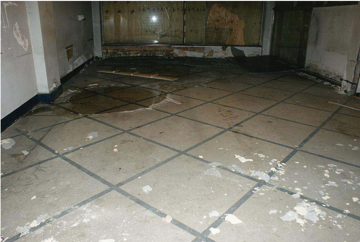
Plate 25: 1940s decorative flooring on ground floor of building
