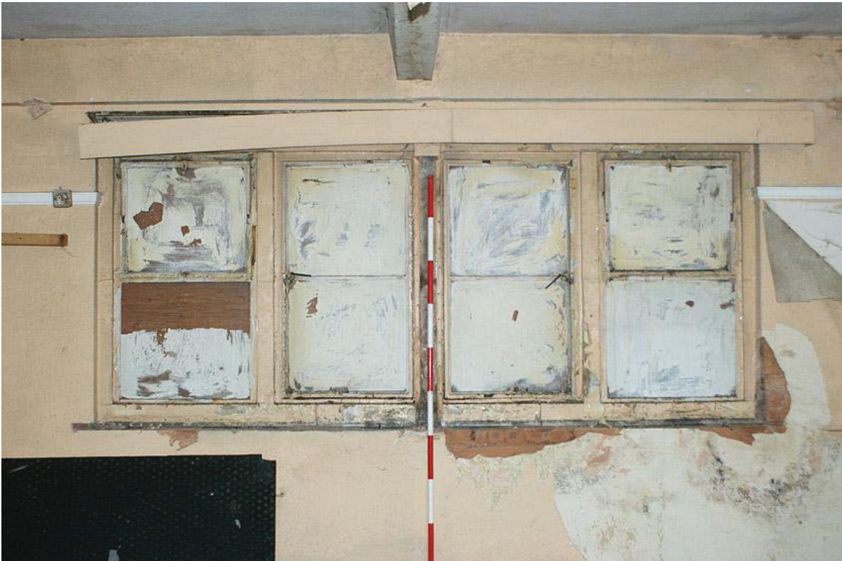
Plate 31: Original windows within 2 nd floor flat
