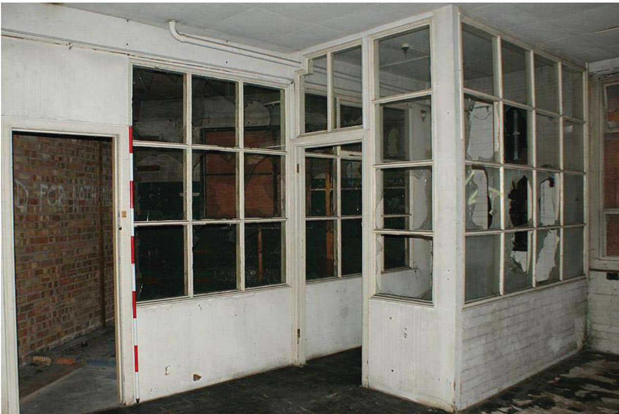
Plate 37: 1940s office partition on first floor
