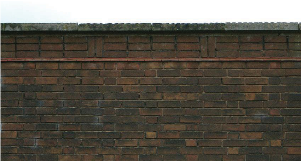
Plate 15: Decorative brickwork and concrete coping of parapet
