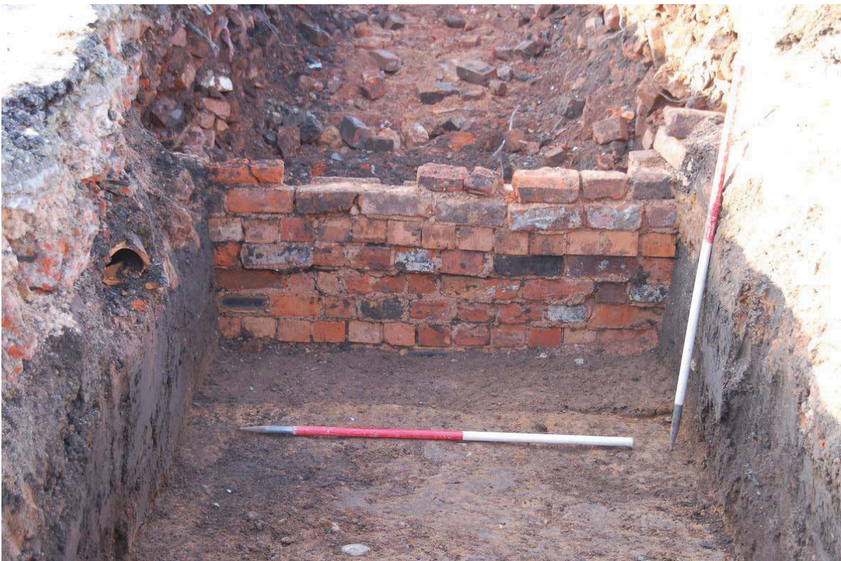
Plate 4: Trench 3, cellar wall 3011, facing west
