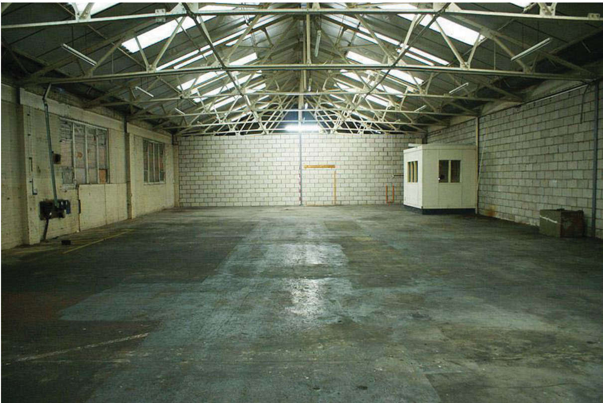
Plate 43: 1950s open space and roof trusses
