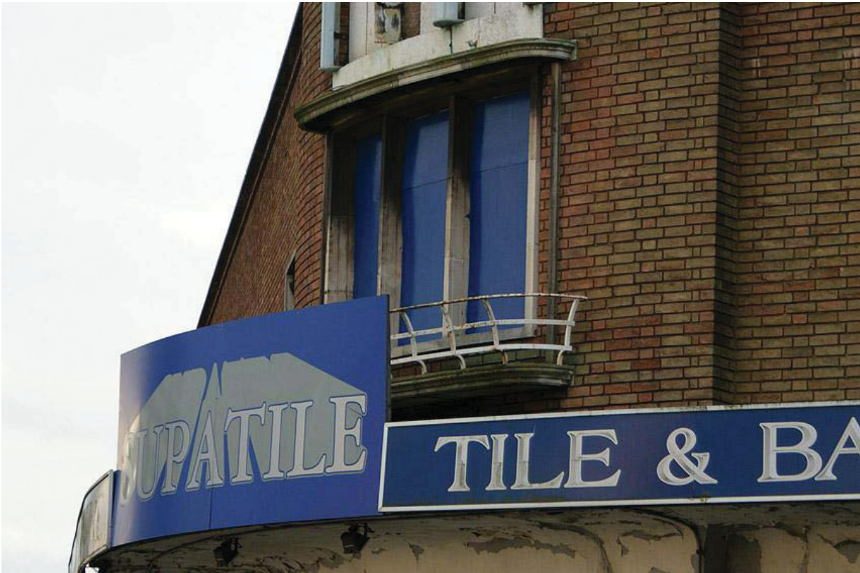
Plate 21: Small balcony in-front of 1 st floor window of the tower
