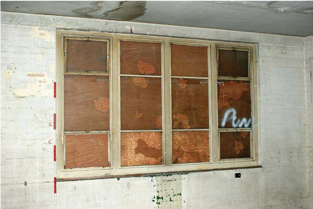
Plate 36: 1940s windows on first floor
