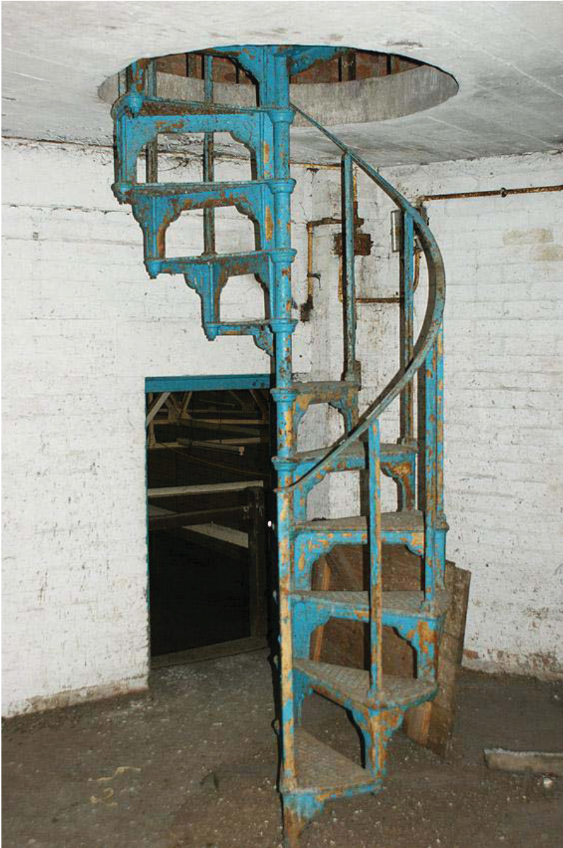
Plate 26: Spiral staircase access within tower
