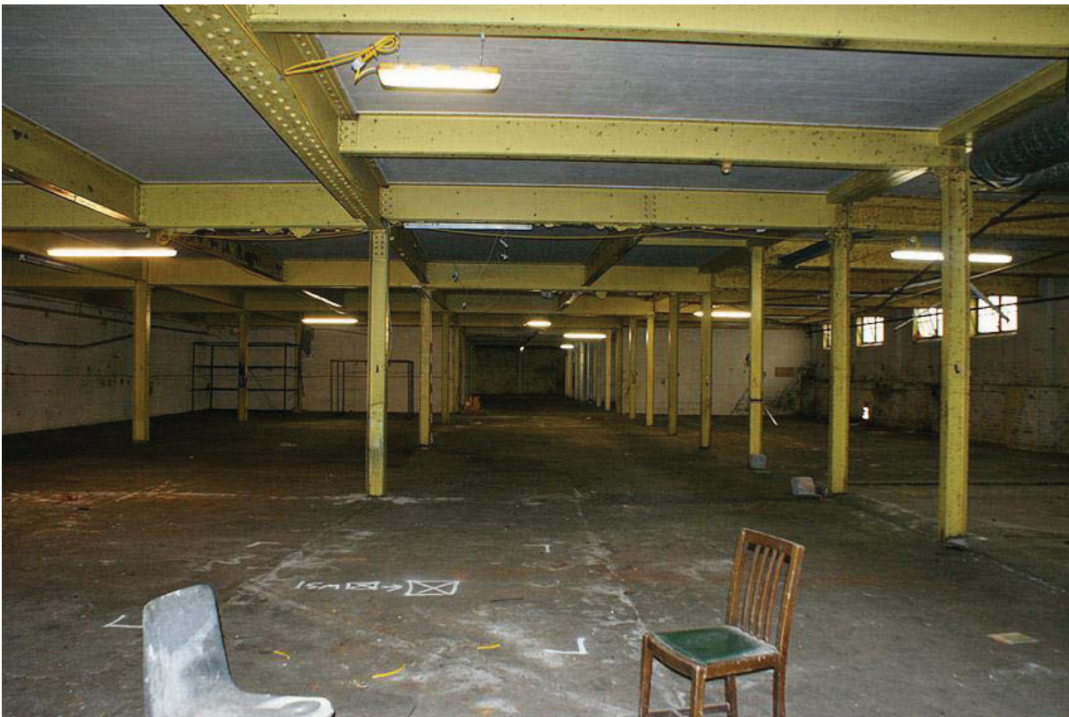
Plate 41: 1950s ground floor interior showing stanchions and RSJs
