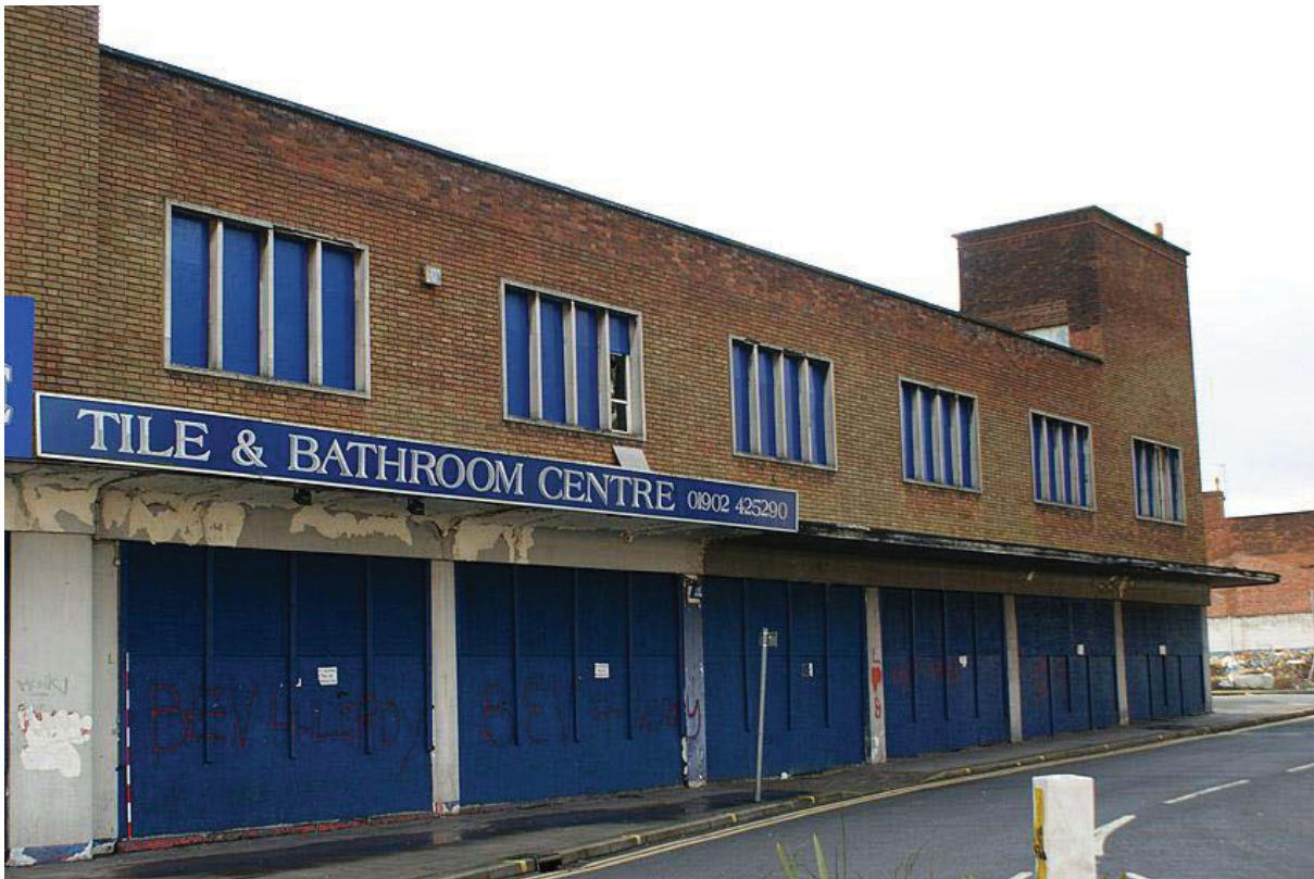
Plate 17: North-west elevation of Attwood building
