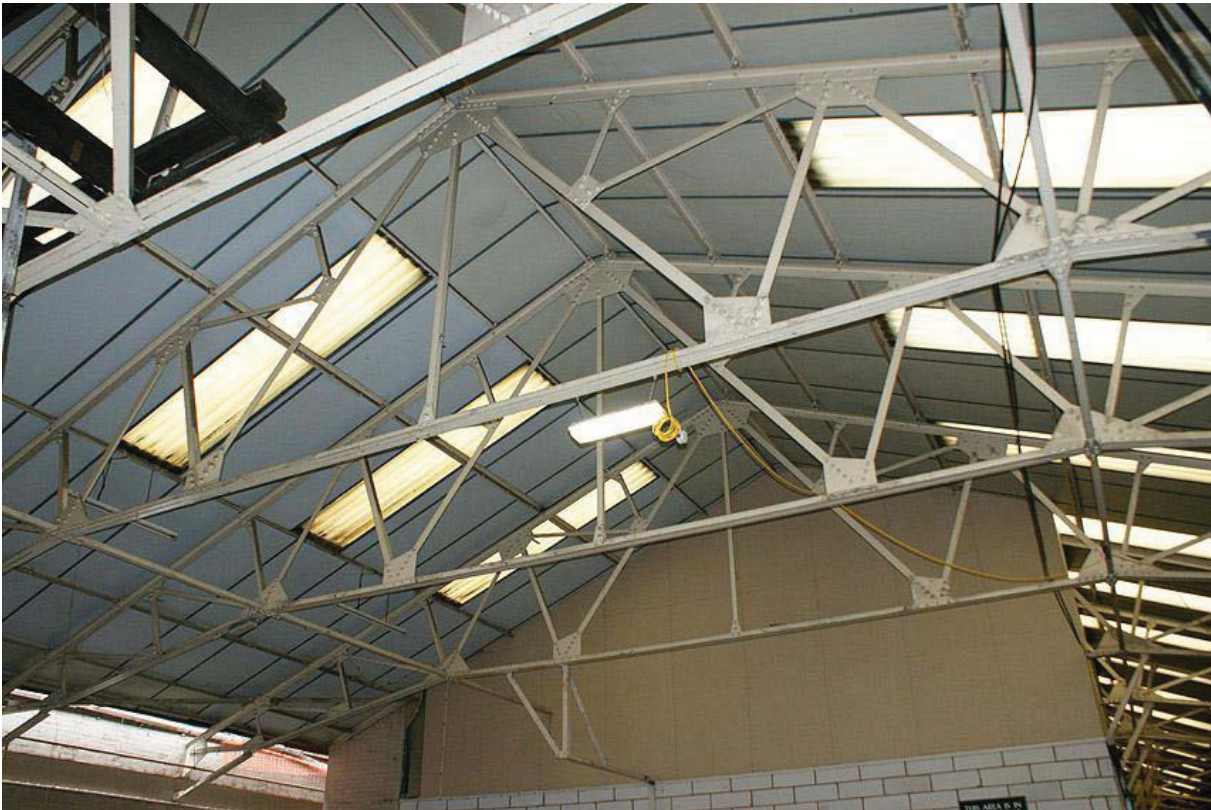
Plate 42: 1950s steel roof structures
