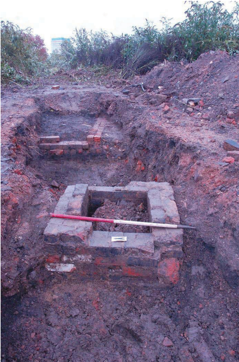
Plate 9: Trench 5, manhole feature 5004 and boundary wall 5003 facing east
