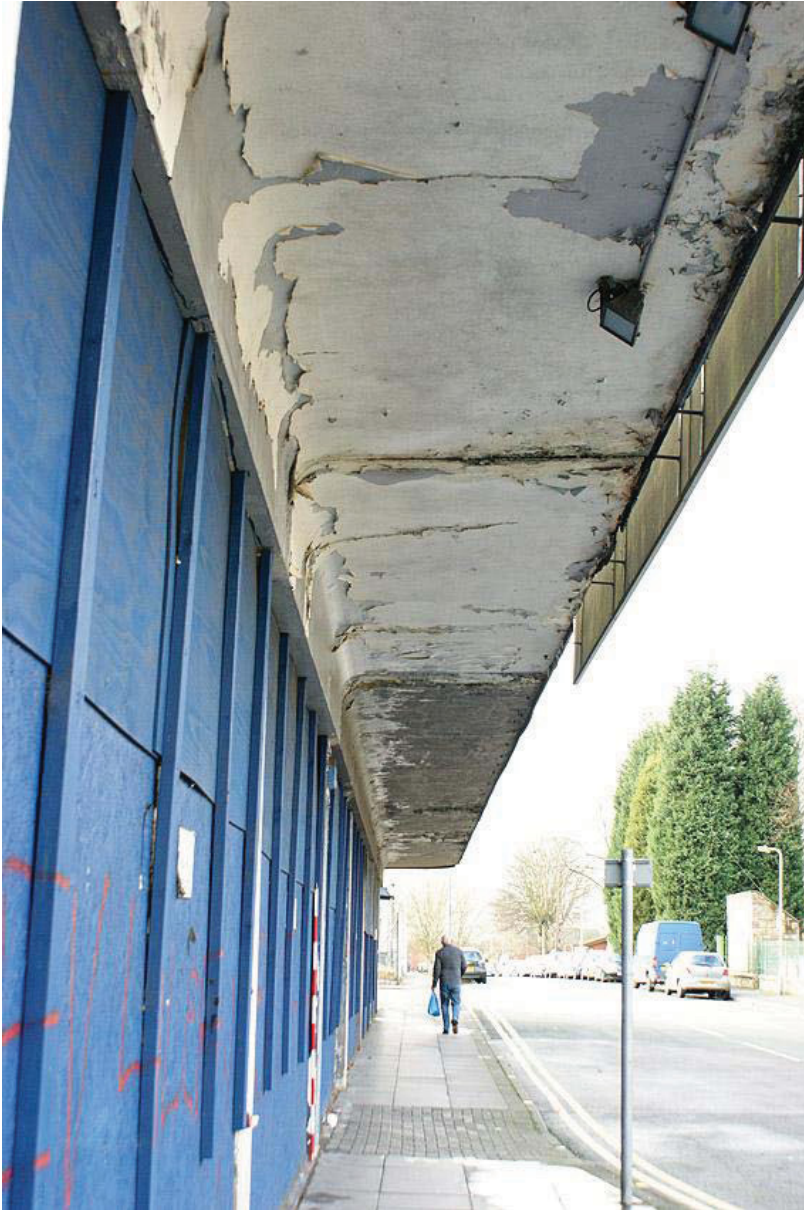
Plate 14: Coving on underside of canopy
