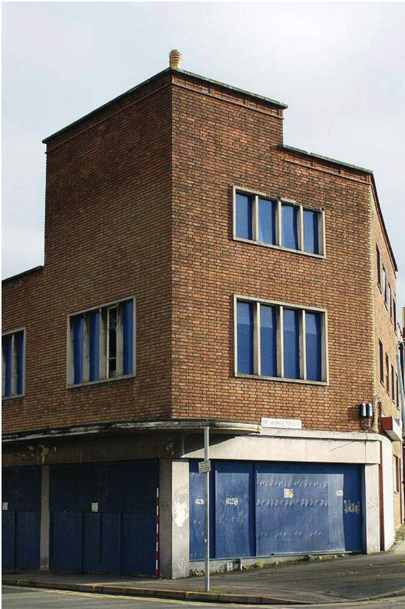
Plate 18: Corner of St Mark's Street and St Mark's Road
