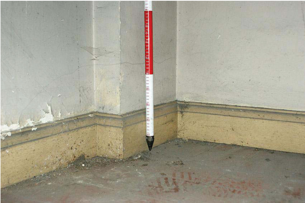
Plate 32: Original skirting within 2 nd floor flat
