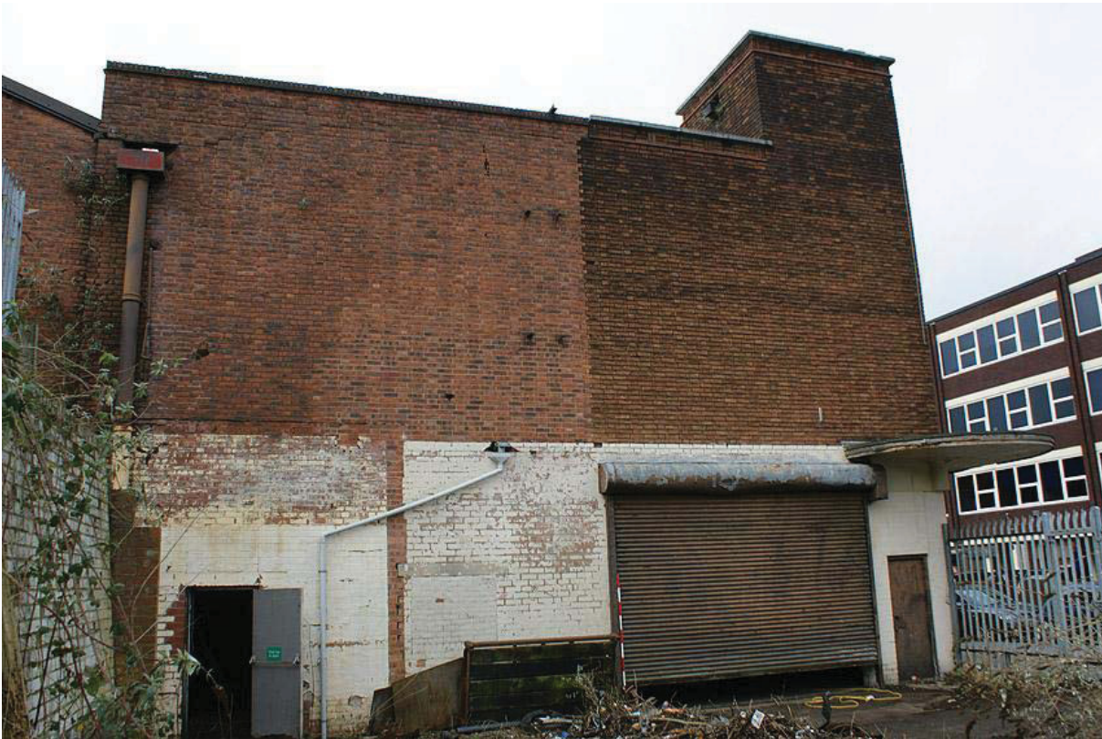
Plate 40: 1950s extension to rear of Raglan Street elevation
