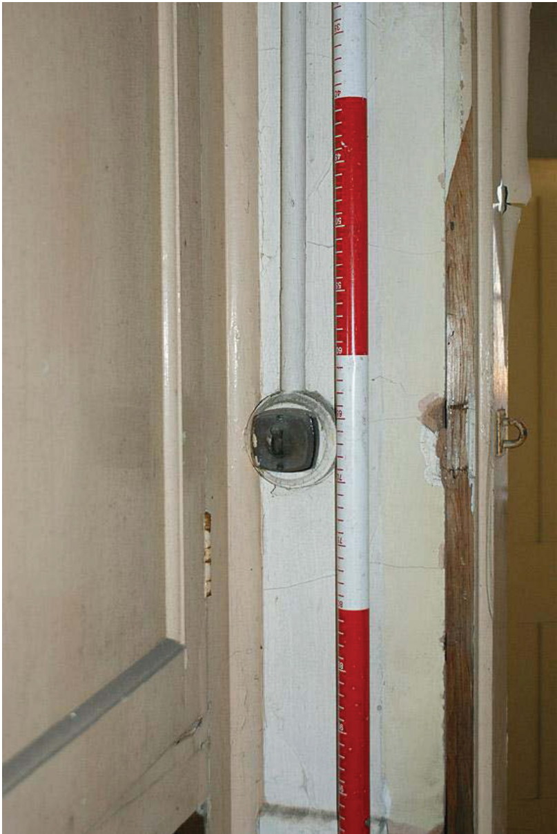
Plate 29: Original electrics within 2 nd floor flat
