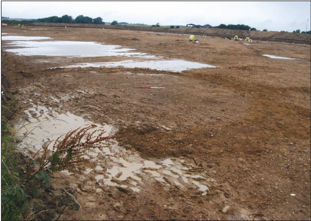
Excavations in progress showing ground conditions
