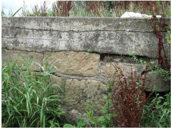
*Plate 2 Retaining wall on south bank. Later phase of concrete over earlier wall probably of stone reused from the abbey*
