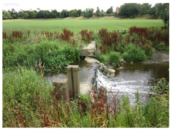
Plate 3 top of picture, retaining wall on south bank. Note stone emerging from concrete, two courses of stone having been removed during works when concrete sluice was inserted
