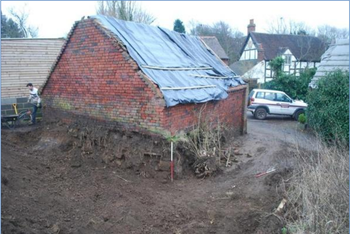
Plate 9 Area around barn reduced to finished levels, looking East
