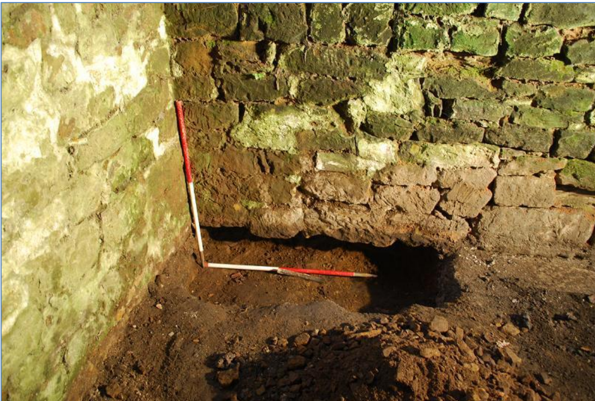
Plate 2 Example of under-pinning trench. View north
