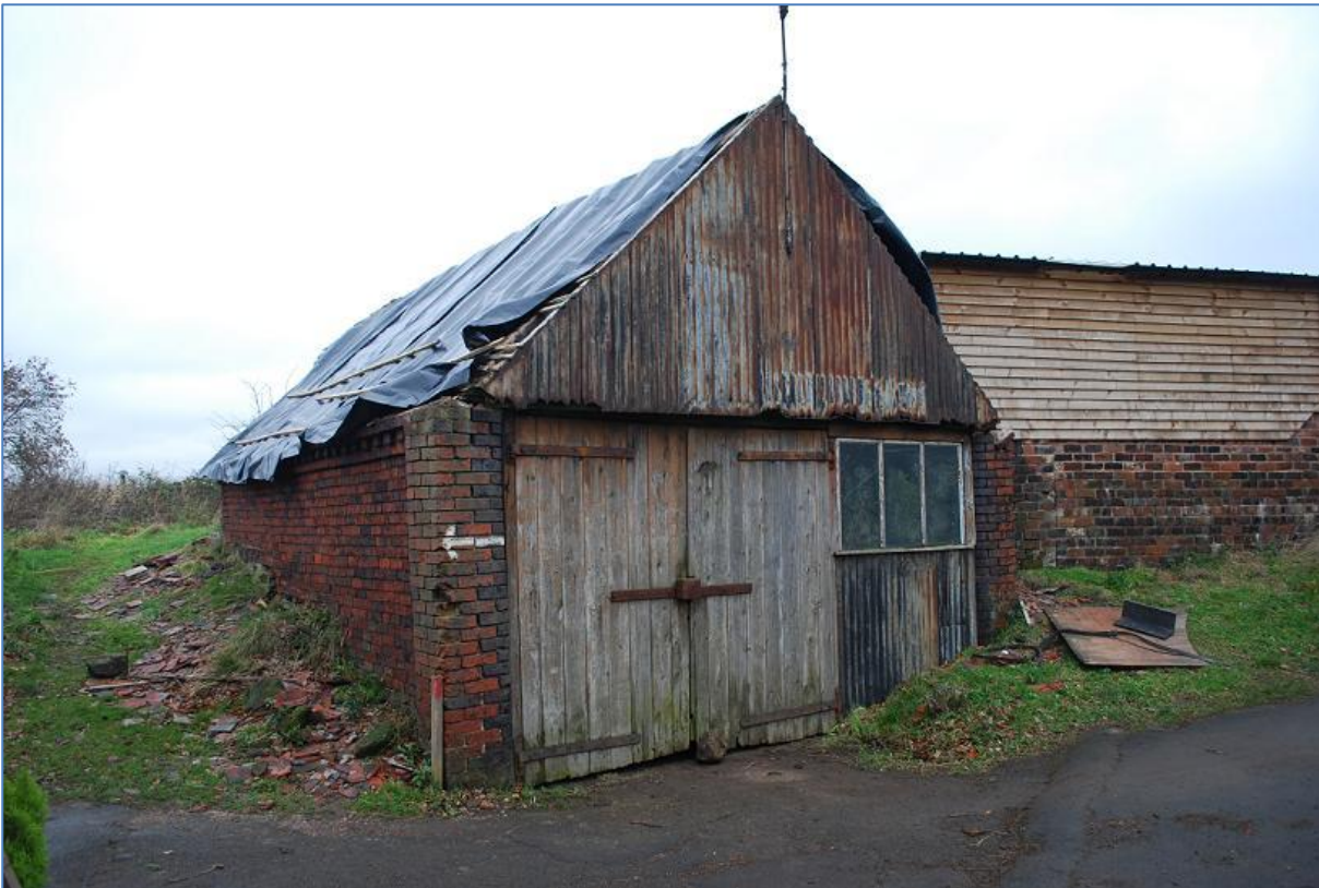
Plate 1 Barn 2 Unit 3, looking north
