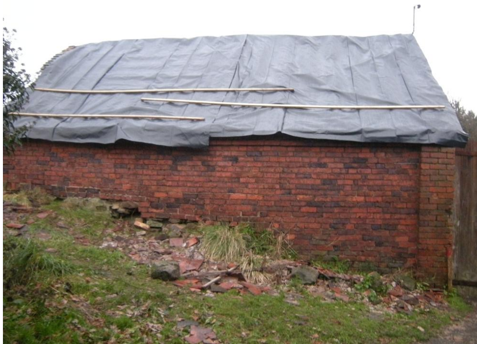
Plate 1 Barn 2 from south-west
