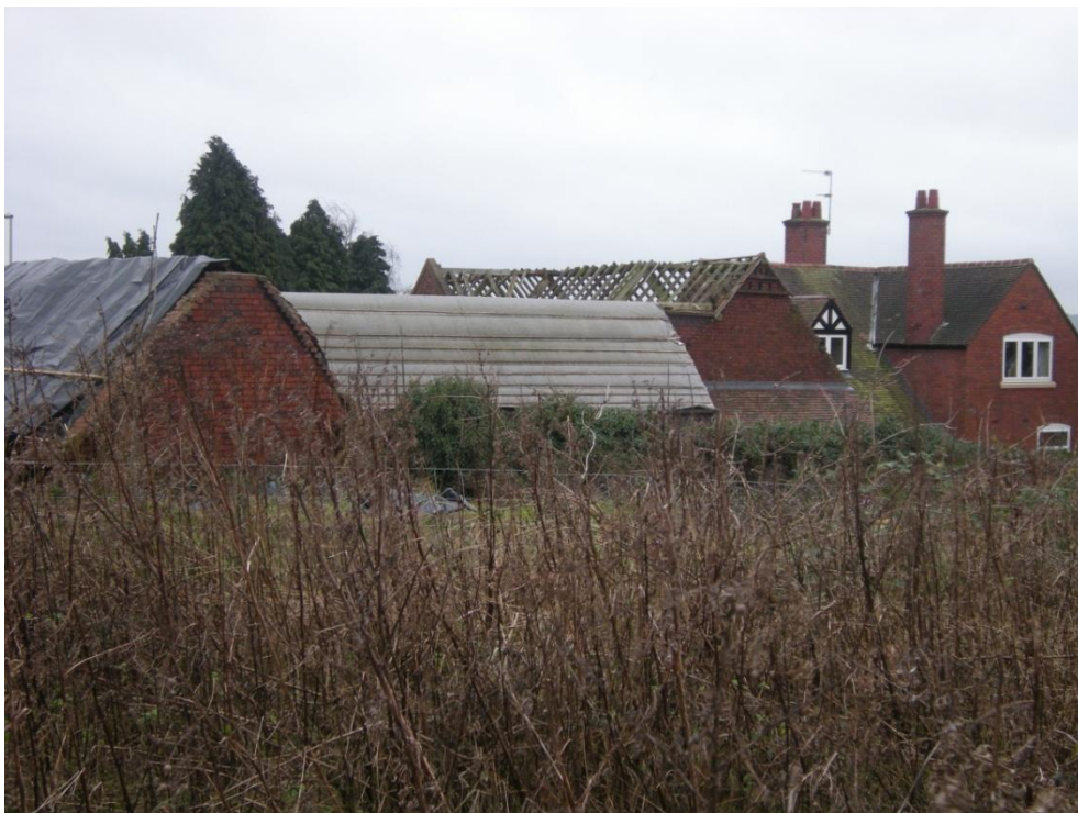
Plate 6 Barn 2 from north-east, showing Pottery Farm Barn (Barn 1)
