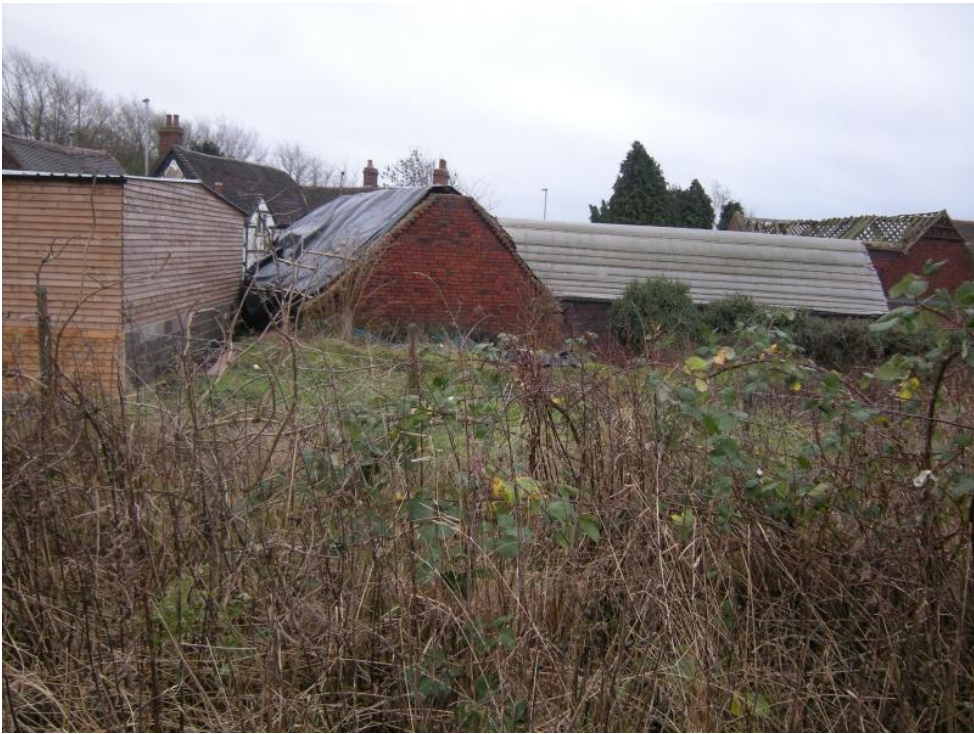
Plate 4 Barn 2 from north-west
