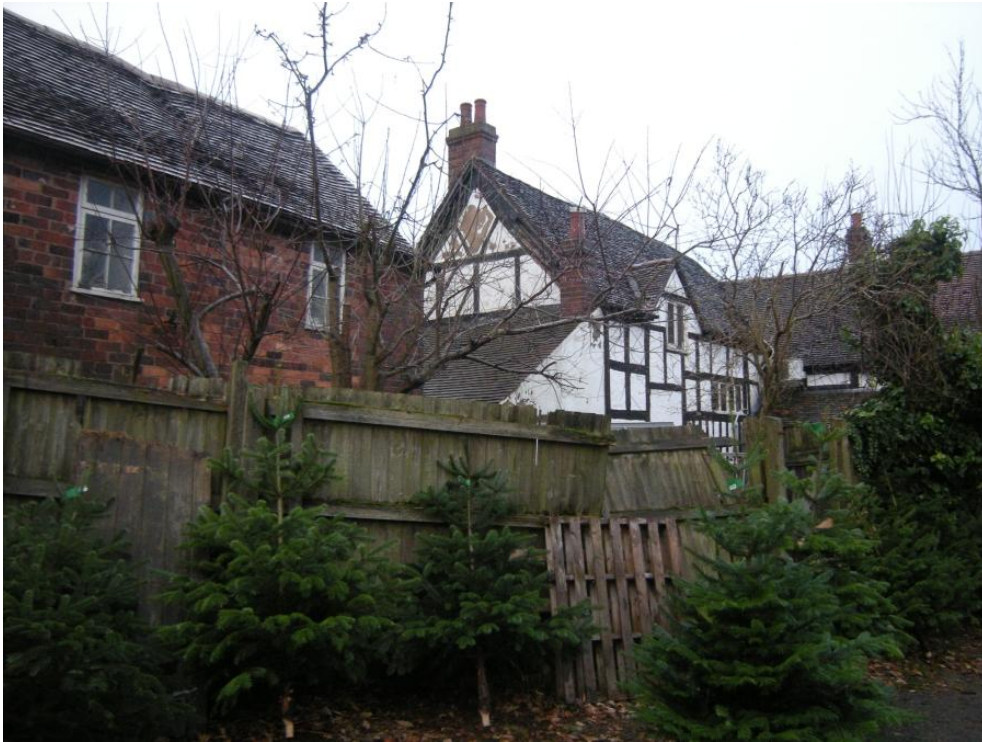
Plate 7 The Old House from north-west, from Barn 2
