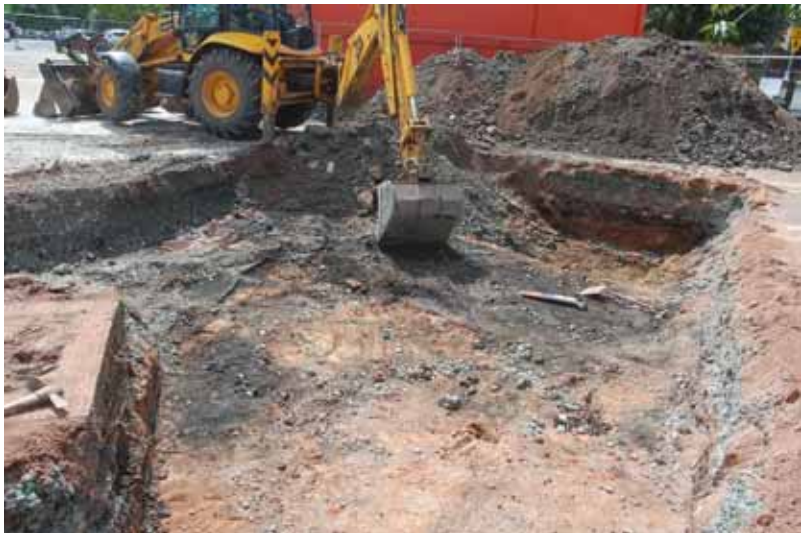
The site being opened with the JCB
