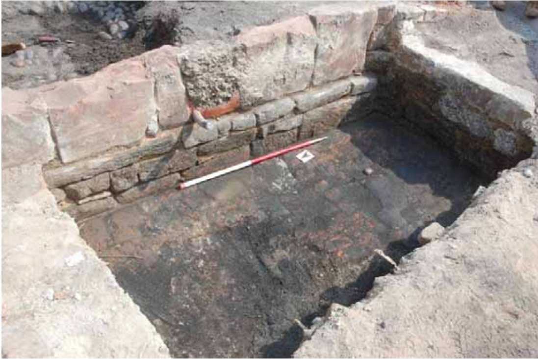
Plate 7: Sandstone foundations and floor of the cellar at the back of house number 6
