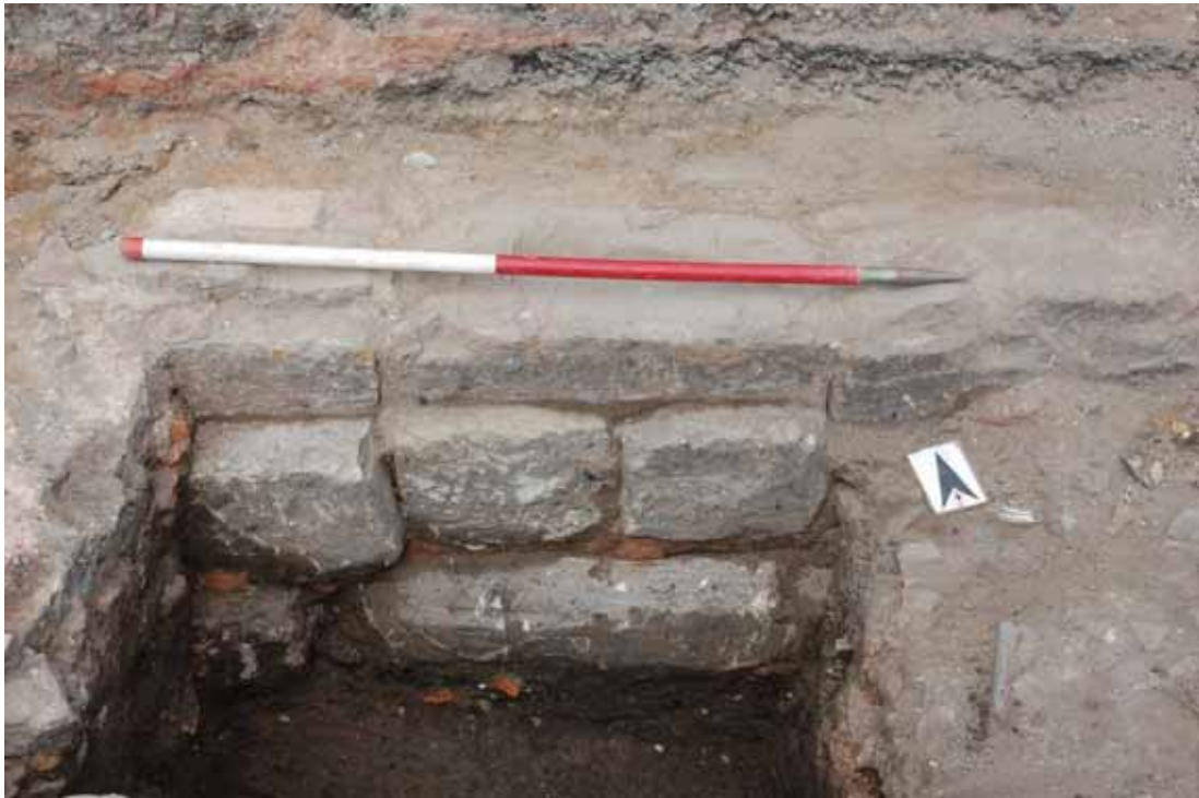
Plate 5: Sandstone foundation wall (26), forming the footings for house number 5; high quality chamfered stone visible in lowest course
