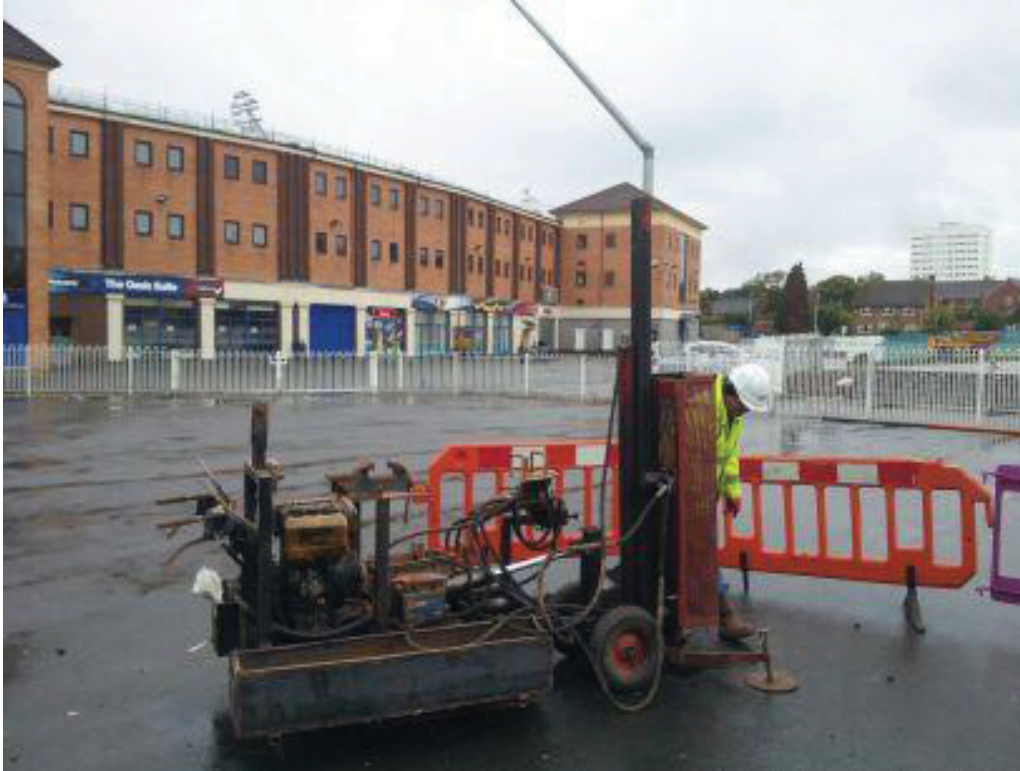
Plate 1 Sinking Borehole 3, looking south-west
