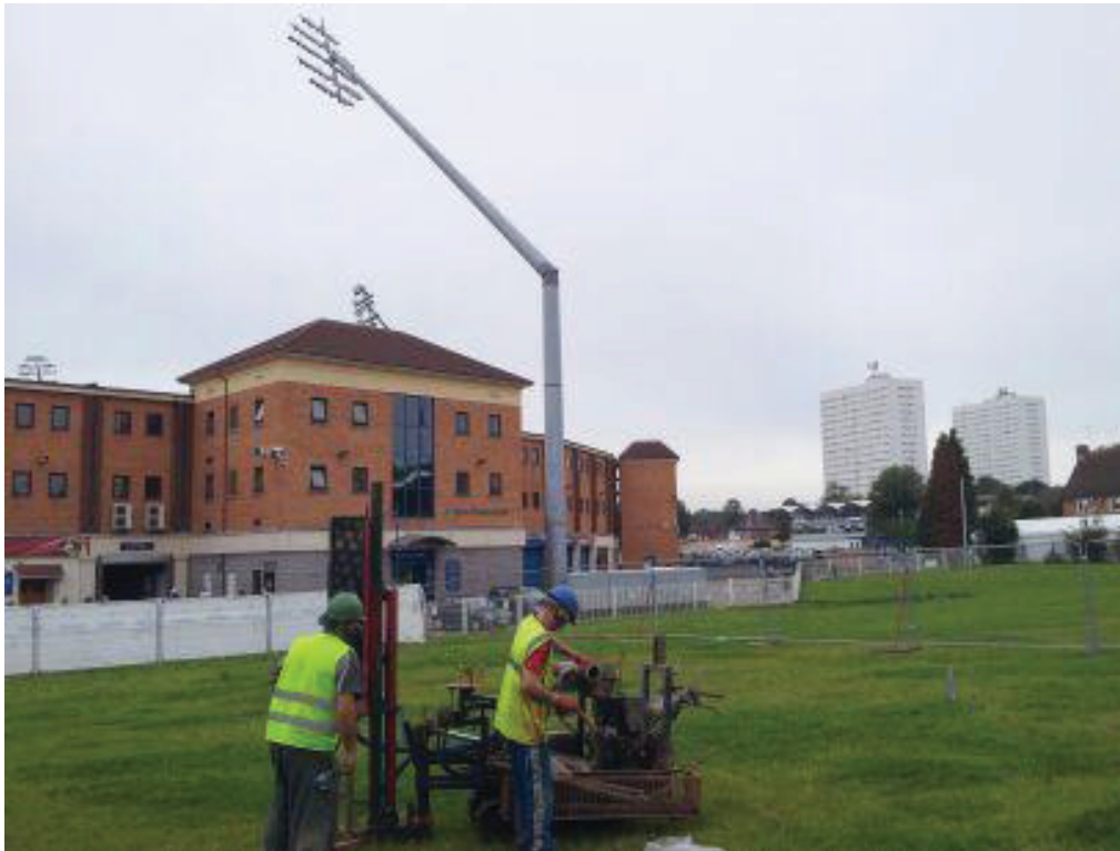
Plate 3 Sinking Borehole 7, looking south-west
