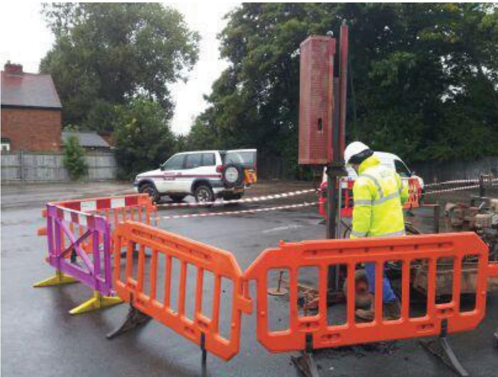
Plate 2 Sinking Borehole 3, looking north-east
