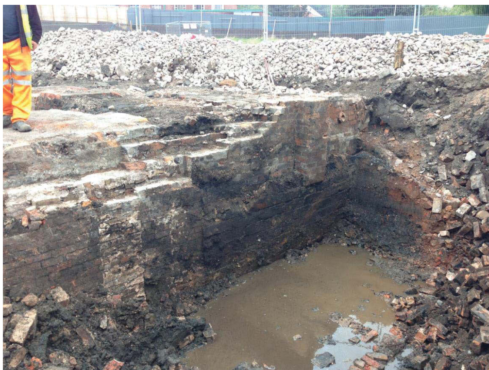
Plate 13: The northern part of structure (1101/1102) was constructed of iron slag and ceramic bricks, and was constructed over a number of phases; view north-west
