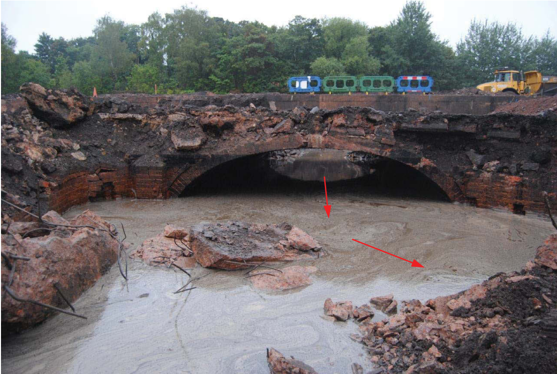
Plate 7: Brick culvert (1030), with retaining wall (202/1003) visible to the right. In the foreground the broken out remains of a later concrete slab extension to the culvert (1034) are visible; view south-west
