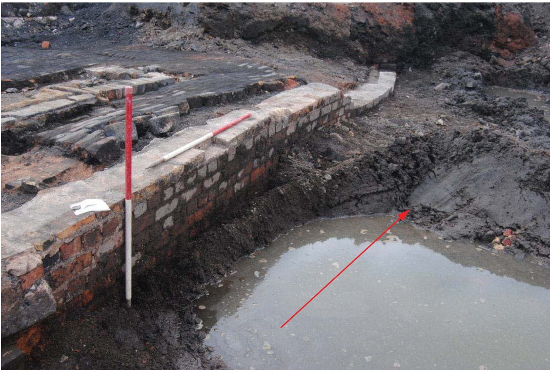
Plate 6: Wall (1003) formed a retaining wall for the channel running to the east of the mill. The arrows indicate the direction of flow; view west
