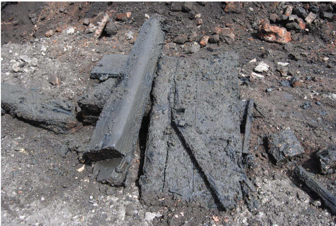
Plate 12: The remains of sluice gate (1027) were also observed during the watching brief as (404)
