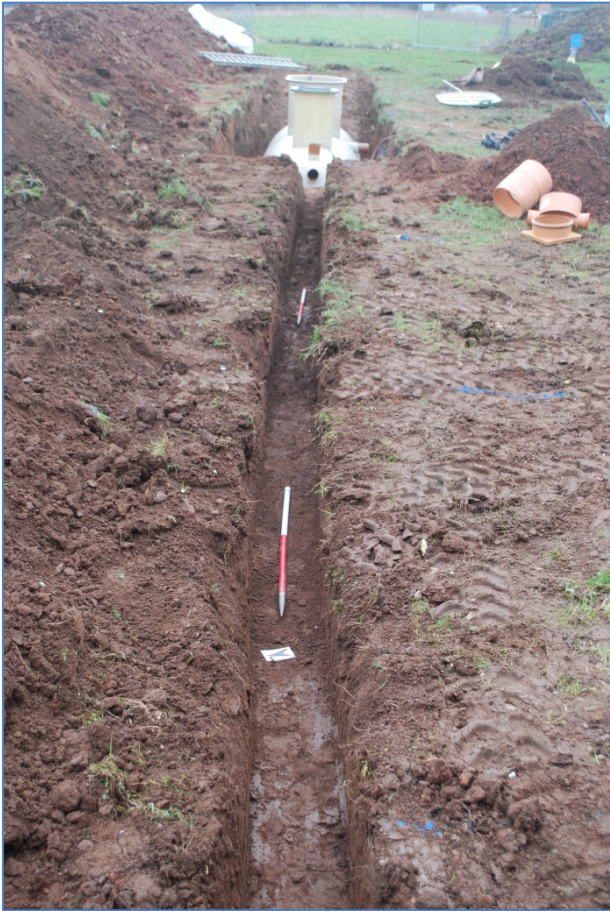
Plate 7: Trench 3, view south-east, 1m scales
