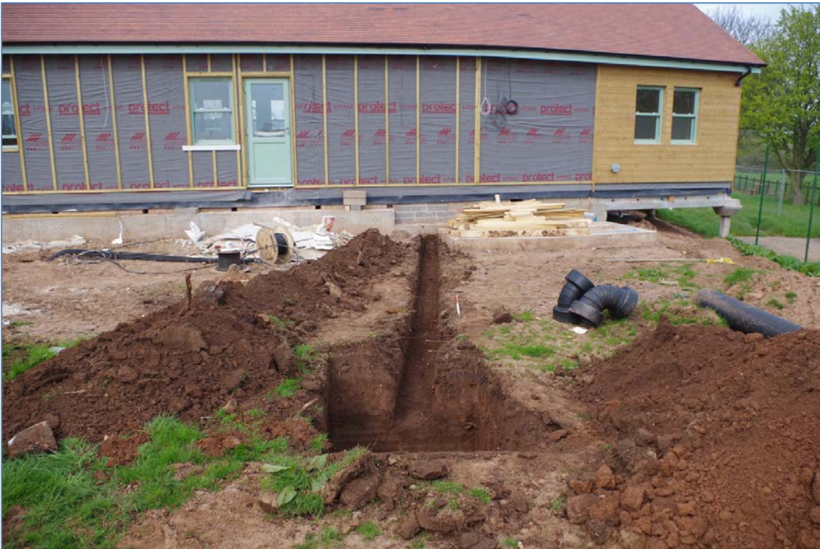
Plate 11: Trench 7 soakaway trench, view north-west, 1m scale
