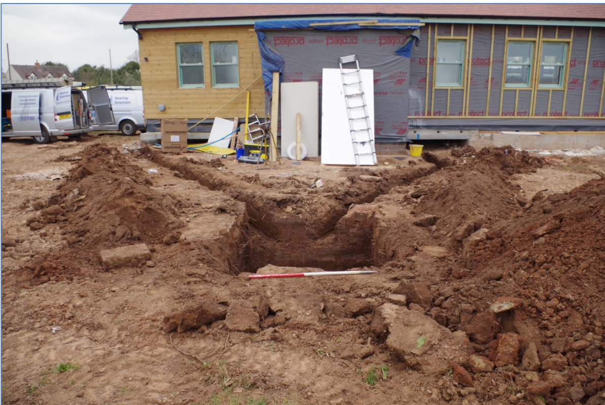
Plate 12: Trench 8 soakaway trench, view west, 1m scale
