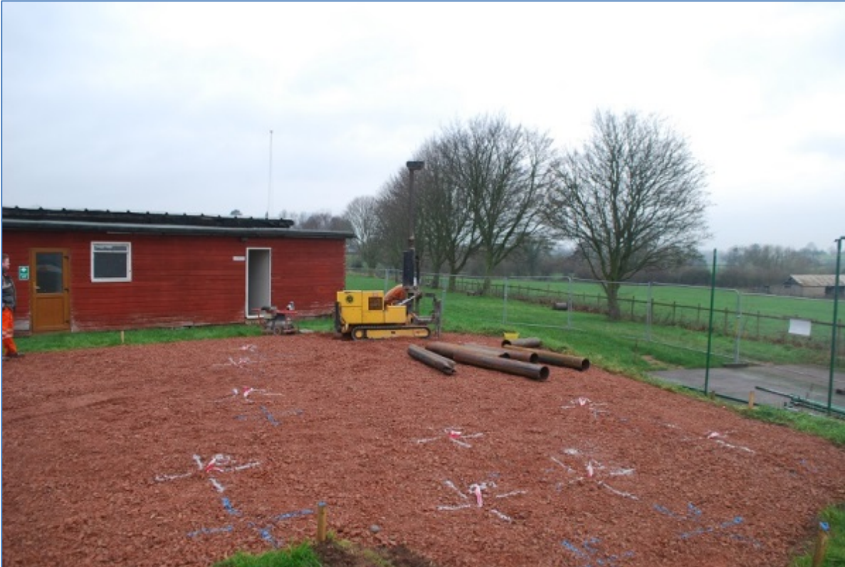
Plate 3: Area after piling matt levelling; piling in progress, looking north-west
