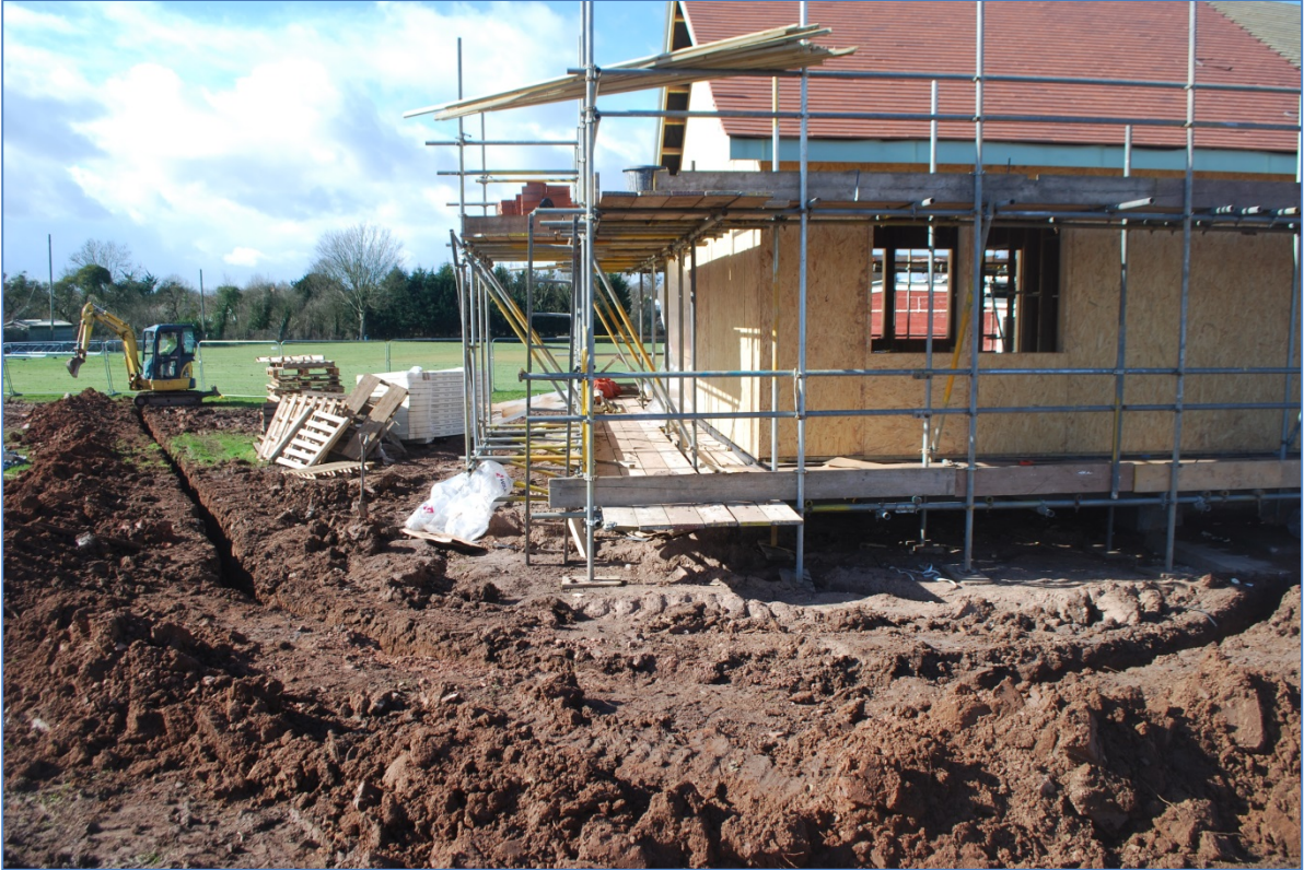
Plate 10: Trench 6, service trench, view west
