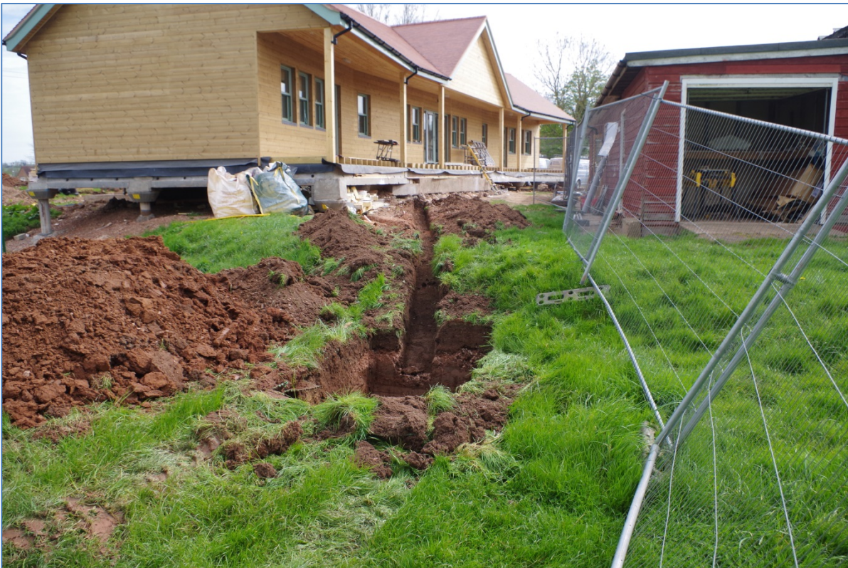
Plate 14: Trench 10 soakaway trench, view south-east
