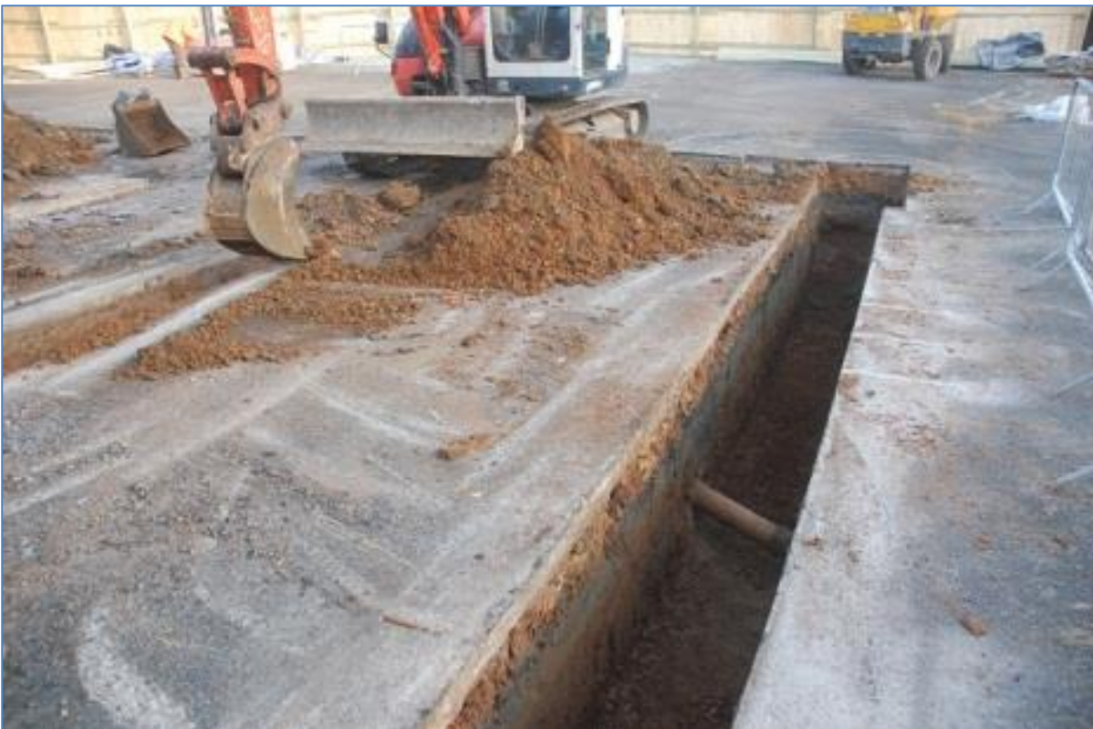
Plate 2 Ground beam in Trench 1 cut by modern drainage
