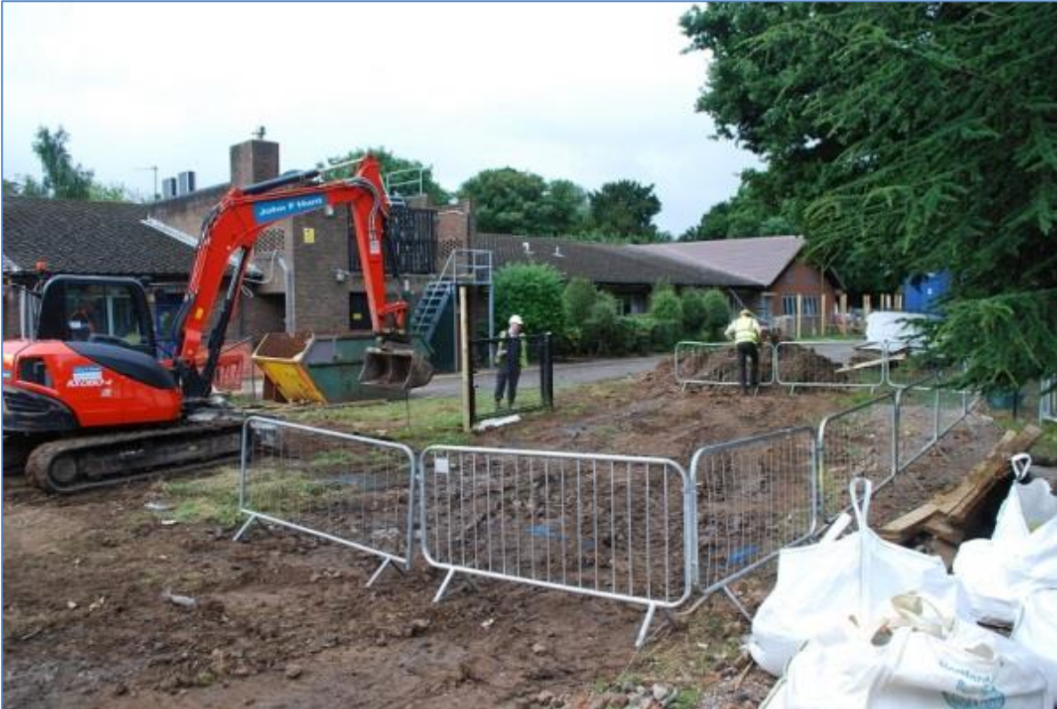
Plate 9 Trench 5 marked out in front of school entrance before works
