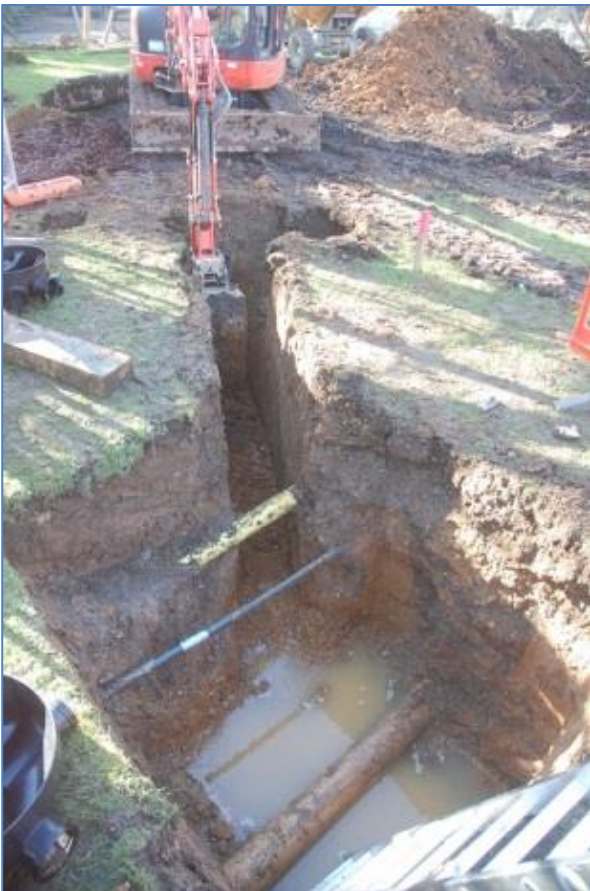
Plate 4 Trench 2 drainage for the south-western extension
