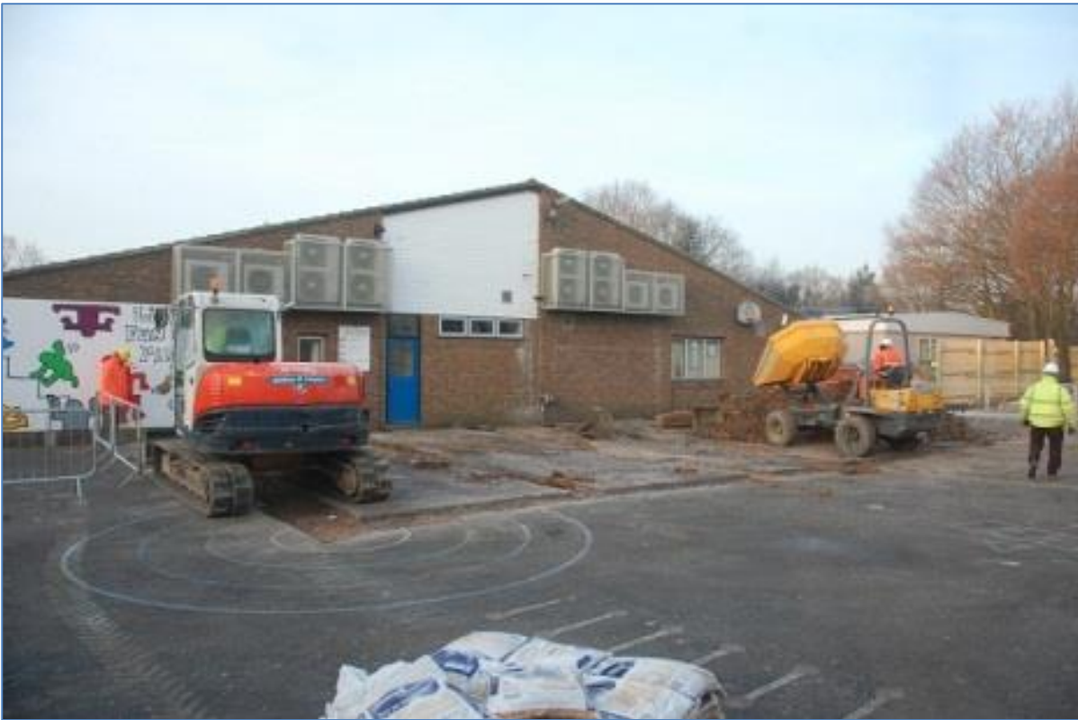
Plate 1 Ground beam excavations to the north-eastern extension in progress
