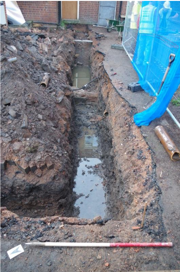
Plate 1 Excavated trench viewed from the north west
