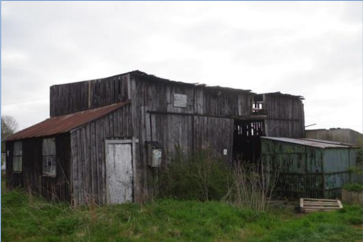
Plate 1 The Black Shed on site
