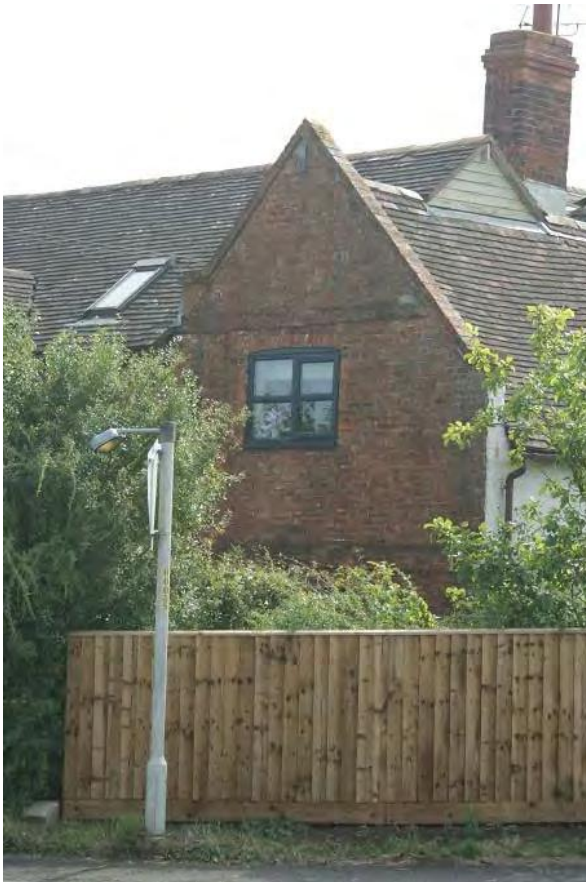
Plate 32 Gable end of former farmhouse, looking south-east
