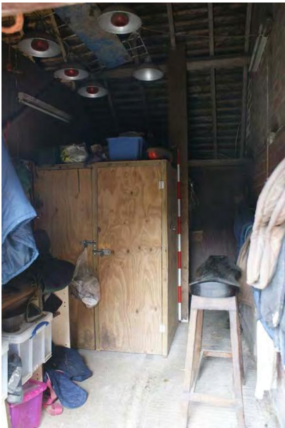
Plate 12 Northern range interior, looking north
