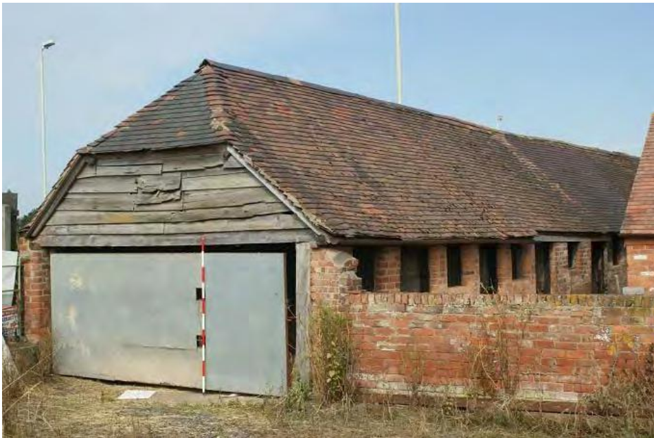
Plate 24 Western range, looking north-west
