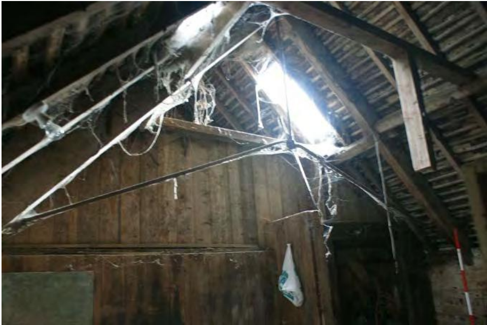
Plate 30 Interior of northern range, looking south-east
