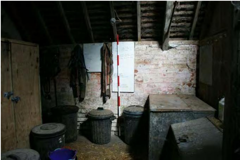
Plate 13 Northern range interior, looking north
