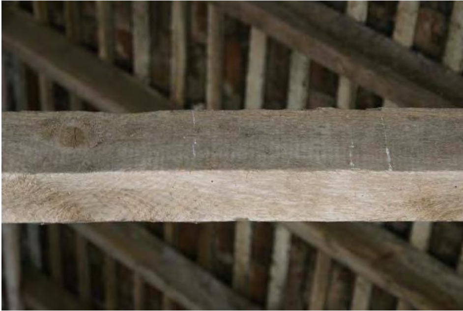
Plate 11 showing evidence of the conversion techniques used on the timbers
