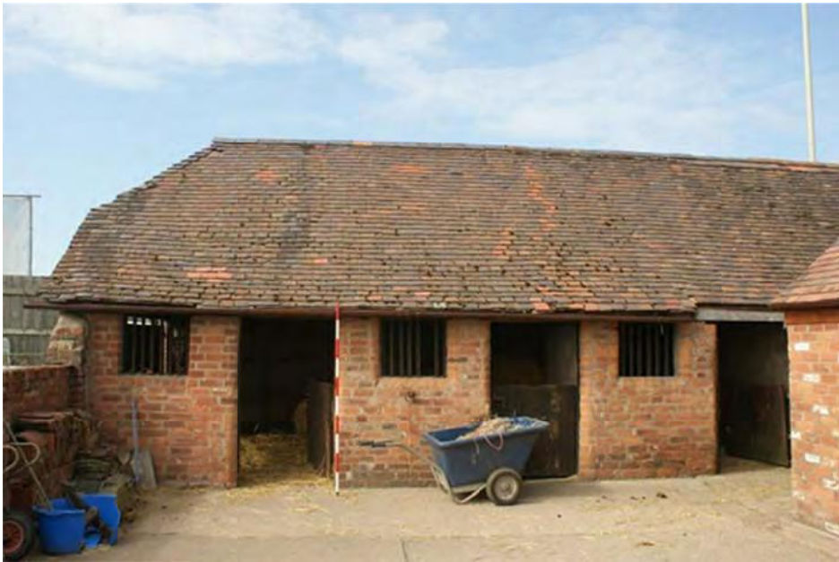
Plate 22 Western range, looking west
