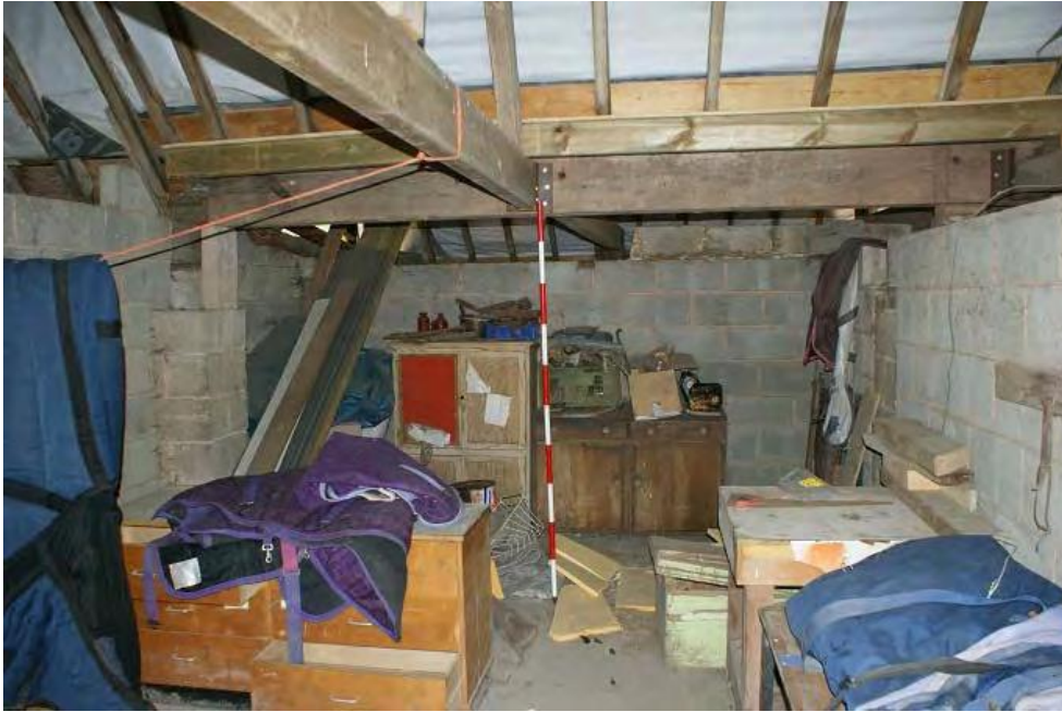
Plate 31 Interior of southern range, looking west
