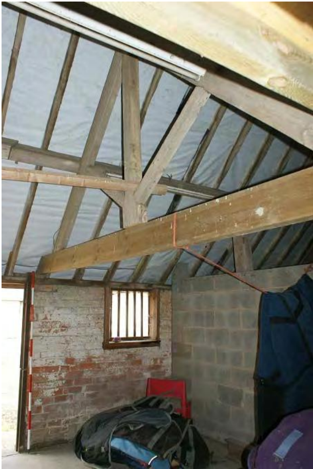
Plate 20 Central range interior, looking north-east
