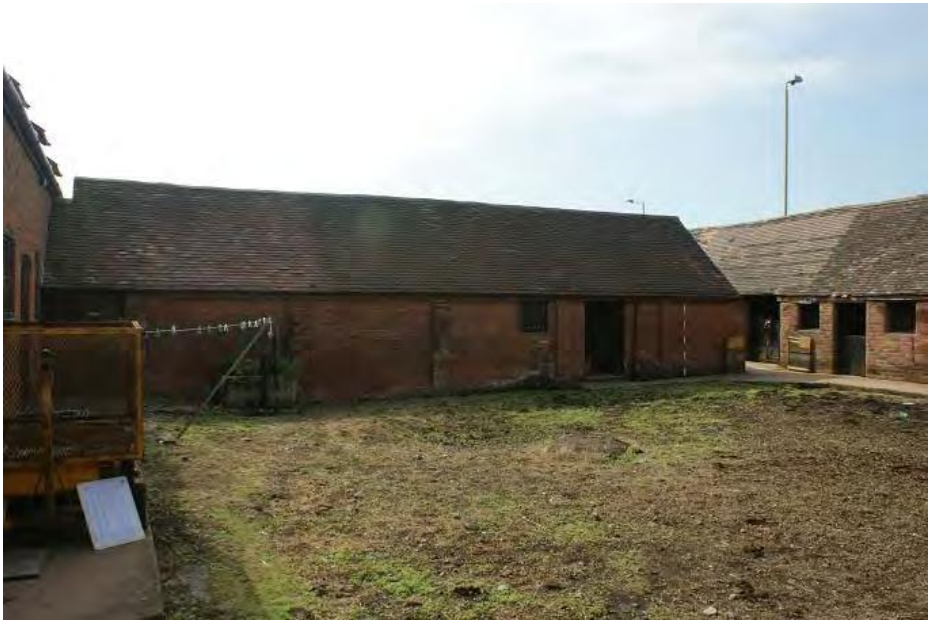
Plate 19 Central range, looking south
