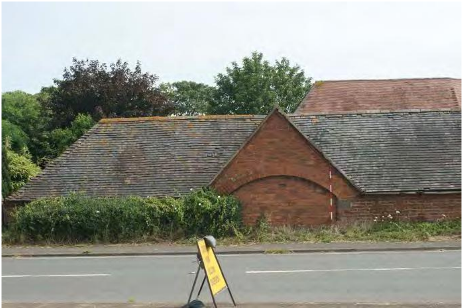
Plate 1. Blocked cart entrance, looking east
