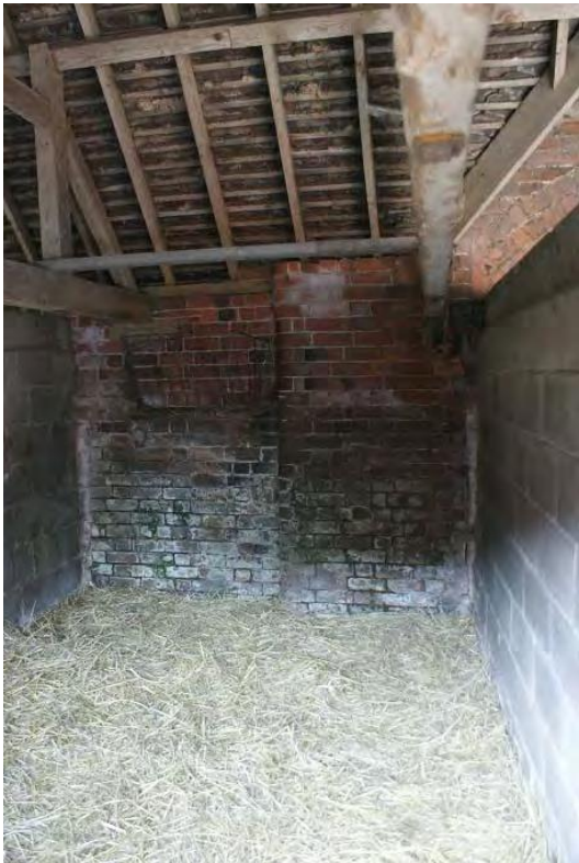
Plate 17 Western range interior, looking west
