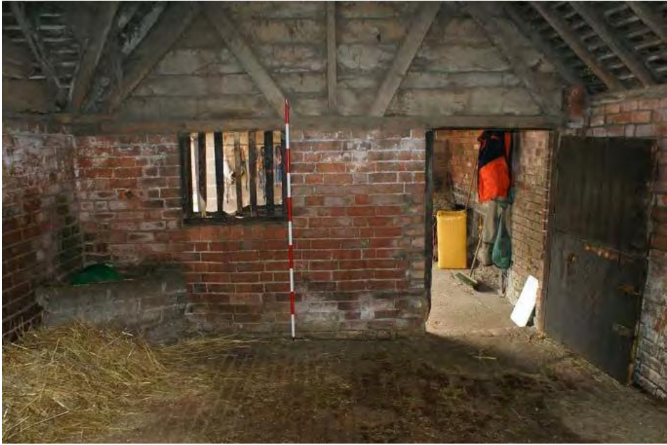
Plate 14 Northern range interior, looking north
