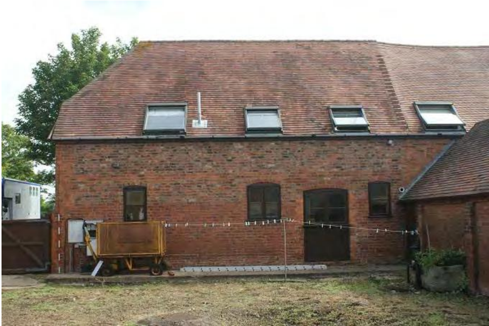
Plate 25 Former stable and hayloft, looking east
