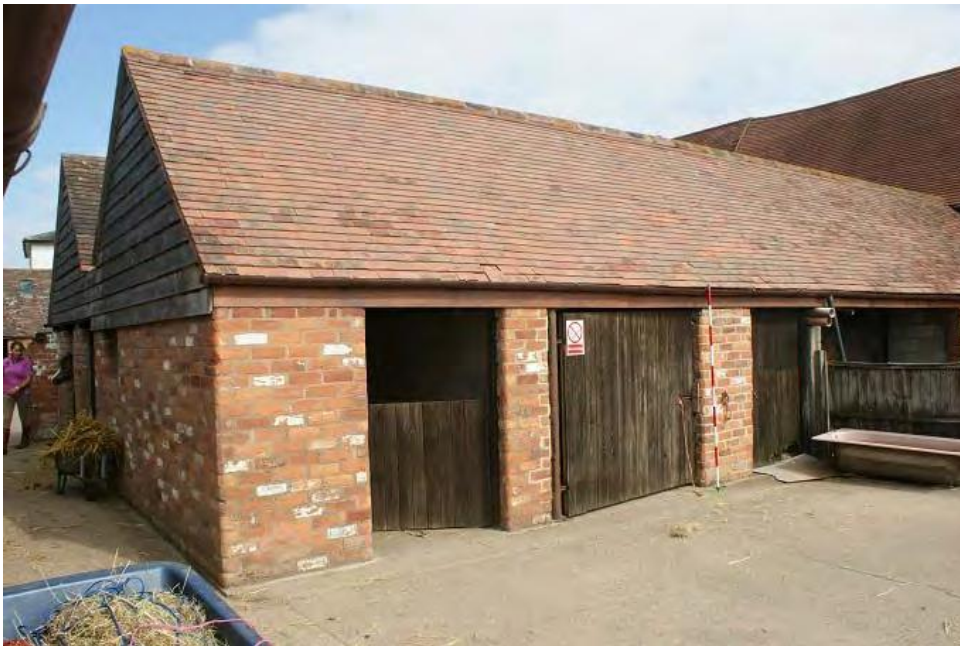
Plate 28 Southern range, looking north-east
