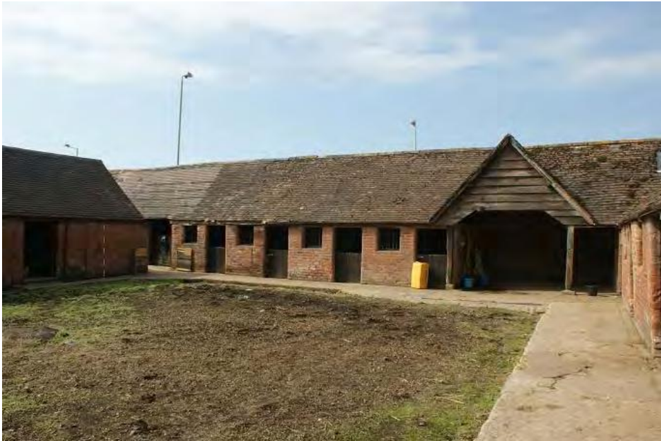
Plate 16 Western range, looking west
