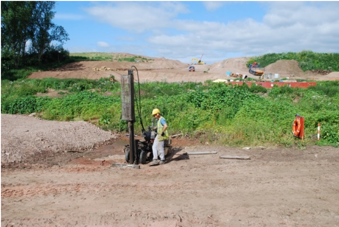
Plate 3 Borehole 4 drilling in progress. Looking west.
