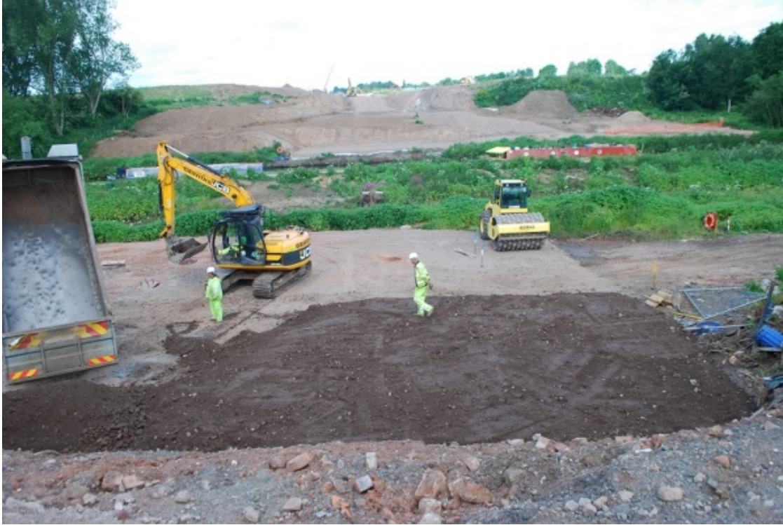
Plate 4 The bridge works in progress, looking west towards the Link Road.
