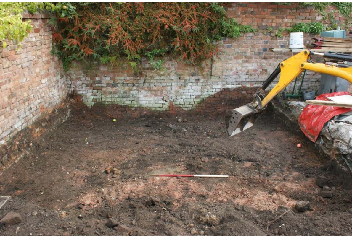
Plate 2 Trench 1 excavation in progress, view east, 2m scale
