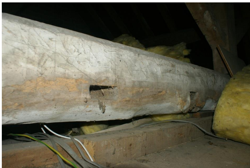
Plate 27 Phase 1 warehouse, evidence of floor joists in roof truss tie beam, looking south west
