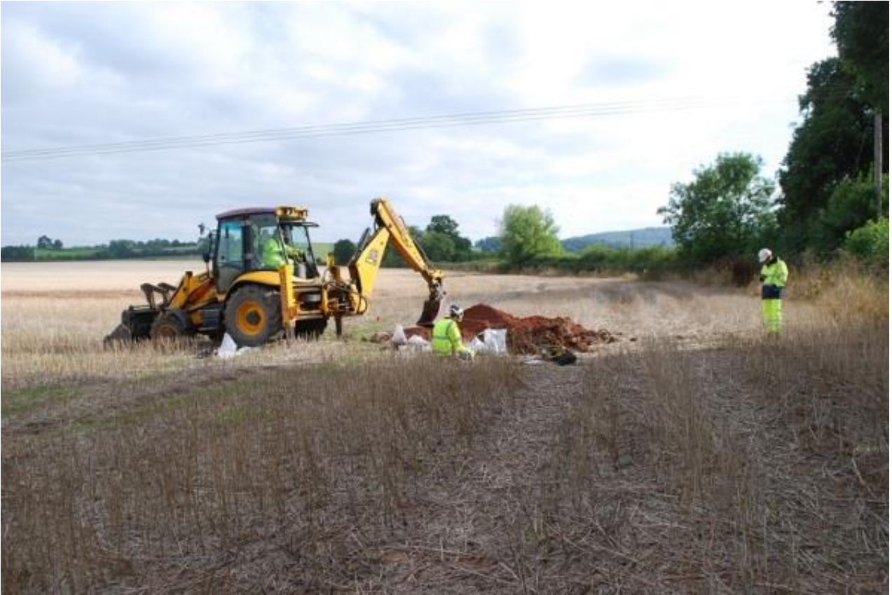
Plate 14 Undertaking geotechnical pitting
