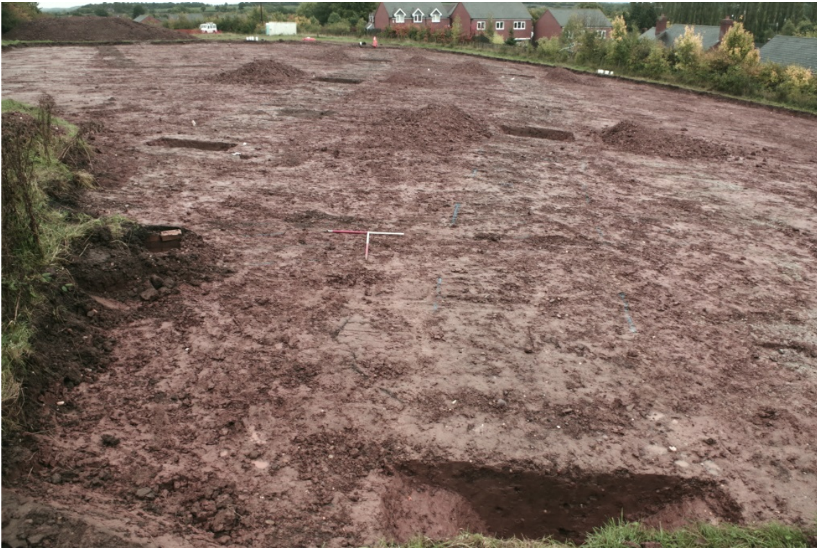
Figure 12 Site looking NE, 1m scales
