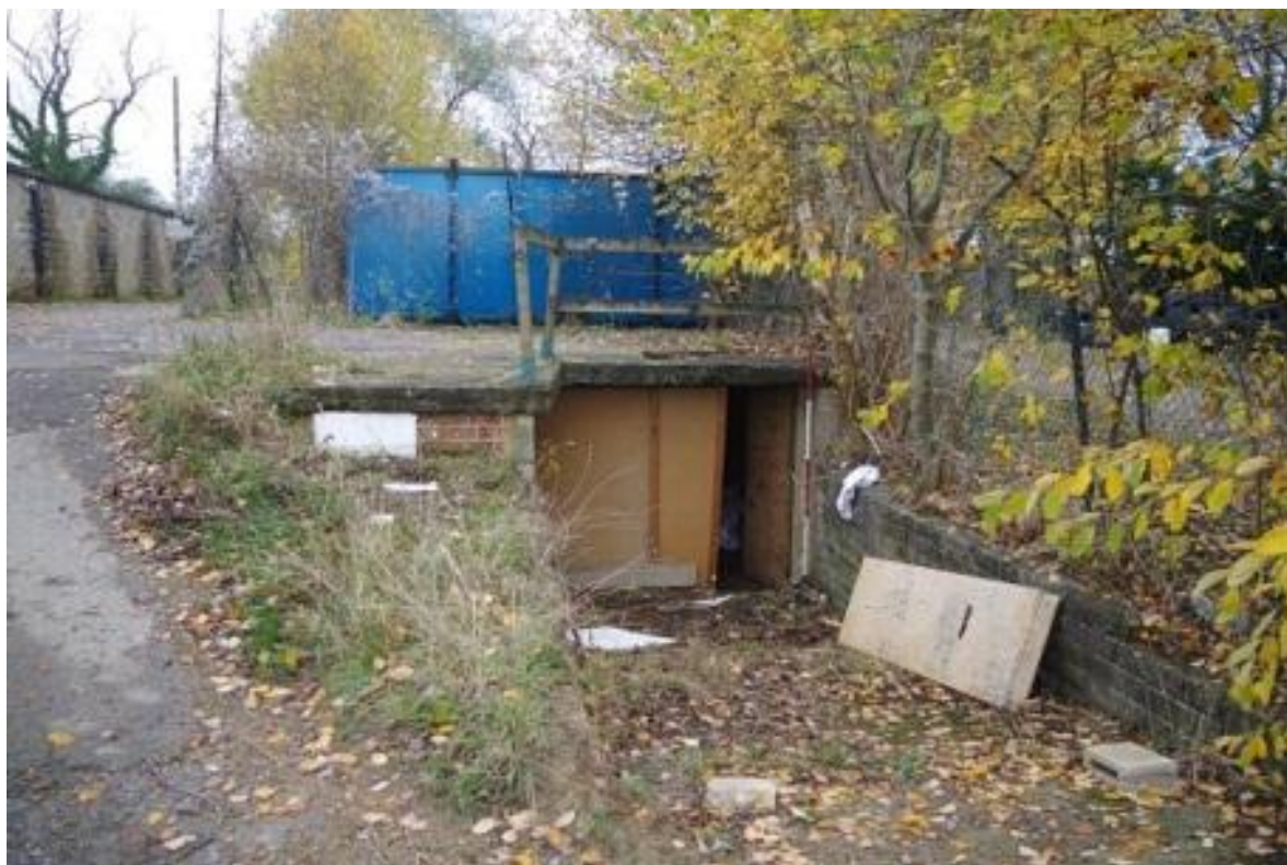
Plate 2, Exterior view of the existing east entrance, looking west (2m scale)
