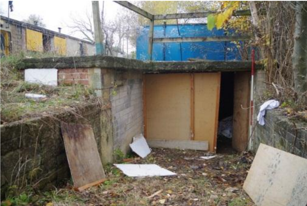
Plate 3, Exterior view of the existing east entrance, looking west (2m scale)
