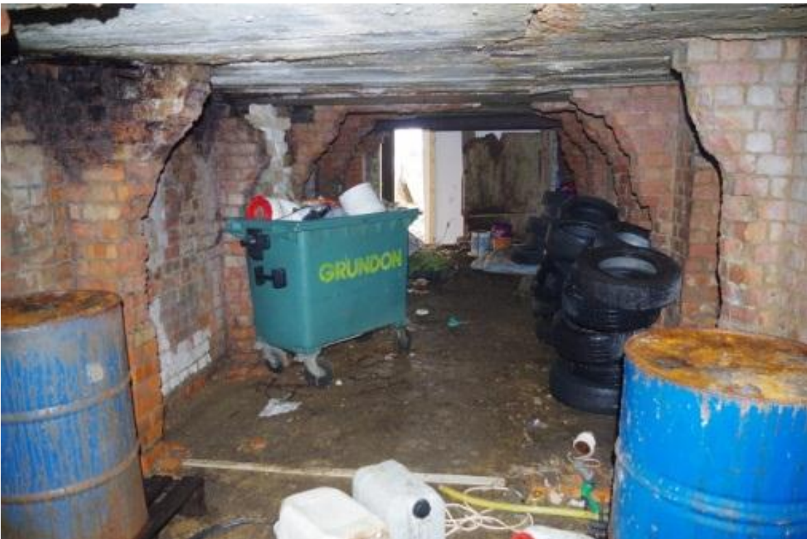
Plate 8, Interior showing the truncated wall divides, looking east toward existing entrance
