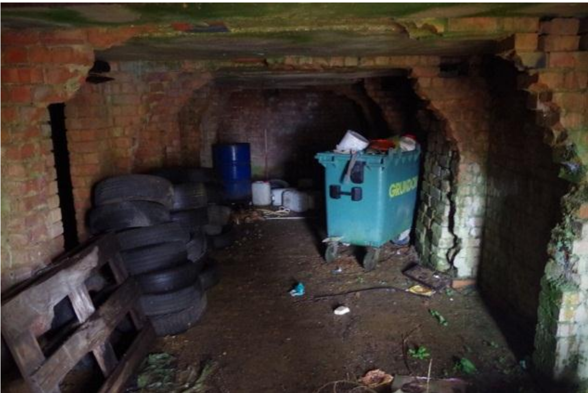
Plate 6, Interior showing the truncated wall divides, looking west
