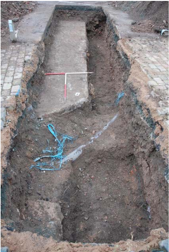
Plate 8: Concrete slab and water pipe in Trench 3
