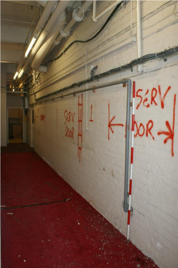
Plate 10 Former eastern wall of structure, Phase 2 (G34)
