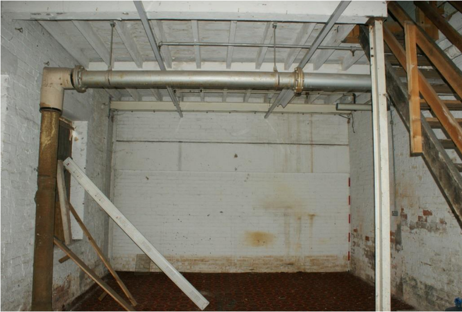
Plate 18 Ground floor within four bay, two storey structure, Phase 2 (G46)
