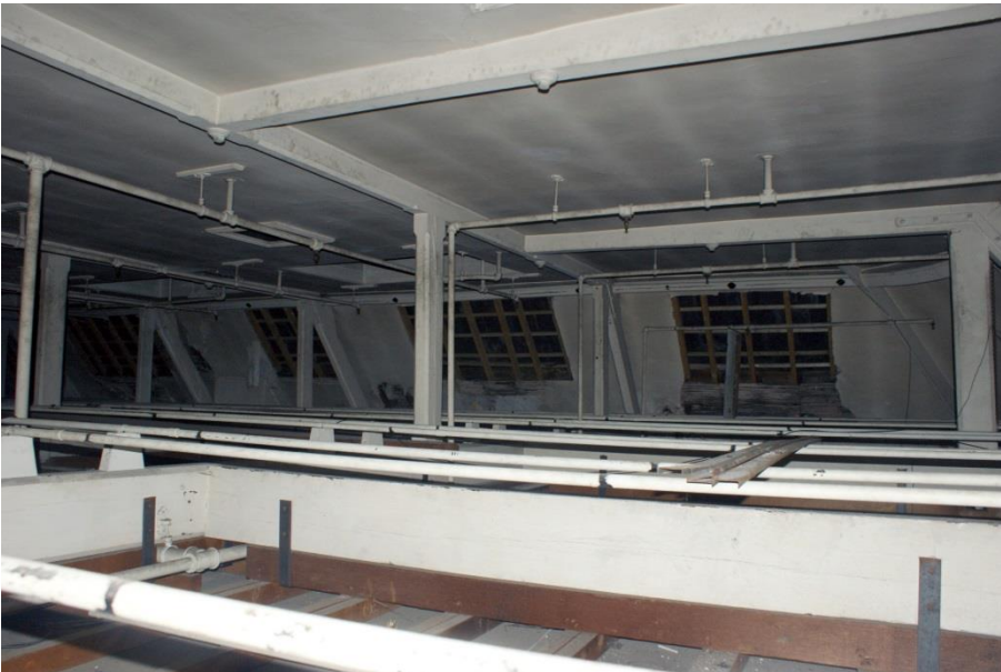
Plate 44 Phase 3 (S28), above modern suspended roof
