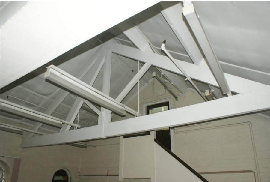
Plate 6 Kingpost truss, Phase 1 (GF1)
