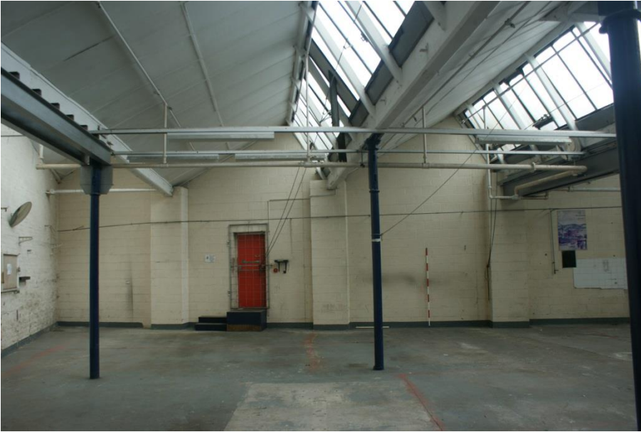
Plate 14 Former weaving shed, Phase 2 (G48)
