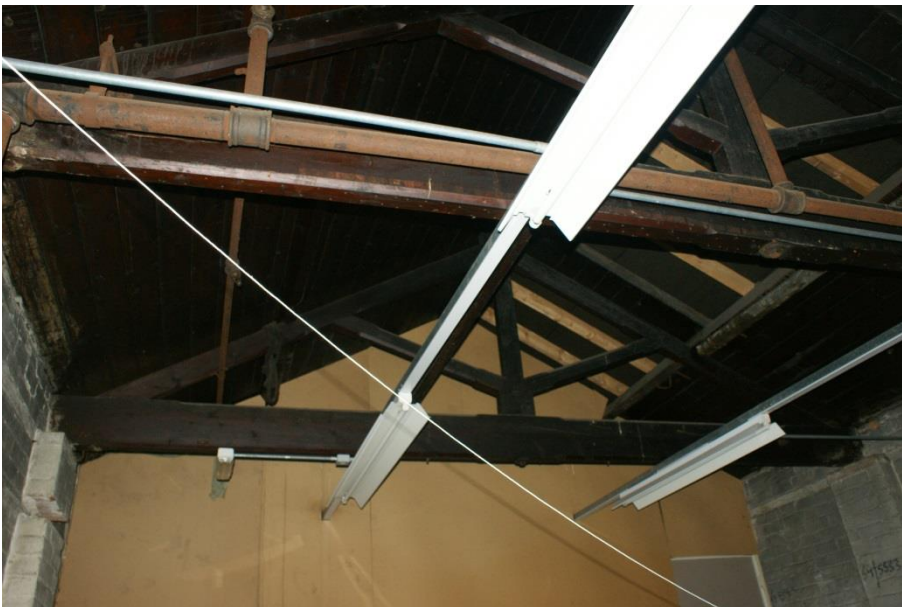
Plate 17 Kingpost trusses within four bay, two storey structure, Phase 2 (F38)
