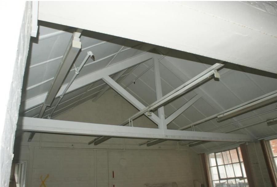
Plate 8 Kingpost truss within two bay structure, Phase 2 (GF1)
