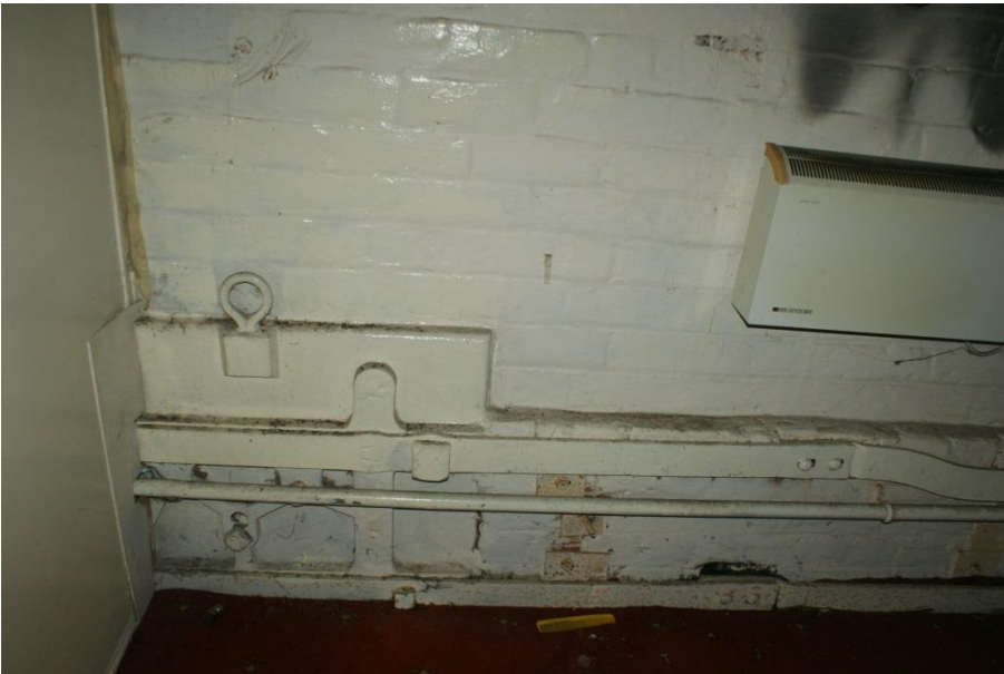
Plate 19 Possible machinery fittings within (F38a)
