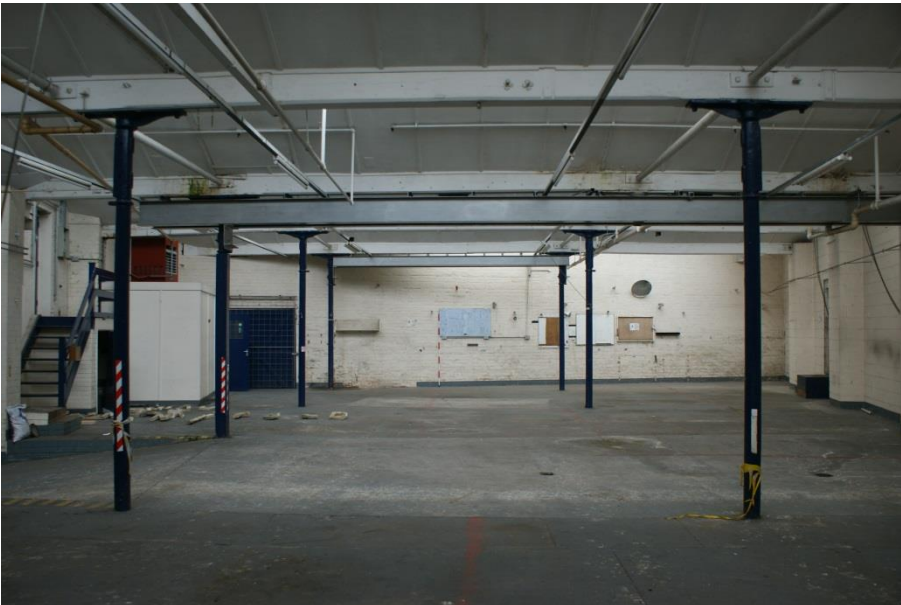
Plate 15 Former weaving shed, Phase 2 (G48)
