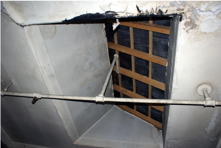
Plate 45 Phase 3 (S28), above modern suspended roof
