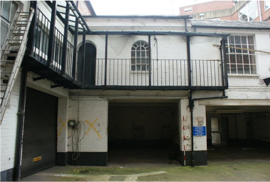
Plate 1 Two bay Phase 1 structure (Y2)
