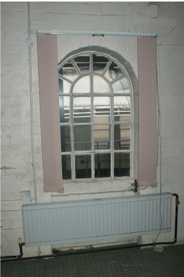
Plate 2 Fanlight windows, Phase 1 (GF1)
