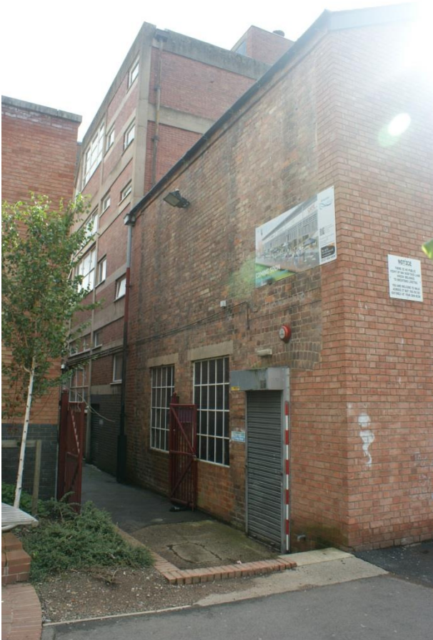
Plate 16 Four bay, two storey structure, Phase 2
