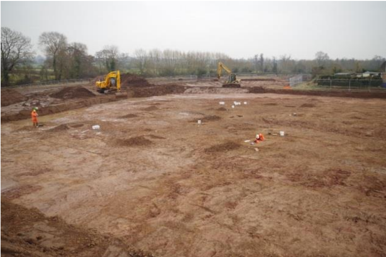
Plate 3 Area 2 looking south
