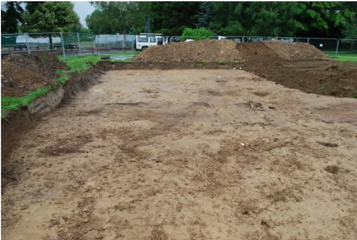
Plate 6 The West side of the excavation area view north showing modern service trench and disturbance
