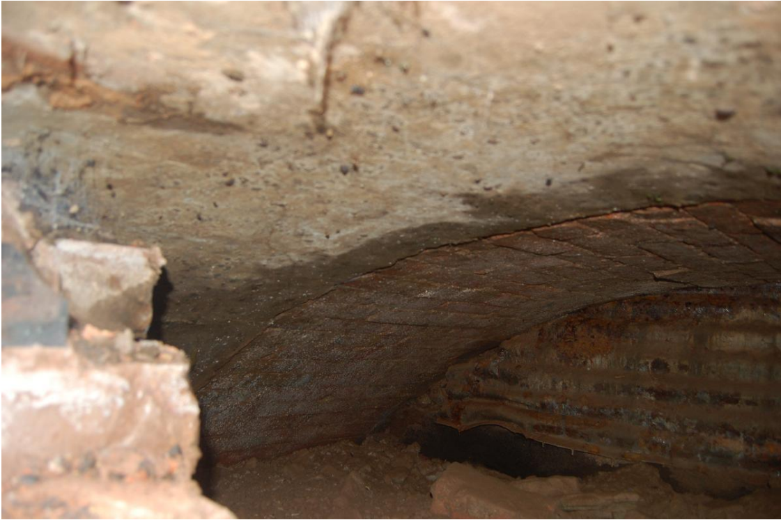
Plate 27 Access Hole 1 (Trench 13), view south-west
