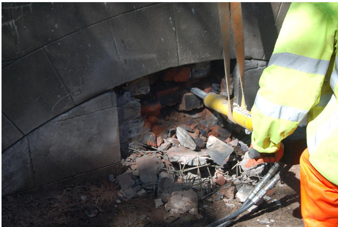
Plate 25 Access Hole 1 (Trench 13), removal of concrete and brick infill
