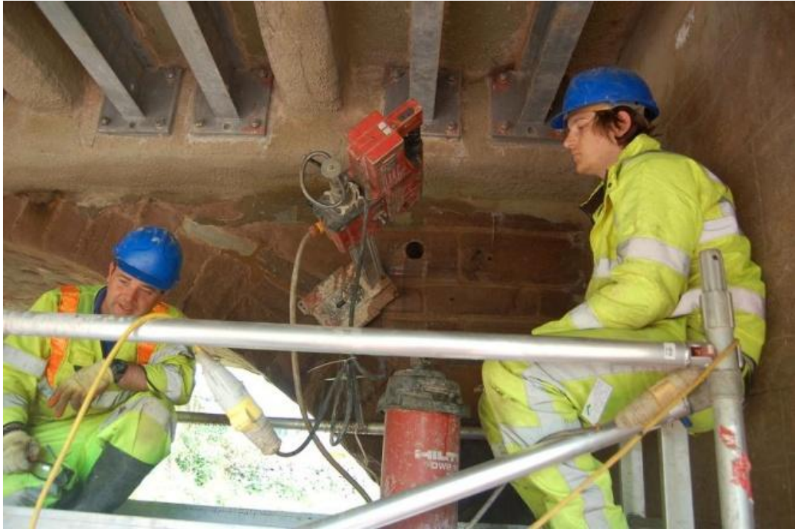
Plate 23 Spandrel core below Span 6 north pier
