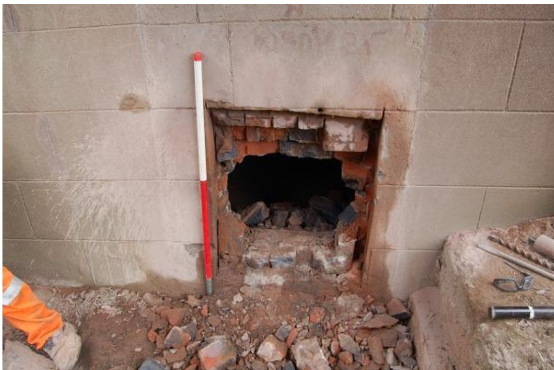
Plate 30 Access Hole 2 (Trench 14) opened showing concrete and brick infill wall
