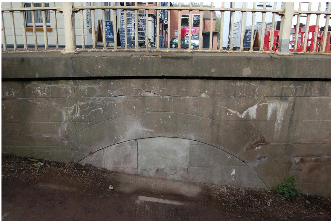
Plate 29 Access Hole 1(Trench 13) reinstated
