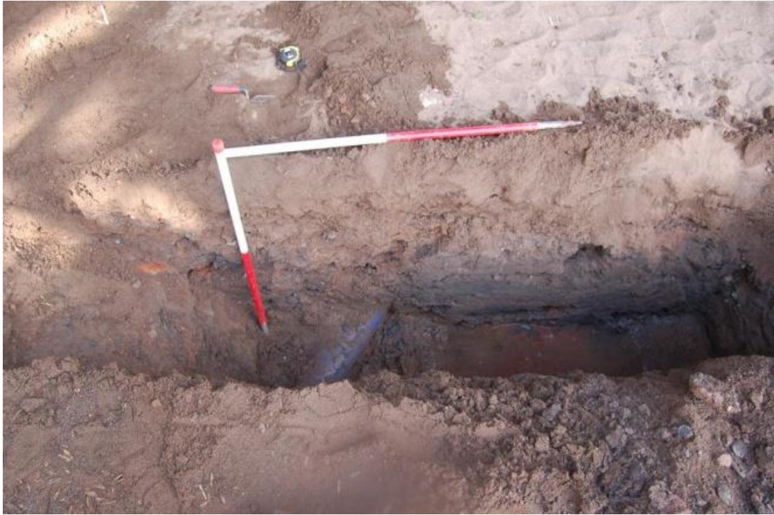
Plate 17 Trench 10 east facing section showing water main and clay deposits
