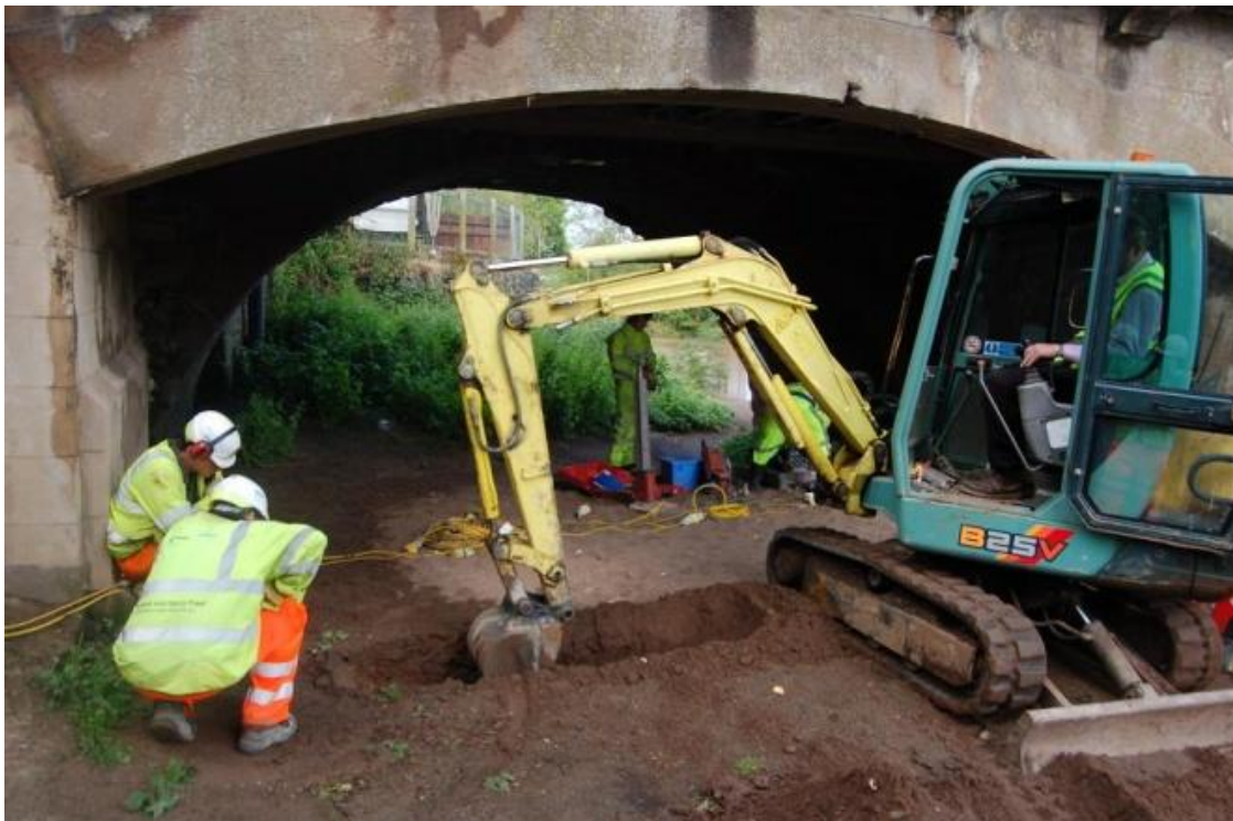
Plate 16 Trench 10 during excavation adjacent to the southernmost bridge arch (Span 6)
