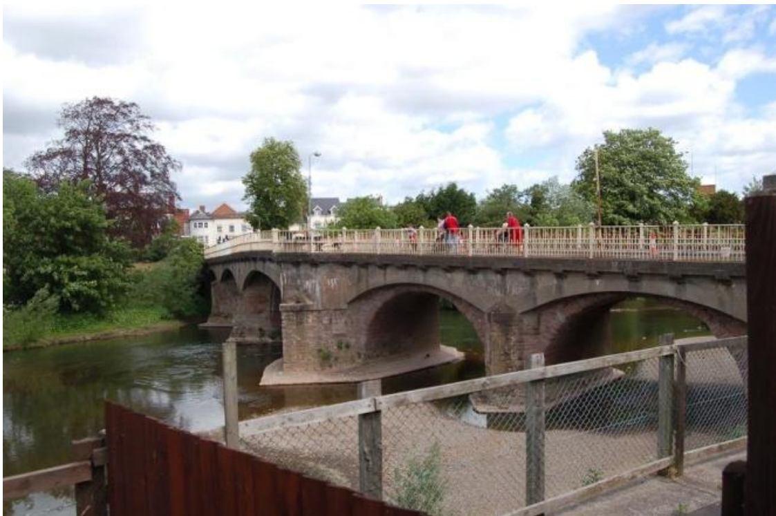
Plate 2 The west side of the bridge looking north-east
