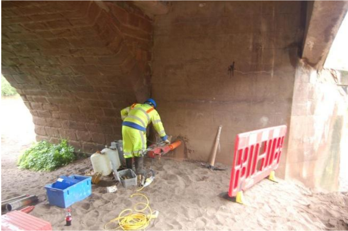
Plate 21 Coring for compression tests through southern pier looking north-west
