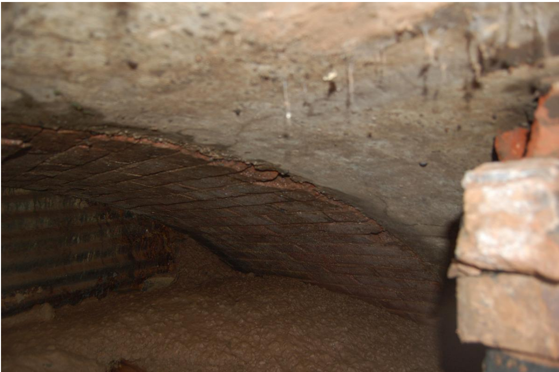
Plate 28 Access Hole 1 (Trench 13), view north-west
