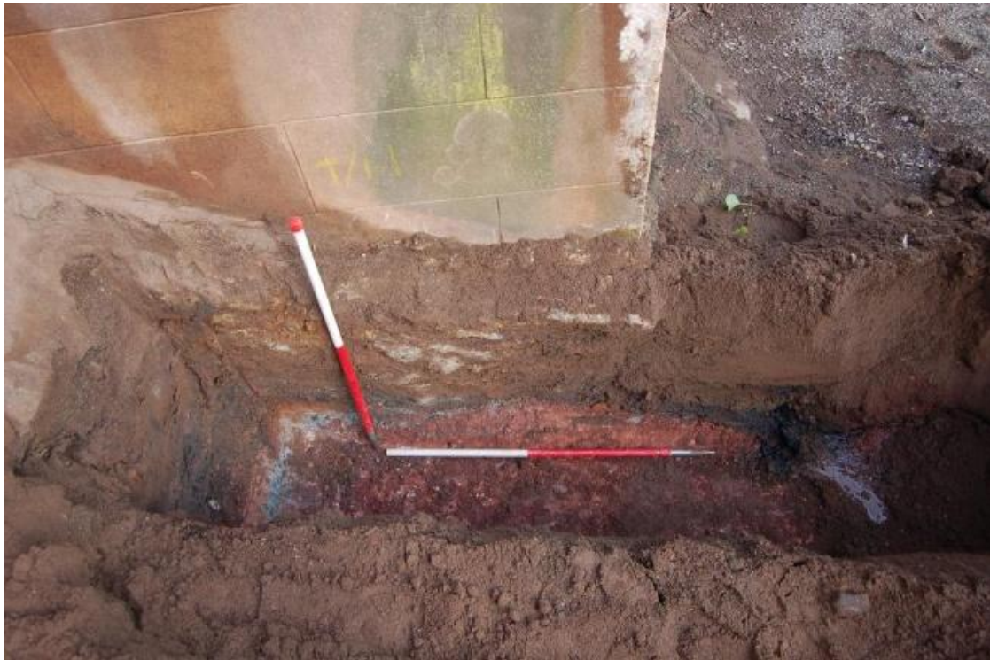
Plate 15 Trench 9 east facing section showing concrete foundations and natural mudstone at base
