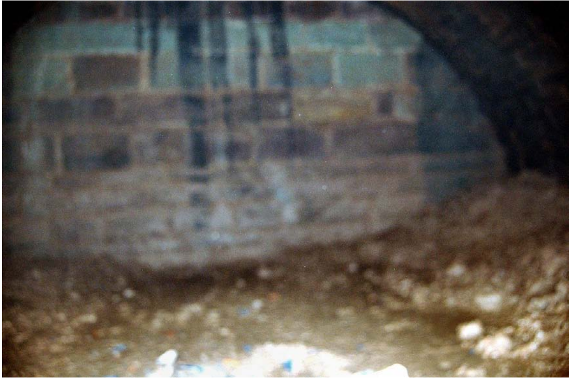
Plate 33 Access Hole 2 (Trench 14), view west (enhanced image)
