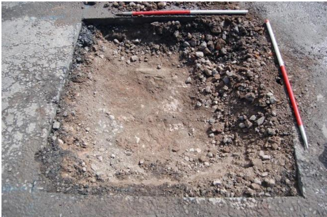
Plate 8 Trial hole 2 (Trench 4) showing concrete and hardcore at the base
