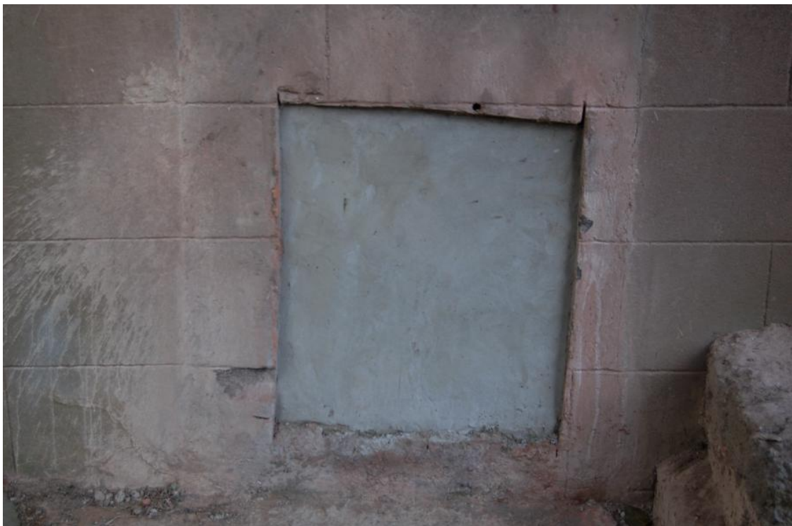
Plate 34 Access Hole 2 (Trench 14) reinstated
