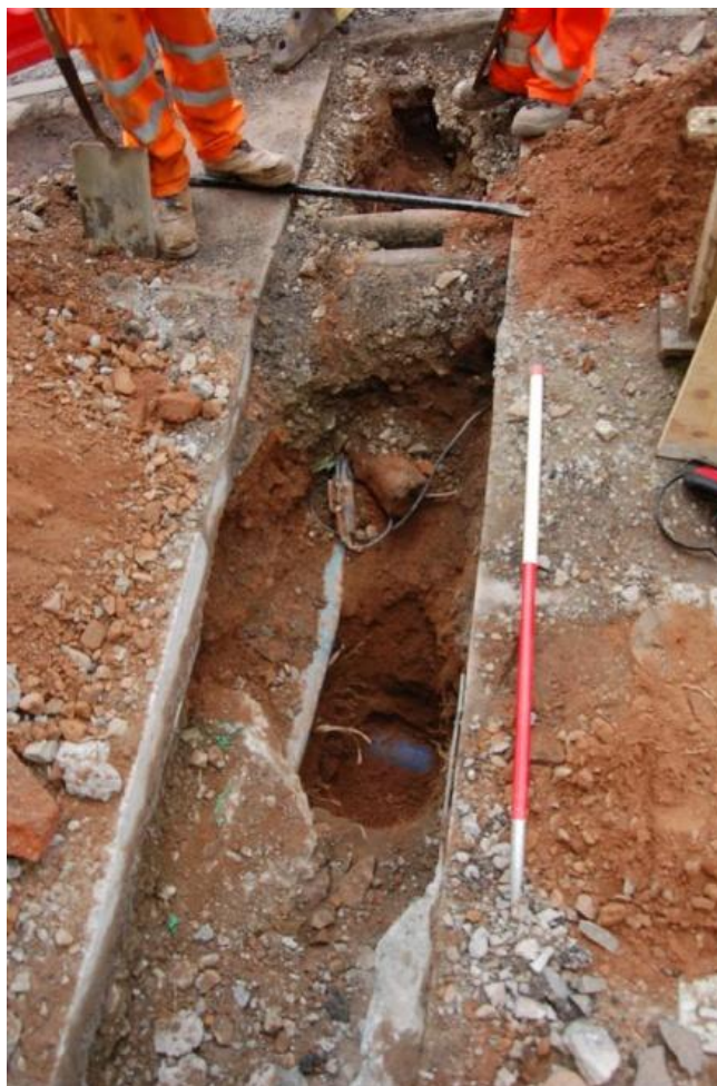
Plate 20 Base of Trench 12 looking west
