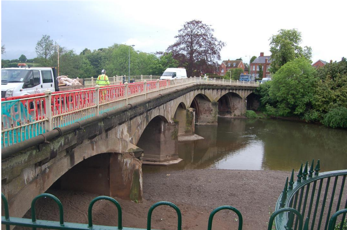
Plate 1 The east side of the bridge looking north
