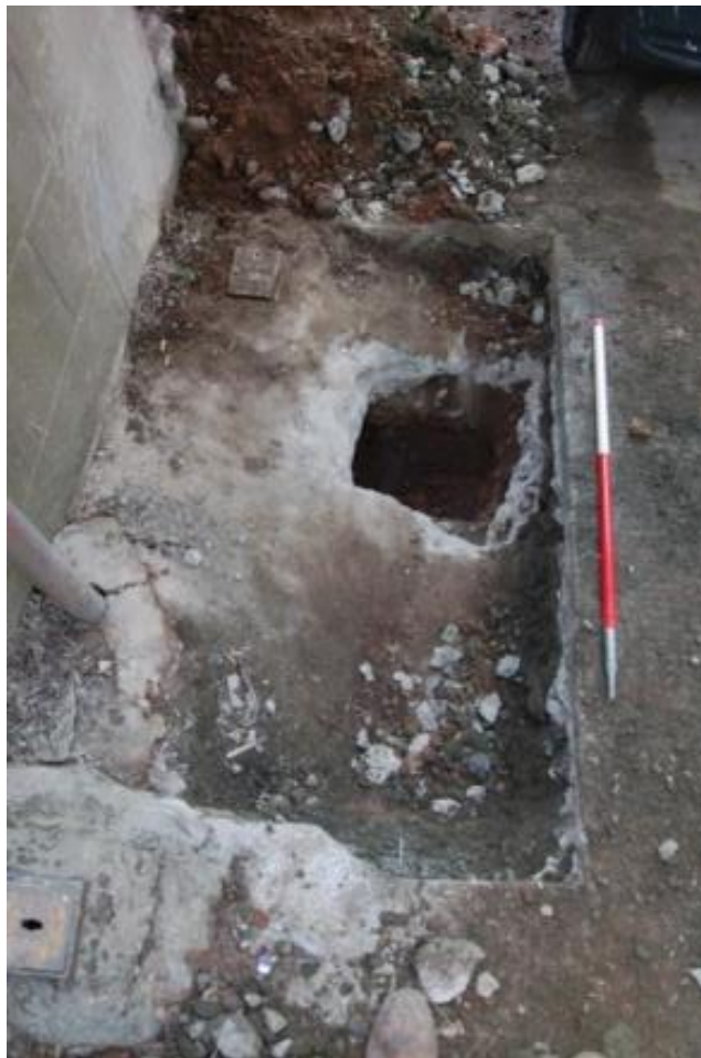
Plate 18 Trench 11 looking north showing concrete covering water services and slip road, and 0.50m square trial hole cut through concrete
