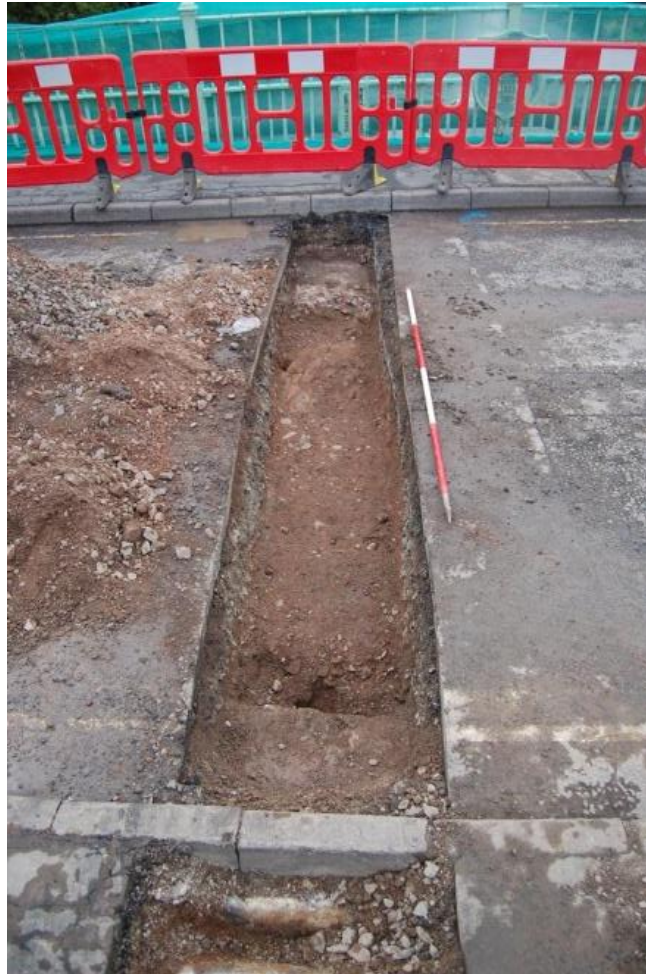
Plate 7 Span 3 in plan looking east showing sandstone surface and concrete widening
