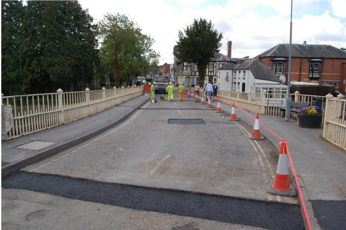
Plate 13 Trenches on the bridge during reinstatement, looking south
