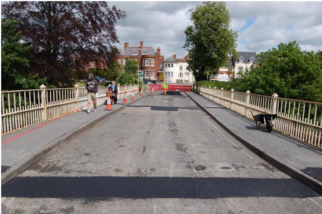
Plate 14 Trenches on the bridge after full reinstatement, looking north
