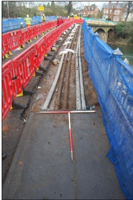
Plate 1 The pavement on the east side of the bridge looking north
