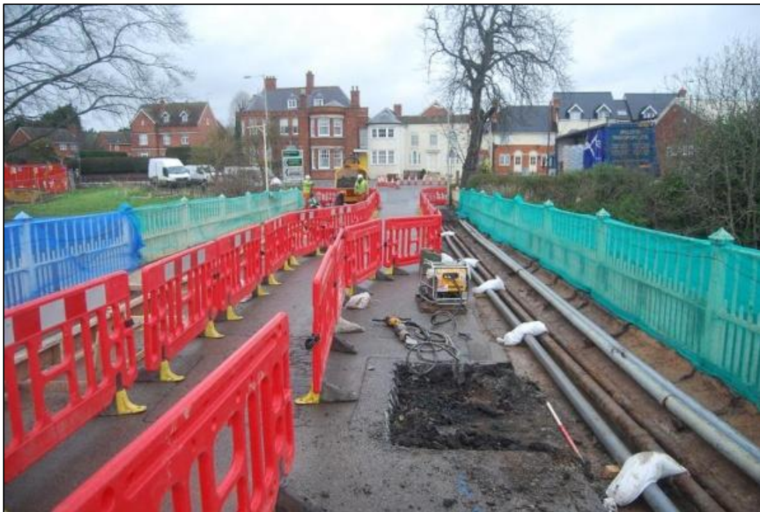
Plate 12 Trench 2 location on bridge looking north
