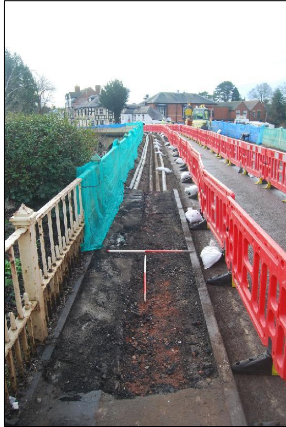
Plate 3 West pavement with tarmac and hardcore removed, showing services, looking north
