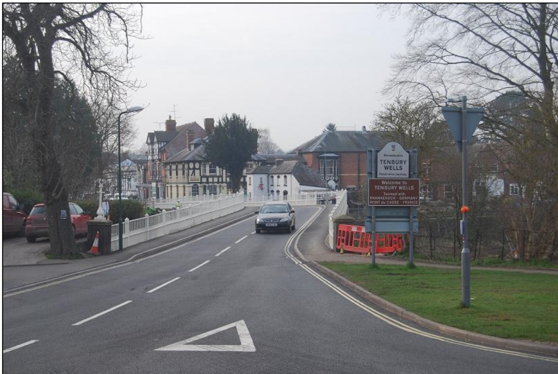
Plate 26 Tenbury Bridge reopened after works to carriageway
