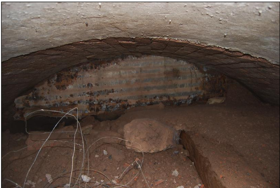
Plate 18 Internal shot of Access Hole 1 showing shuttering against original wall
