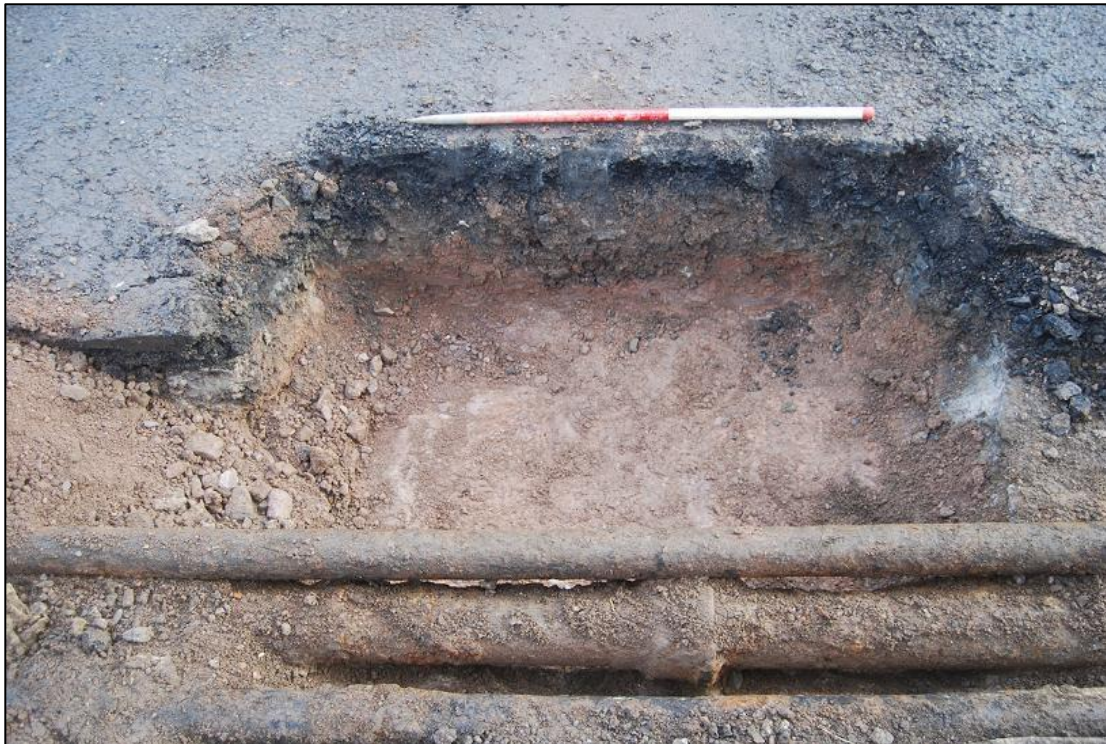
Plate 7 West facing section of Trench 1 road surfacing layers above original sandstone bridge
