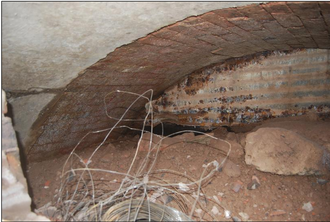
Plate 19 Side view of concrete and brick sections of arch with Access Hole 1 looking south
