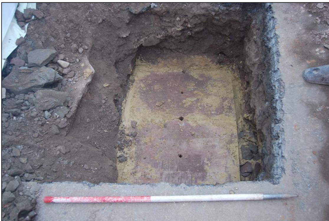
Plate 16 Trench 2 keystones replaced and grouted
