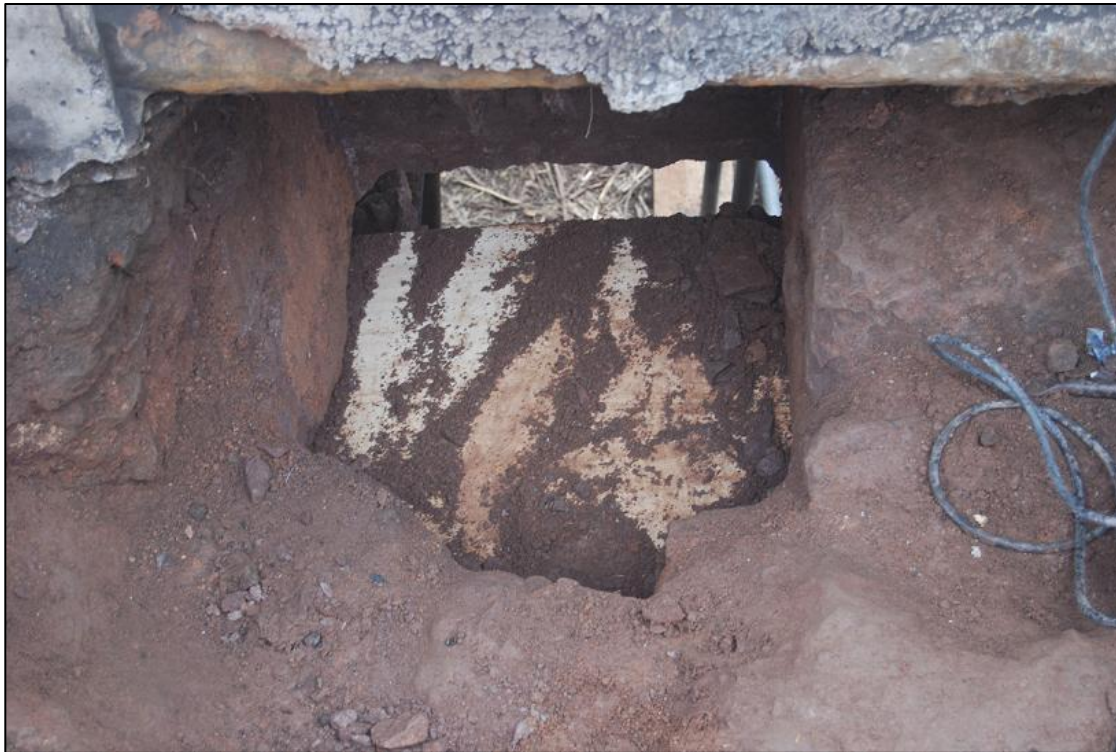
Plate 9 View of Trench 1 with damaged keystones removed, showing layers of bridge and extant keystones. Scaffolding platform below to stop sandstone falling through
