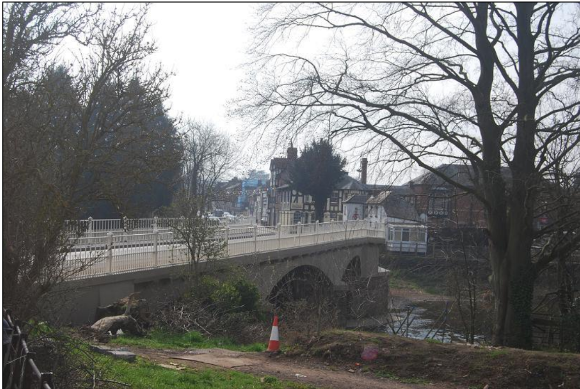
Plate 25 View of the west side of the bridge looking south
