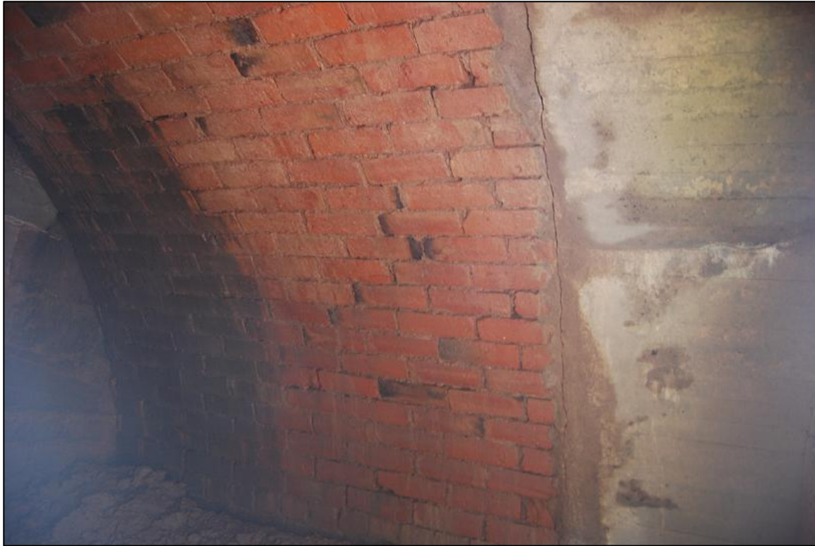
Plate 21 Access Hole 2 side view of arch, showing brick and concrete sections
