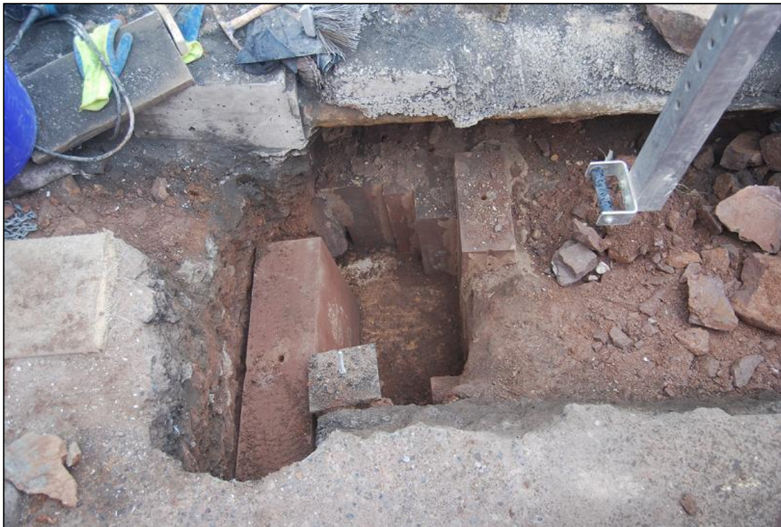
Plate 10 New keystones in place and partially grouted
