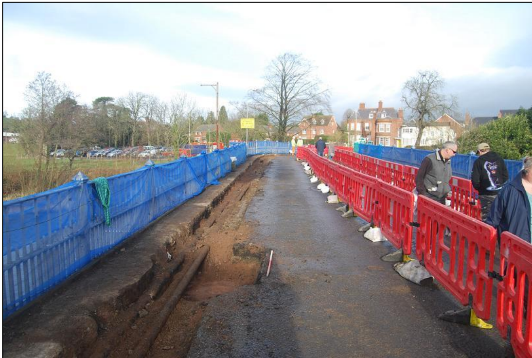
Plate 6 Location of Trench 1 looking north
