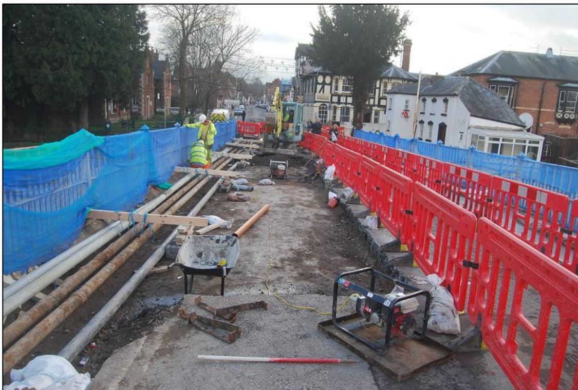
Plate 2 Removing tarmac and hardcore overlying the concrete extension looking south
