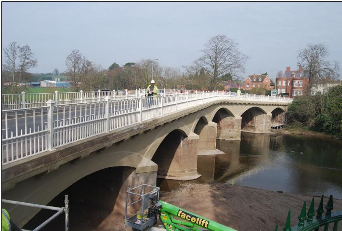
Plate 24 East side of bridge after works are complete looking north-west
