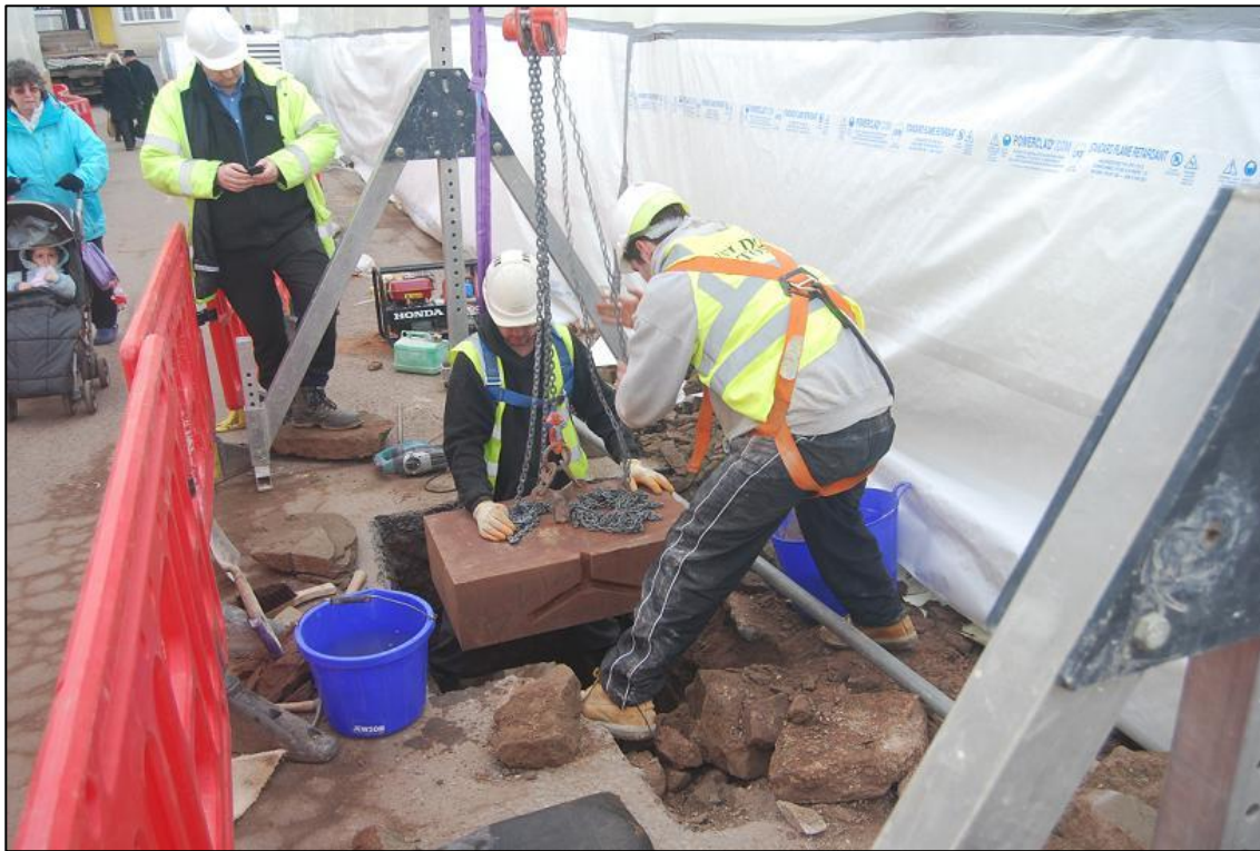
Plate 15 Replacing the keystones in Trench 2 using a winch
