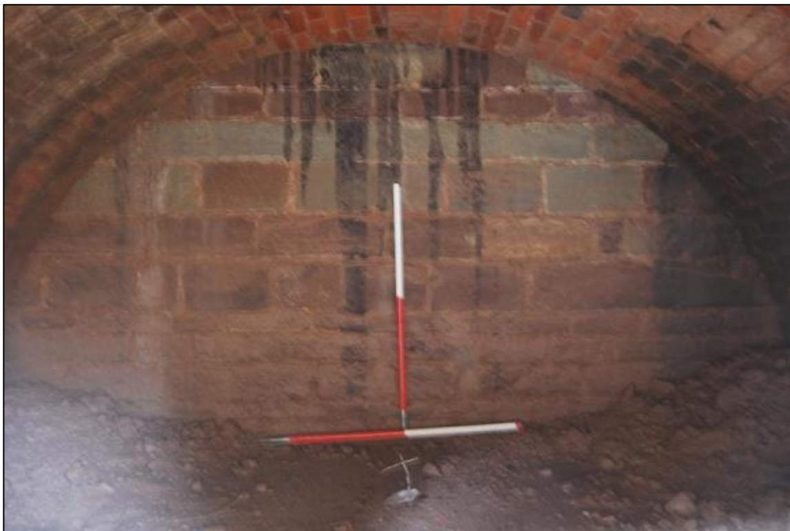
Plate 20 Access Hole 2 showing original sandstone wall at back of the arch
