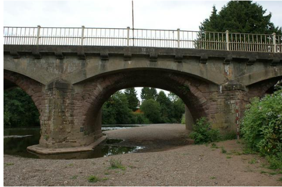
Plate 4: Sandstone bridge, span 5 from the west
