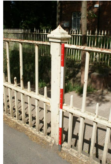
Plate 10: 1908 period railings and post
