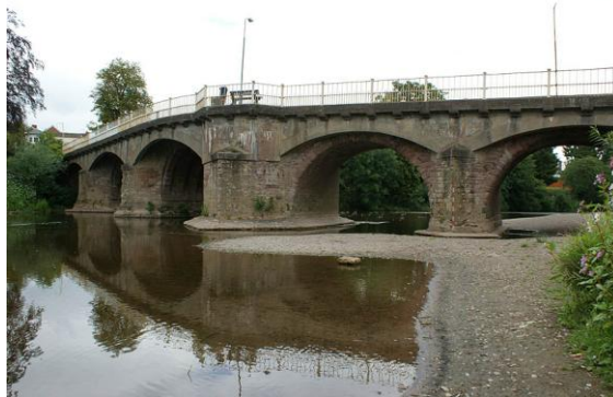
Plate 1: Tenbury Bridge, July 2011, from the south west
