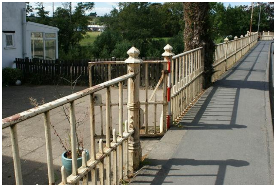
Plate 8: Telford period cast iron posts
