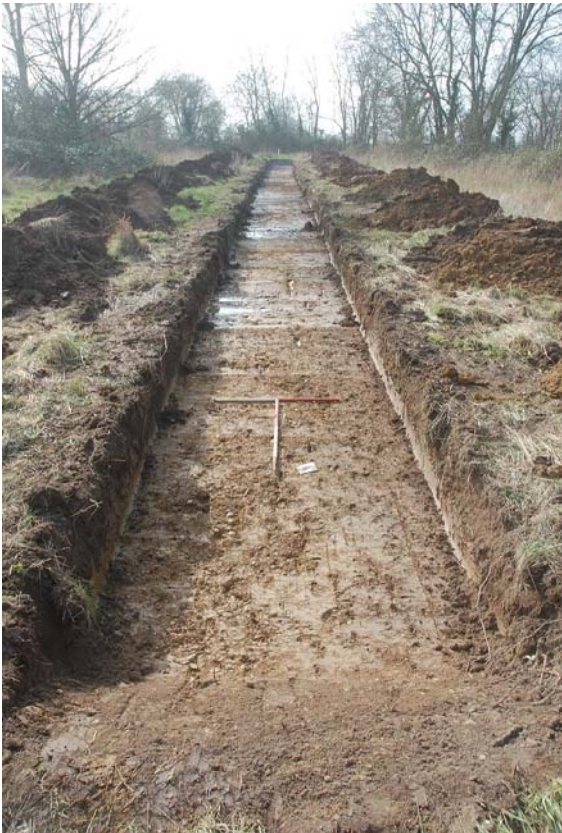
Plate 5: General view of Trench 12, facing south-west
