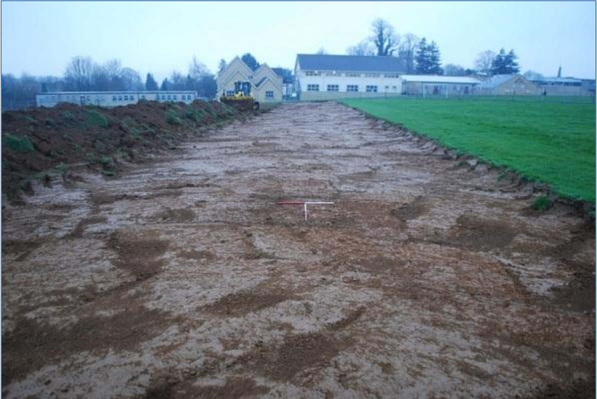
Plate 3 Initial topsoil strip of area in progress
