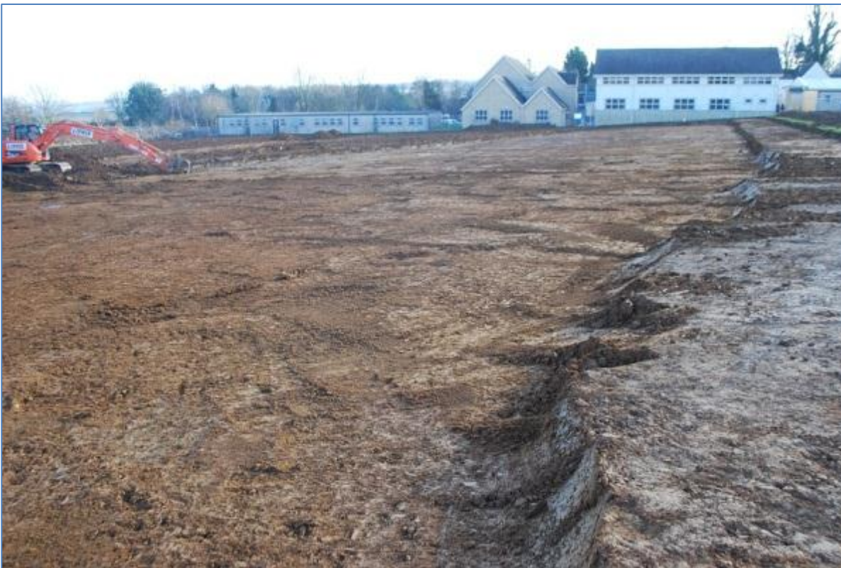
Plate 8 General shot of overall area stripped of topsoil and subsoil looking south east
