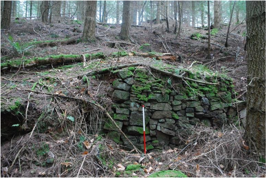
Plate 15 Workings to the north of Mapleford Engine Coal Level, looking north east
