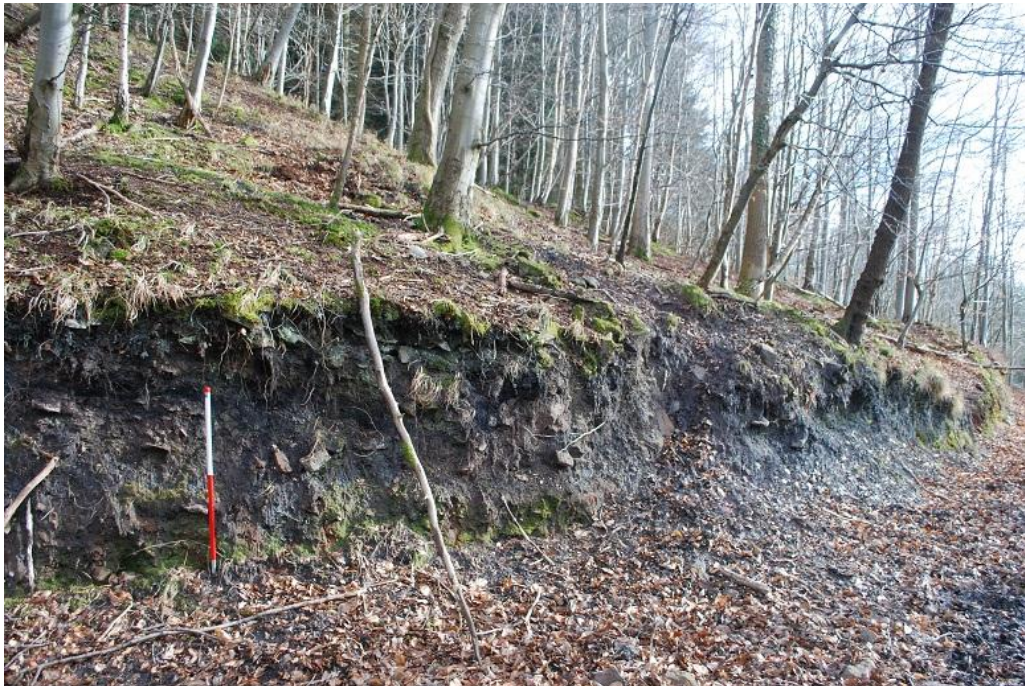
Plate 4 Spoil deposits associated with Mapleford Engine Coal Level as seen in section, looking north east
