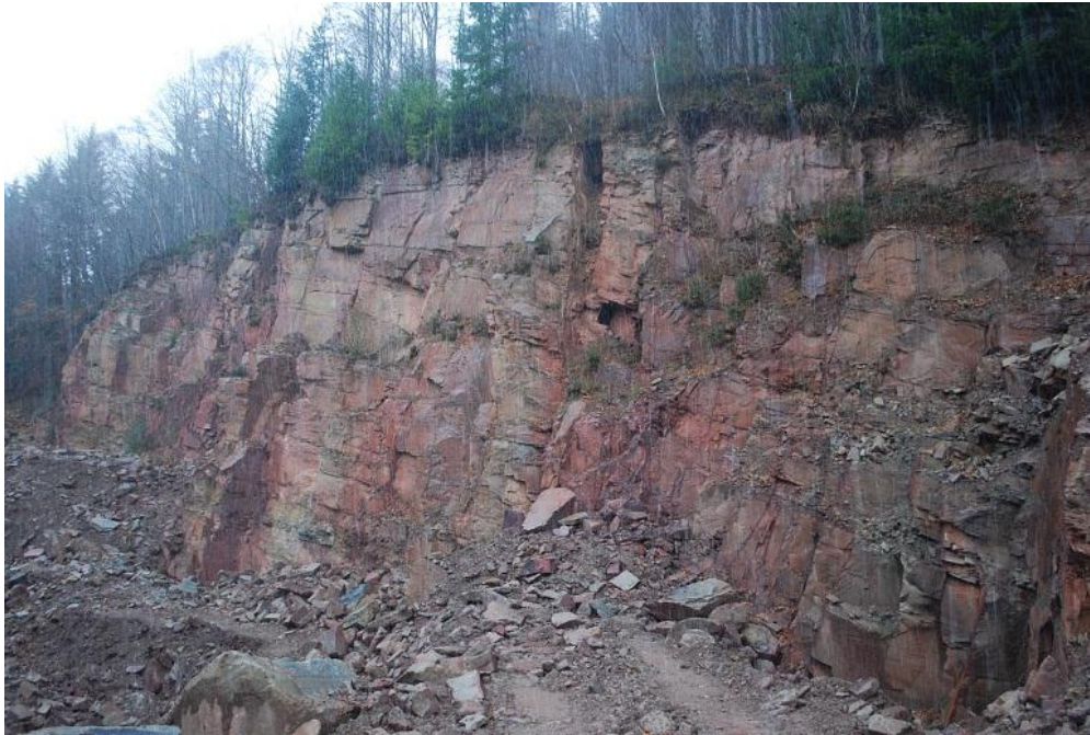
Plate 9 The working face of Mine Train Quarry with two adits associated with AHA3 visible, looking north west
