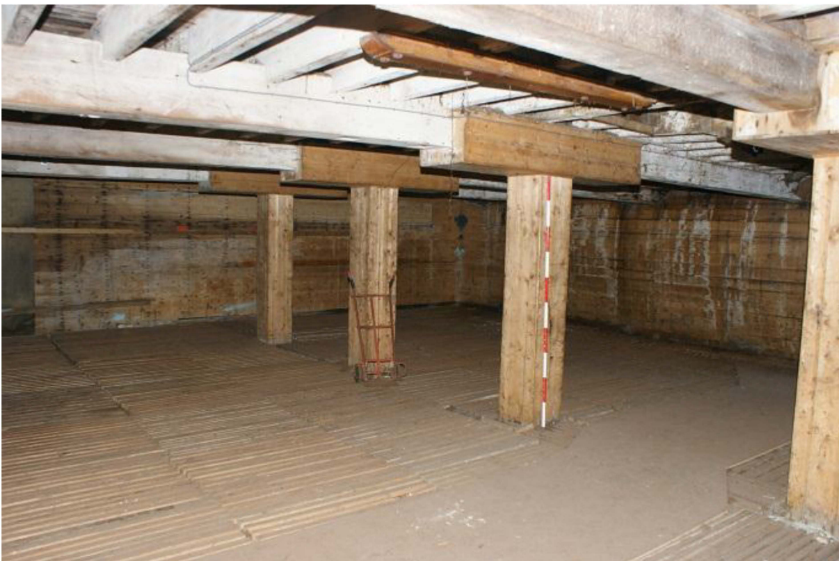
Plate 10 Larger room on the third floor of the mill looking south-east
