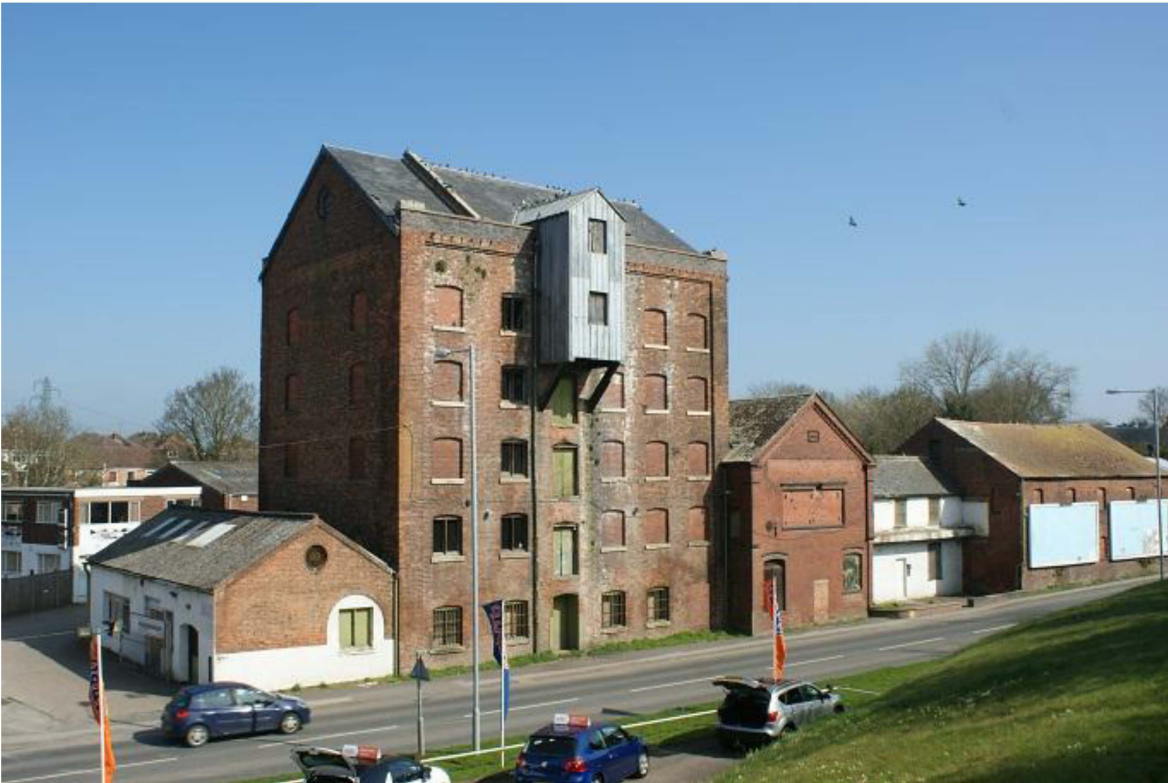
Plate 5 The mill and associated buildings looking north-east
