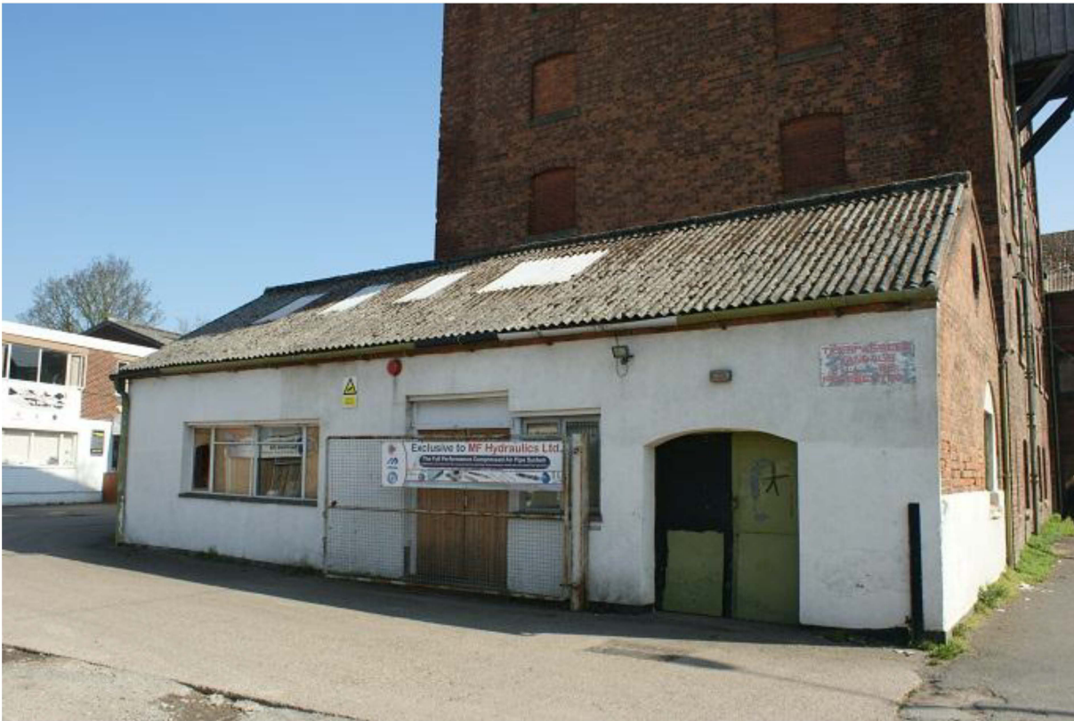
Plate 1 Possible grain drying building looking north-east
