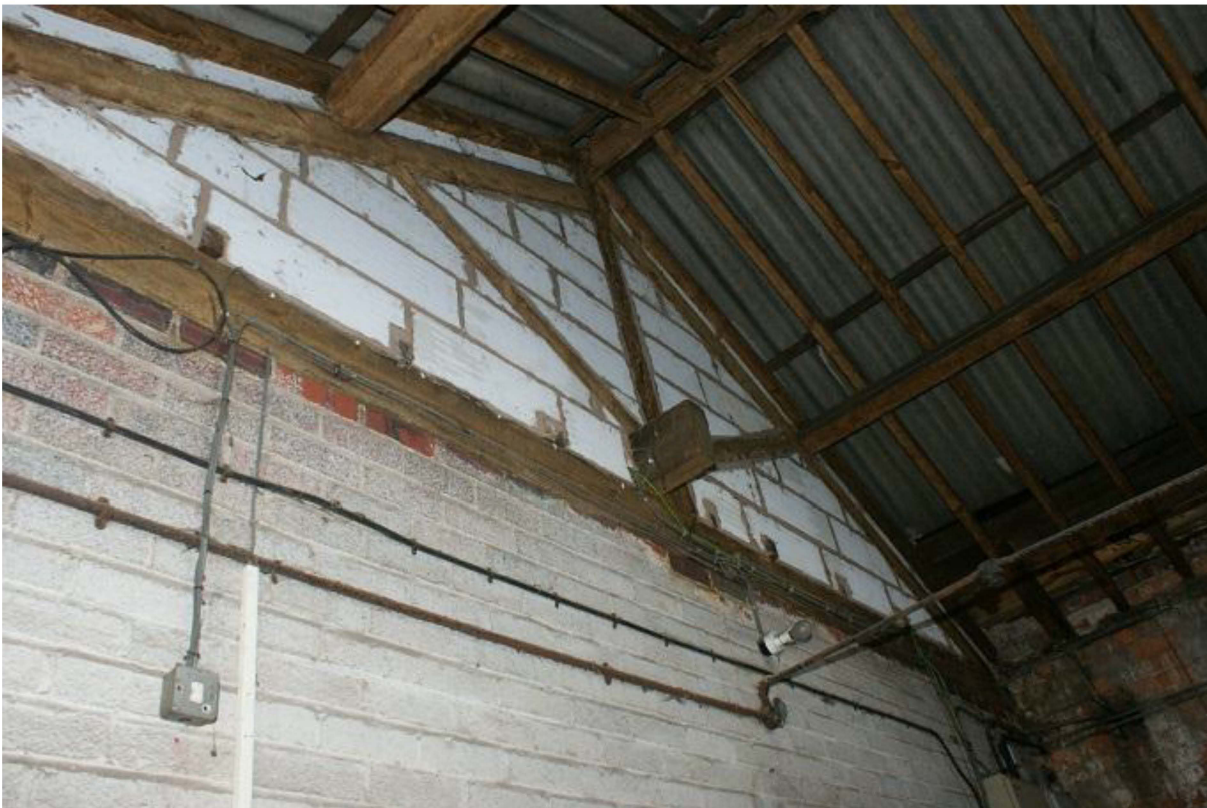
Plate 2 Roof truss of possible grain drying building looking north-east
