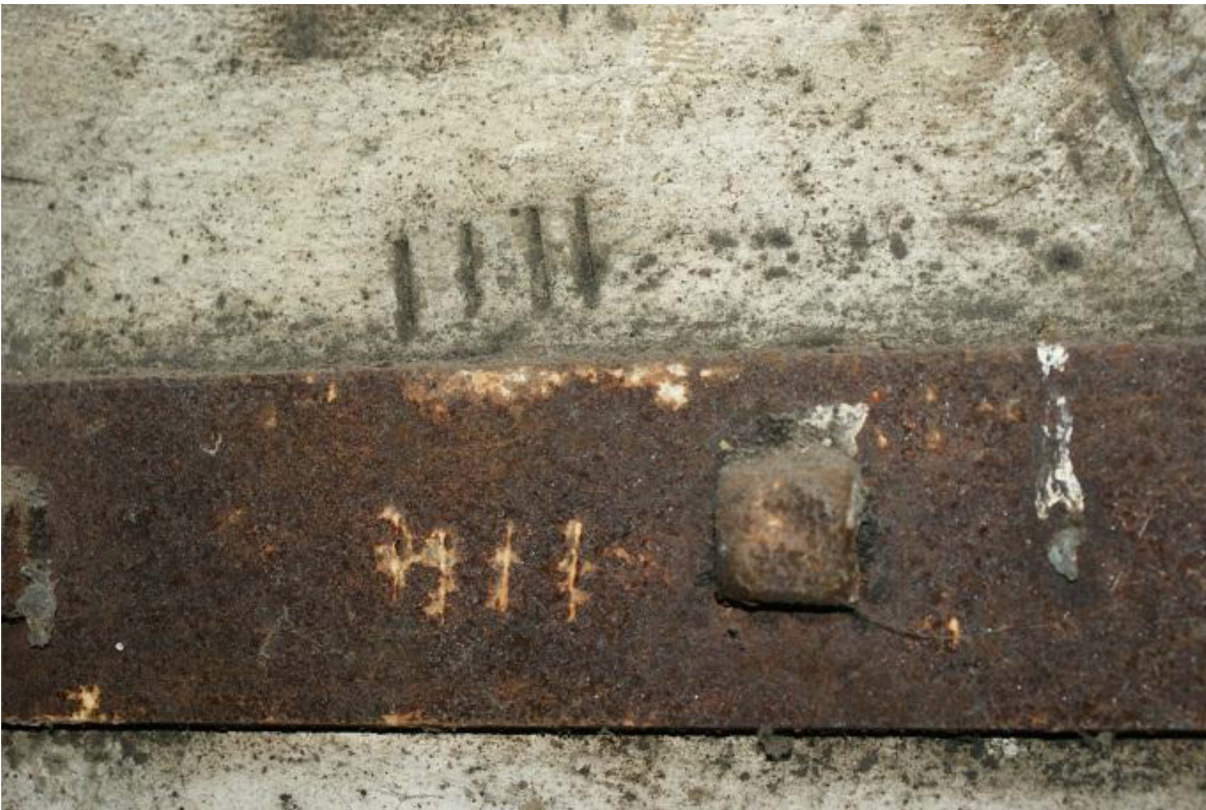
Plate 7 Construction marks on roof trusses
