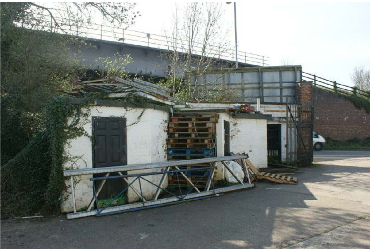
Plate 32 c 1942 single storey buildings, looking south
