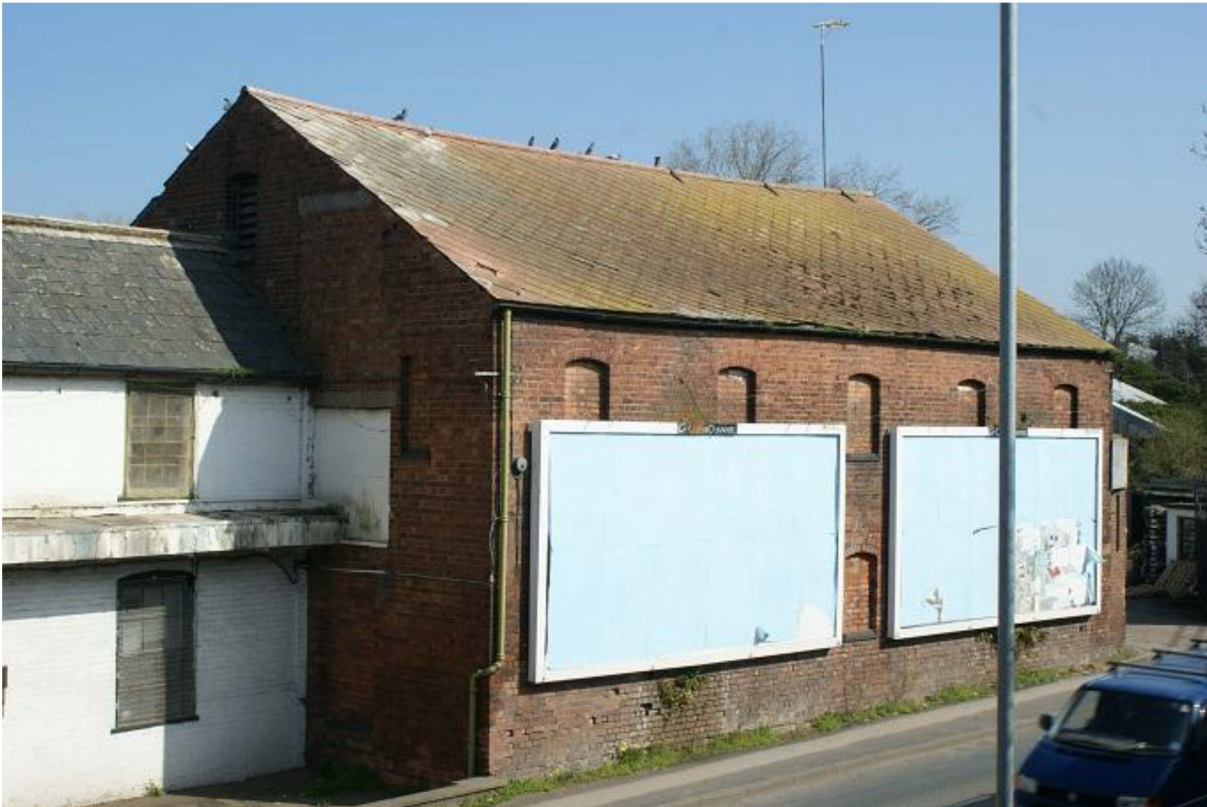
Plate 17 Former storage building, looking north-east
