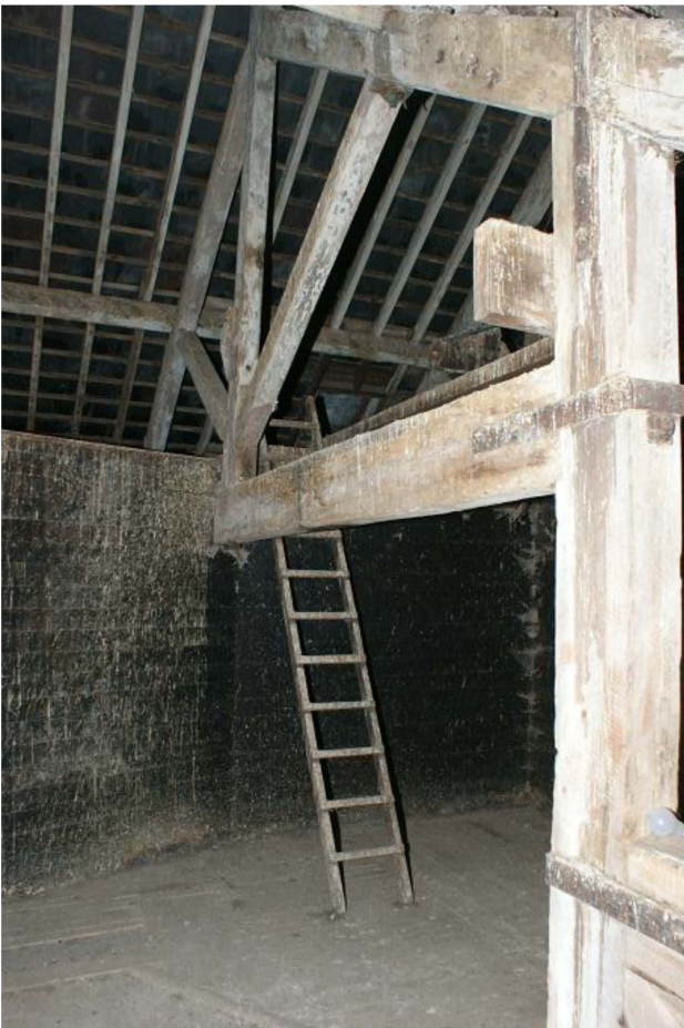
Plate 6 Roof truss visible on the sixth floor looking north-east
