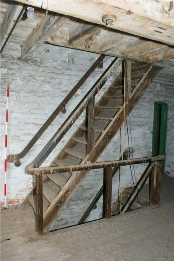
Plate 11 Inserted staircase, on the third floor looking north-west
