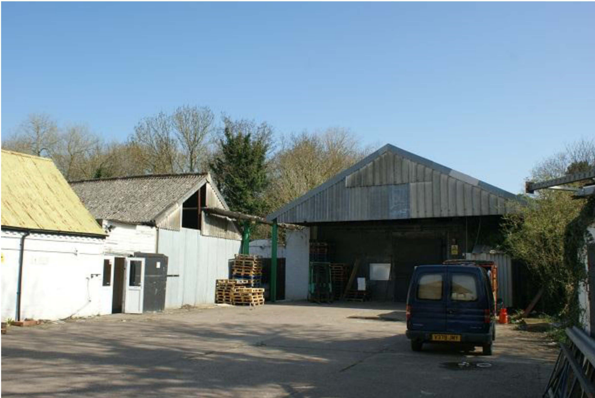
Plate 33 Post 1950s storage units, looking north-east
