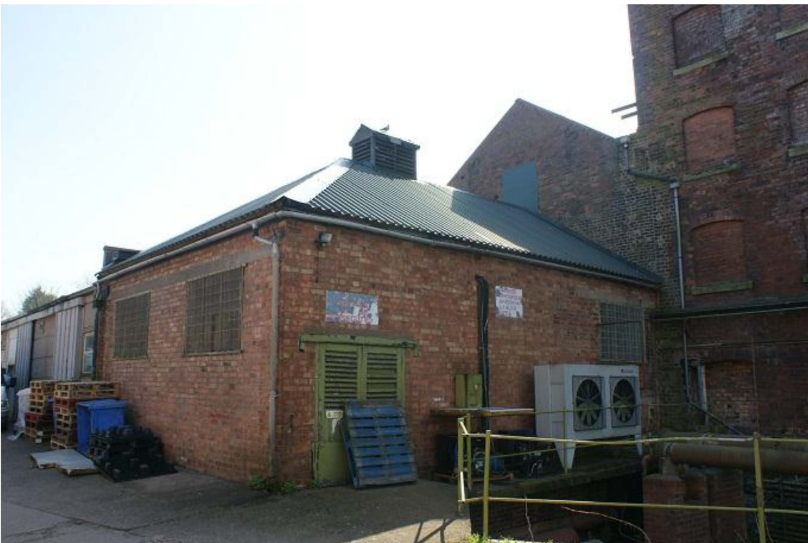
Plate 24 1905-28 cooling building, looking south-east
