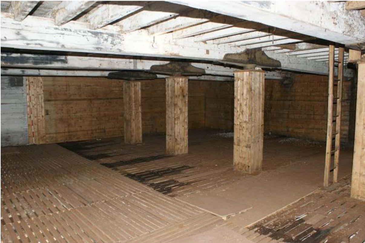
Plate 9 Larger room on the fifth floor of the mill looking south-east
