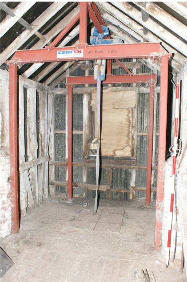
Plate 4 Interior of the Lucam on the sixth floor looking south-east
