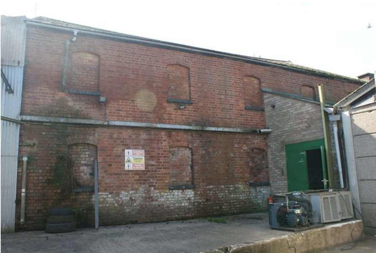
Plate 18 Rear of former storage building, looking south
