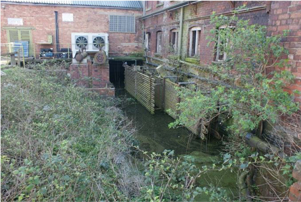
Plate 25 Cooling bars within the former mill race, looking south-east
