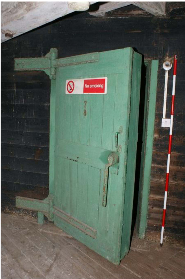
Plate 26 Insulating doors within the former mill building
