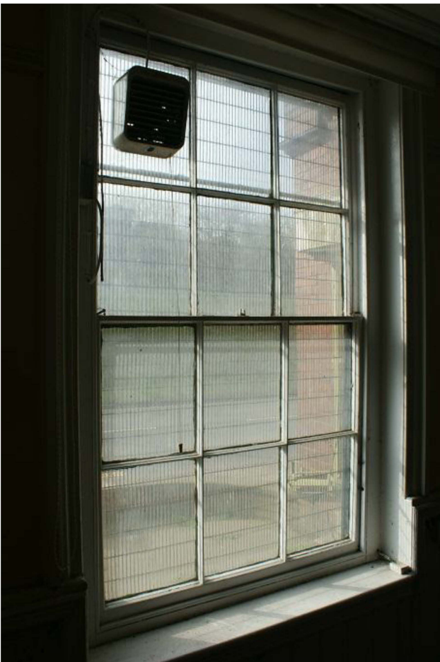
Plate 16 Sash windows on the first floor of the house looking south-west
