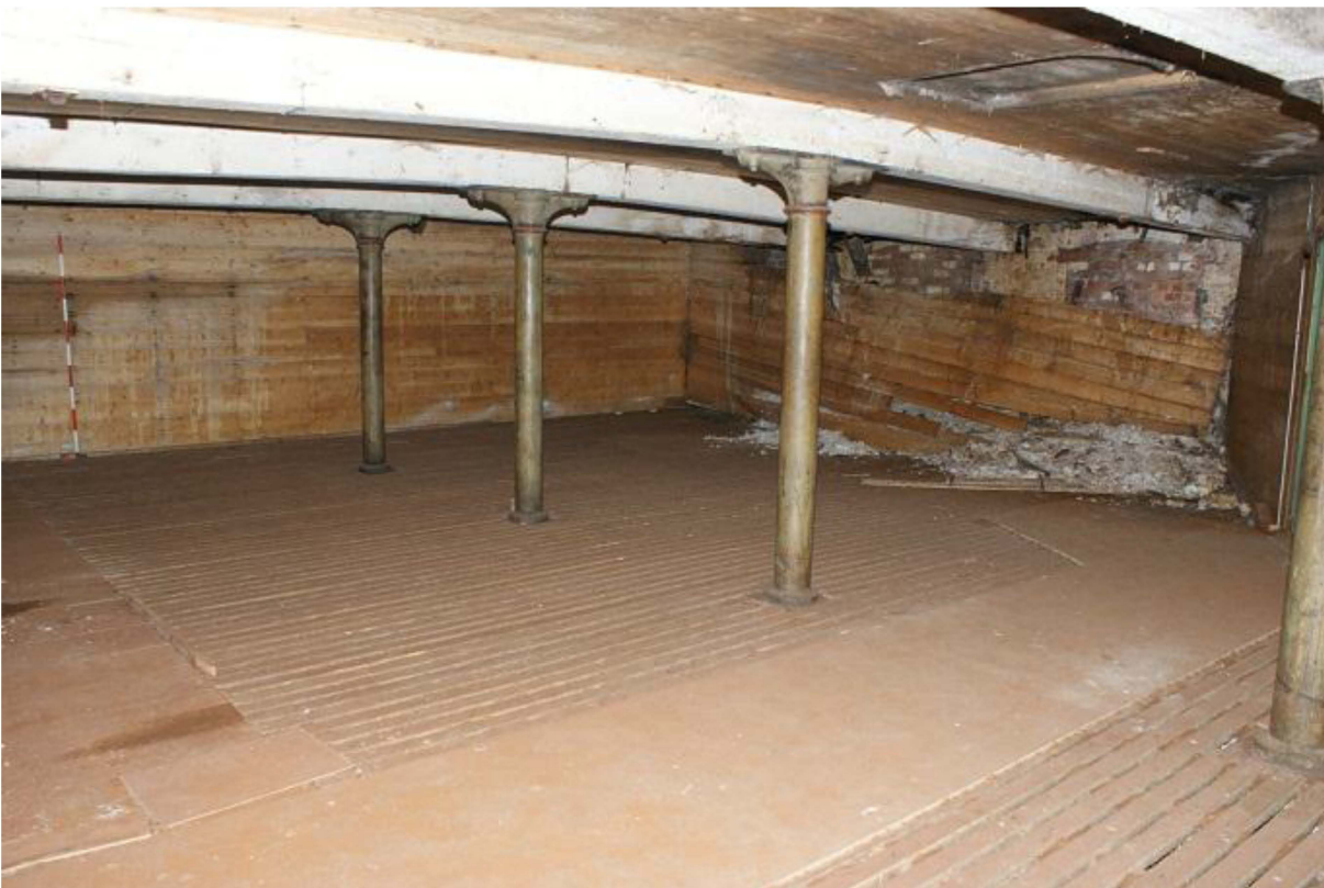
Plate 8 Larger room on the sixth floor of the mill looking south-east
