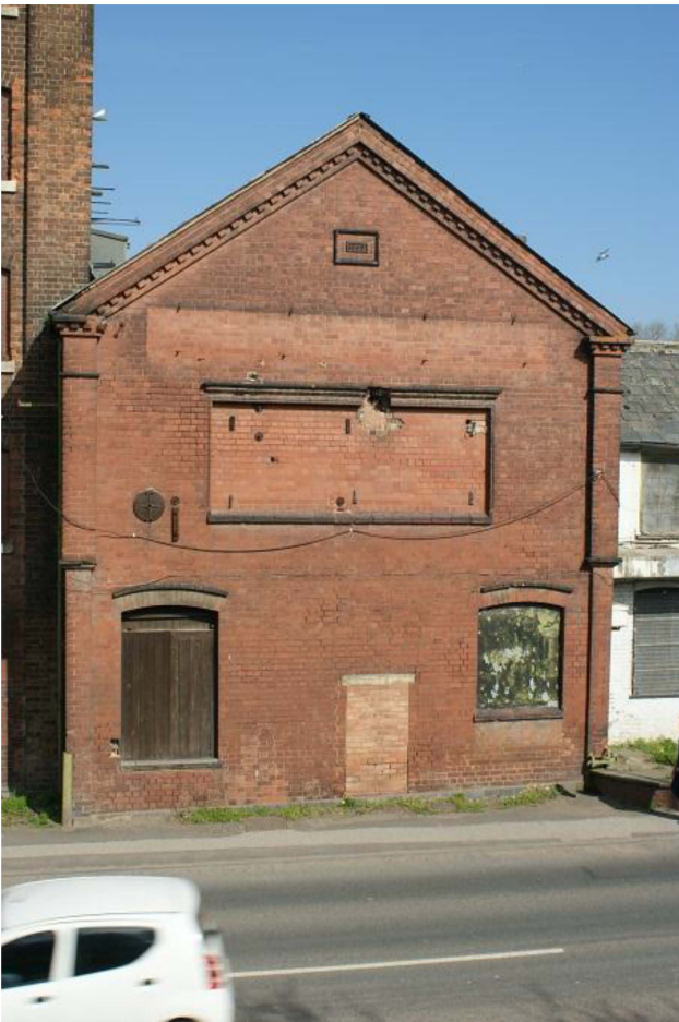
Plate 23 Gable of 1899 storage building, looking north
