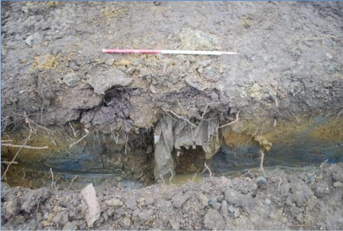
Plate 3 Modern soak away trench in Trench 1, backfilled with plastic and rubble. View southeast.
