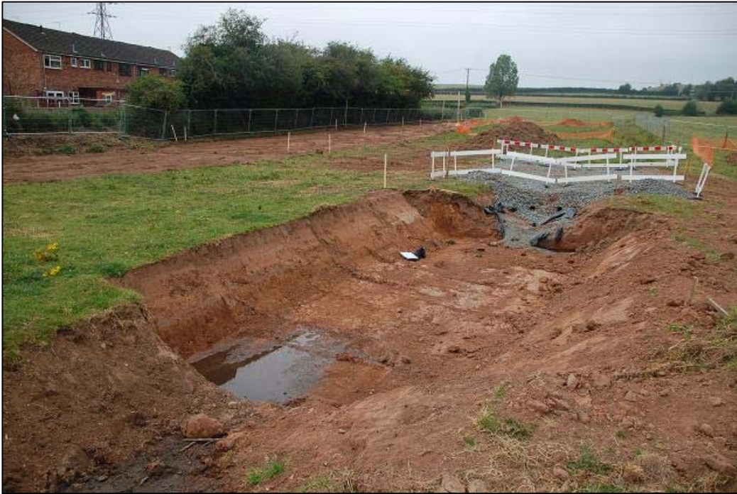
Plate 1 Trench 1 looking west
