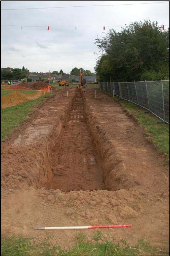
Plate 4 Trench 3 after excavation, looking east
