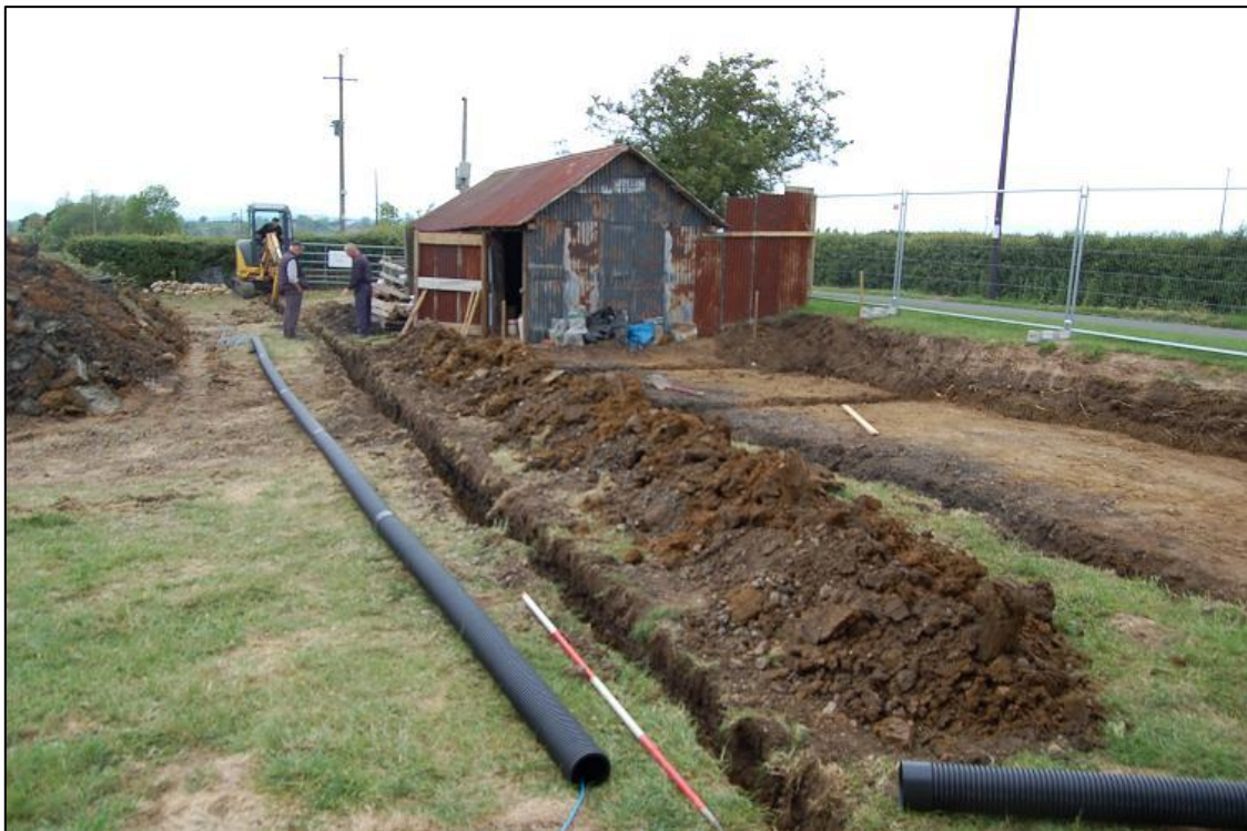
Plate 10 Service Trench 3 during excavation, view north-west
