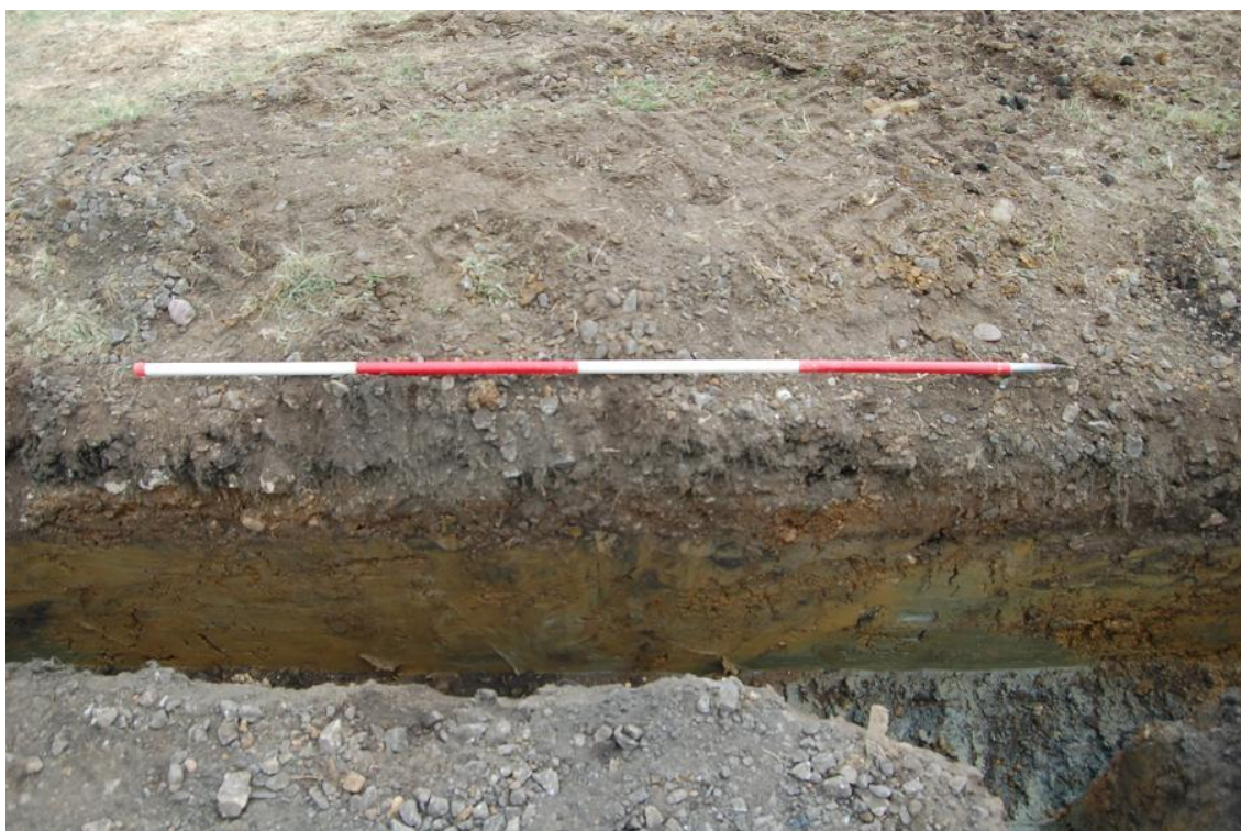
Plate 8 North facing section of foundation Trench 1 showing gravel and hardcore yard surface above natural sands and clays
