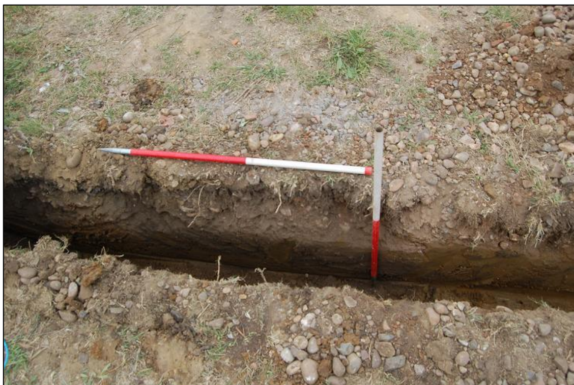
Plate 12 North facing section of Trench 3 showing modern pebble hardcore road surfacing (307) at entrance to the farm yard.
