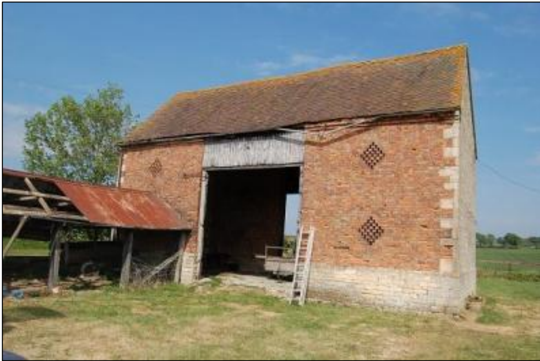
Plate 1 The threshing barn and cattle shelter shed before cattle shed demolition, view north-east
