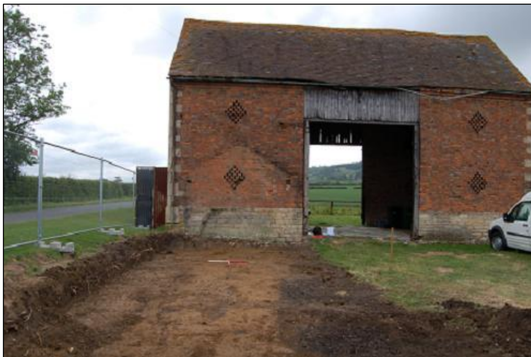
Plate 3 Trench 1 topsoil strip, view east
