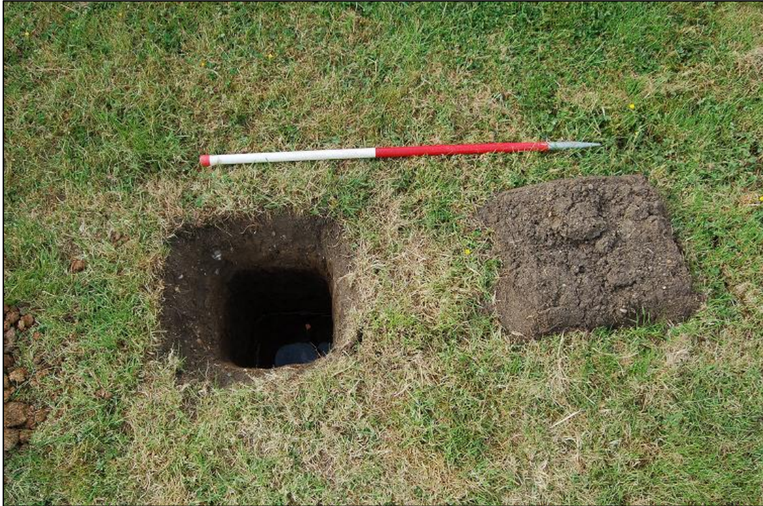
Plate 9 Example of one of the soakaway pits
