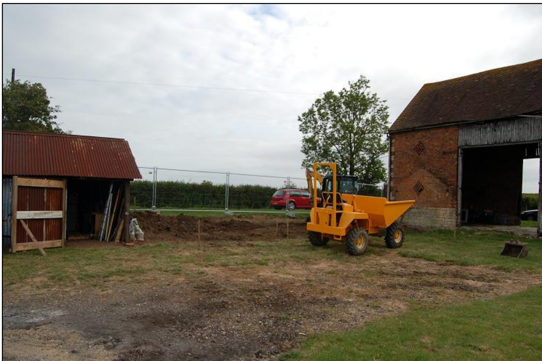
Plate 2 Location for new building prior to excavations commencing, view north-east
