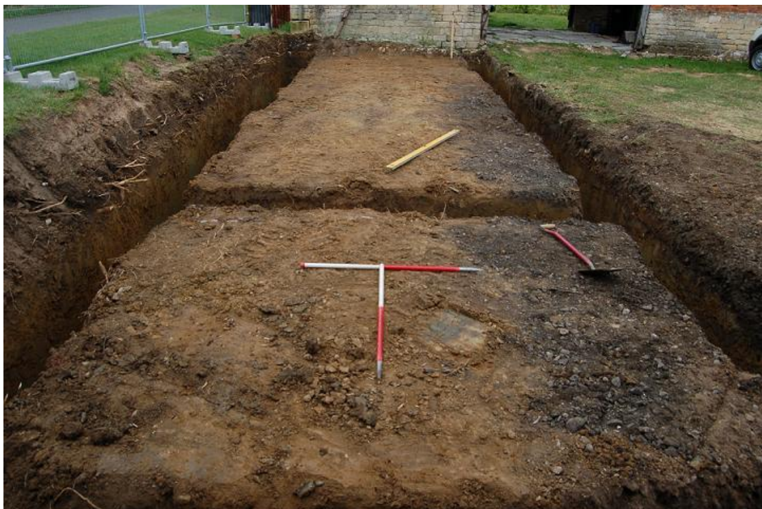
Plate 7 Trench 1 foundations complete, with hardcore surface (102) to the right, view east
