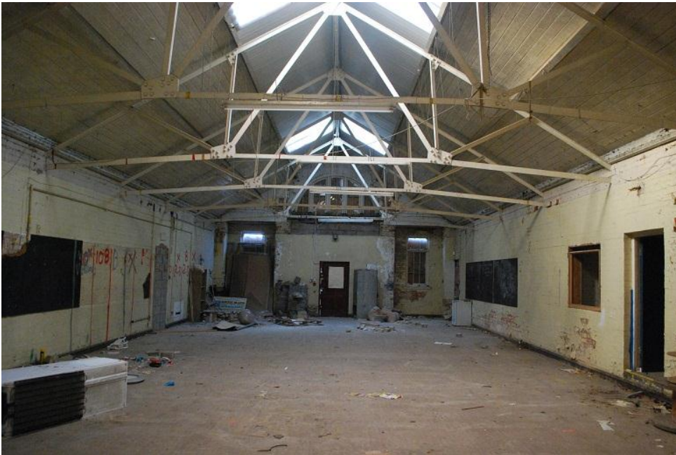
Plate 5 The hall, looking south west
