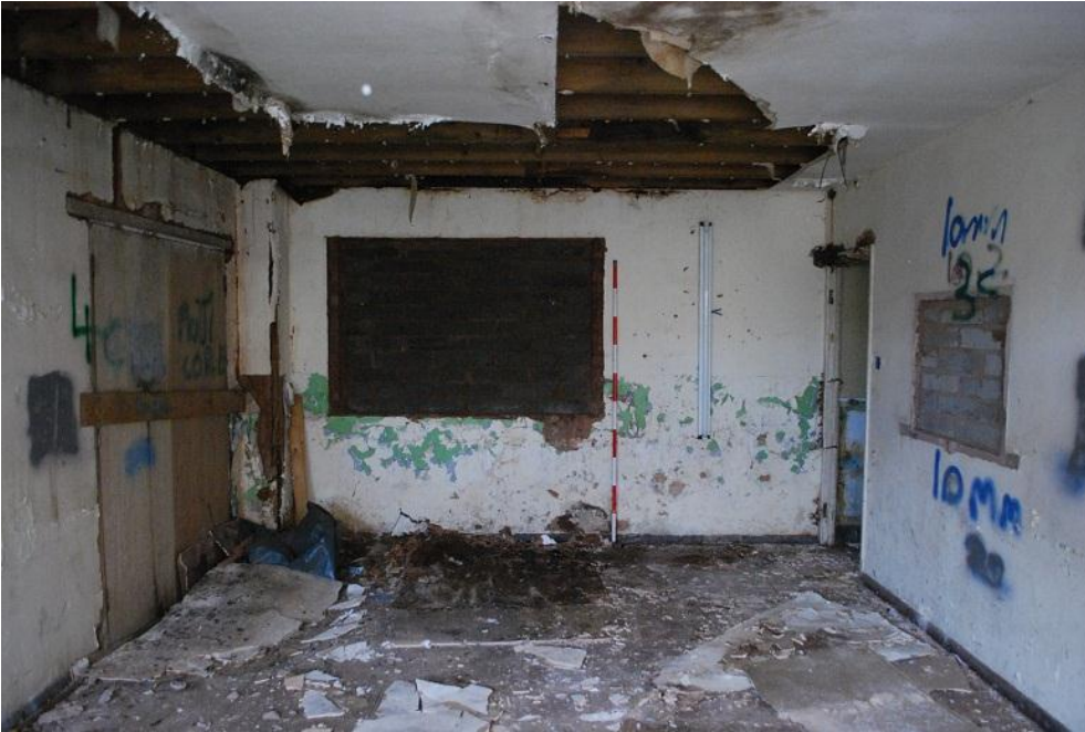
Plate 51 Interior of phase 2 structures, looking south east
