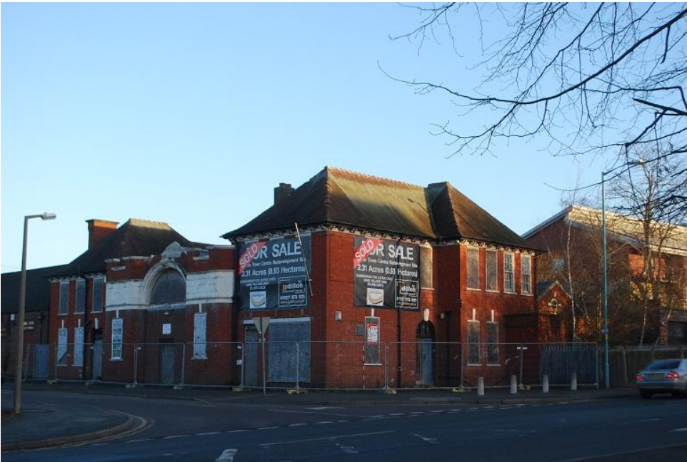
Plate 3 The Drill Hall looking north
