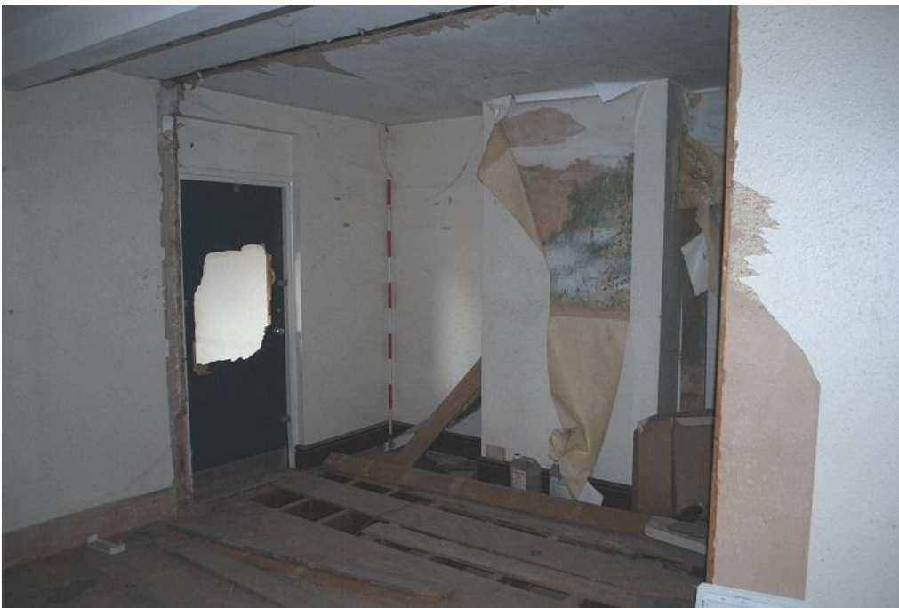
Plate 20 Bedroom of the drill sergeants' house, looking north east
