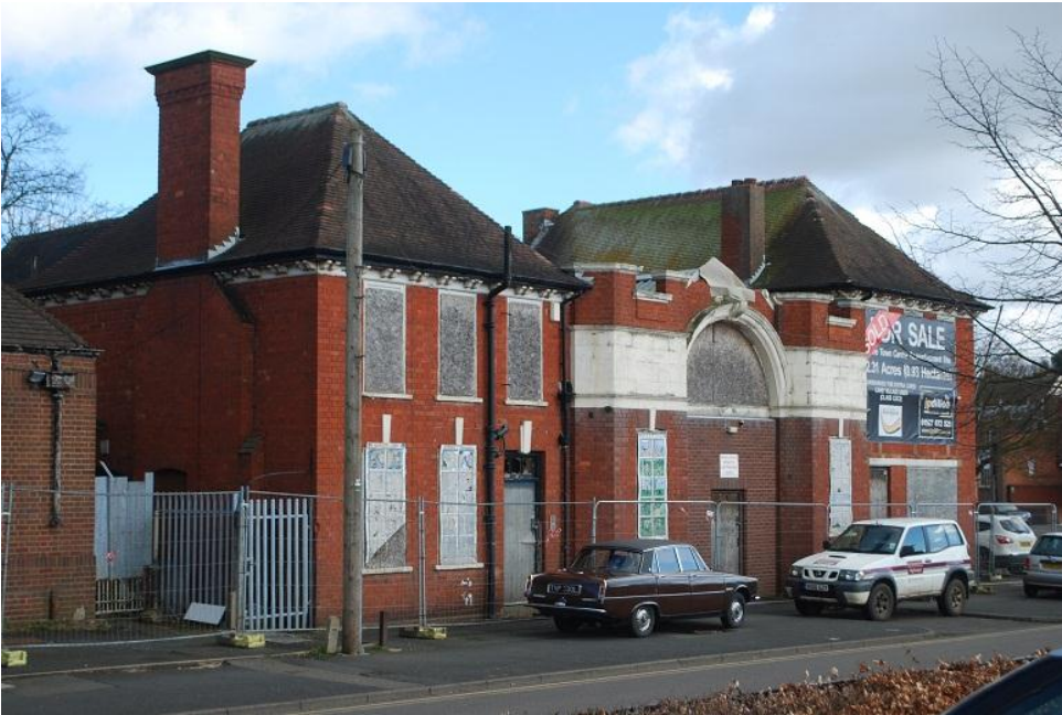
Plate 1 The Drill Hall looking east
