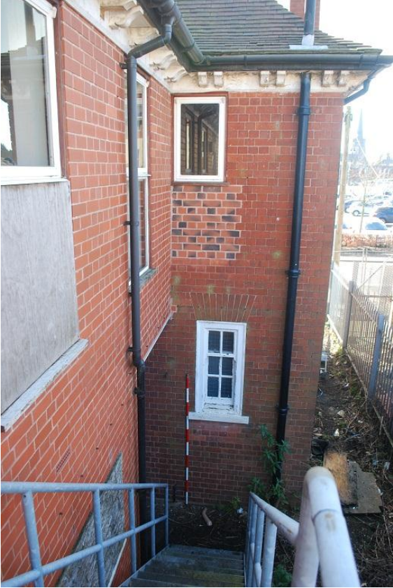
Plate 13 Exterior elevation of the drill sergeants' house, looking south west
