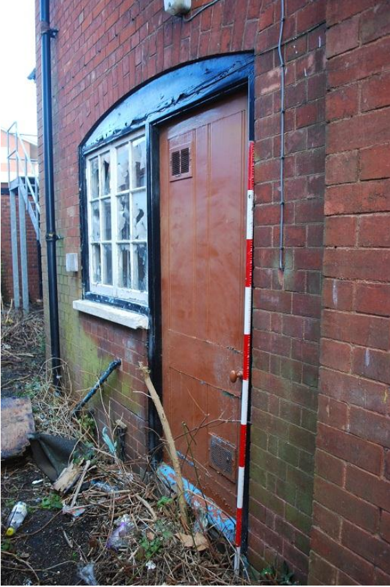
Plate 11 Exterior elevation of the drill sergeants' house, looking north east
