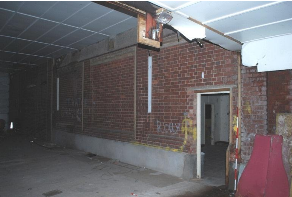
Plate 7 The gable end of the hall, looking south
