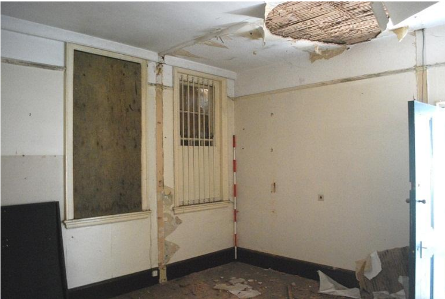
Plate 32 Interior of the social rooms, looking south
