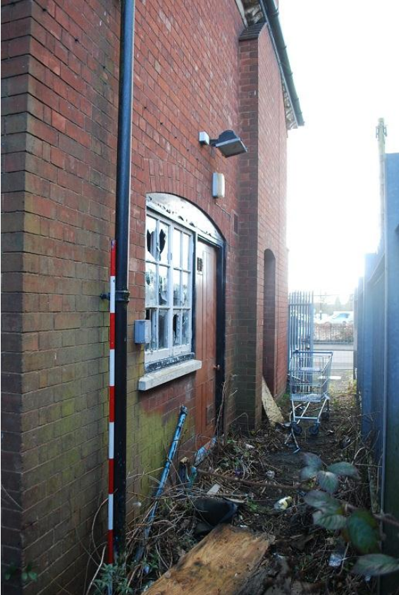
Plate 12 Exterior elevation of the drill sergeants' house, looking south west
