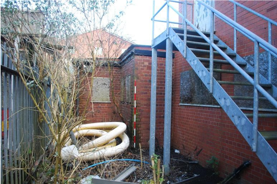
Plate 46 Exterior elevation of phase 2 structures, looking north east
