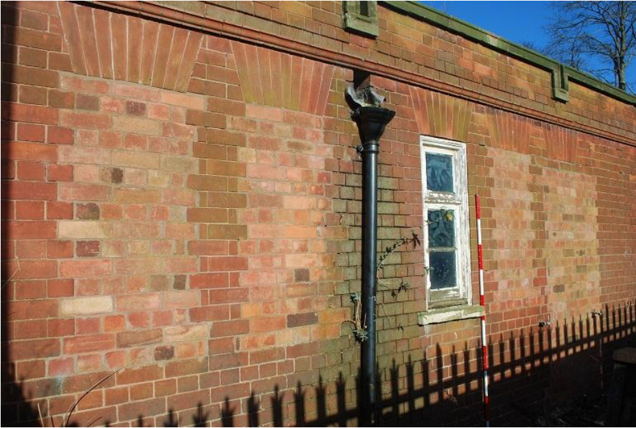
Plate 41 Exterior elevation of the toilet block and armoury, looking north
