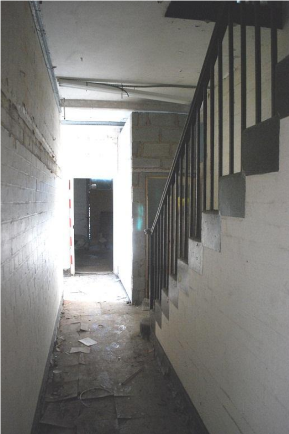
Plate 29 Interior passage of the social rooms, looking south west
