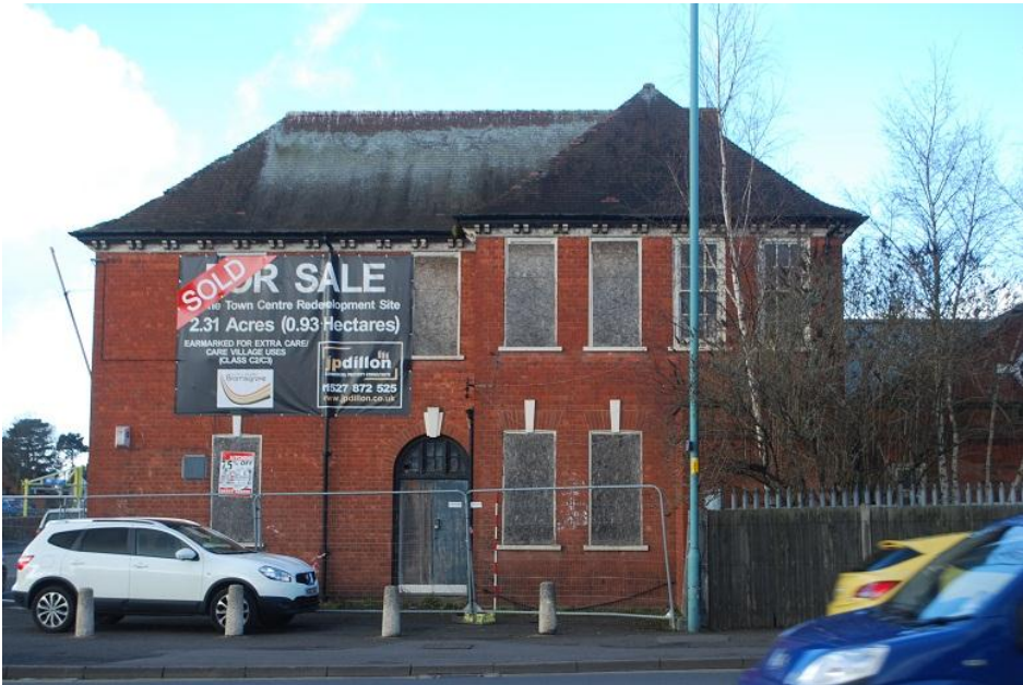
Plate 25 Exterior elevation of the social rooms, looking north west
