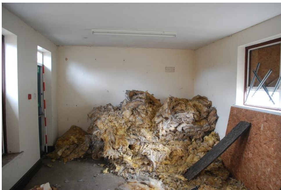
Plate 58 Interior of phase 3 structure, looking north east
