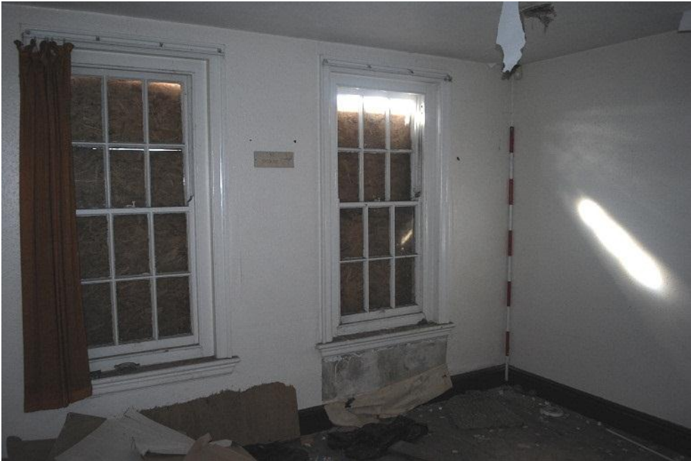
Plate 21 Bedroom of the drill sergeants' house, looking west
