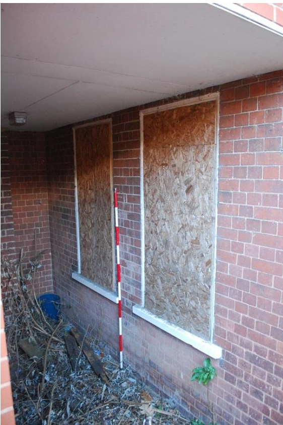
Plate 14 Exterior elevation of the drill sergeants' house, looking south east
