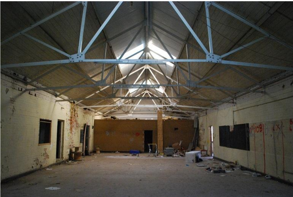
Plate 4 The hall, looking north east
