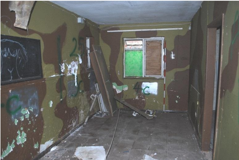
Plate 49 Interior of phase 2 structures, looking north west
