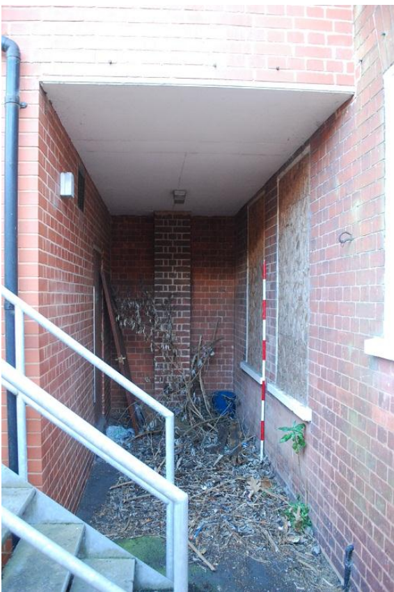
Plate 56 Exterior elevation of phase 3 structure, looking south east
