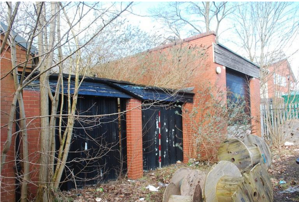
Plate 54 Exterior of phase 3 rifle range and garage, looking north west
