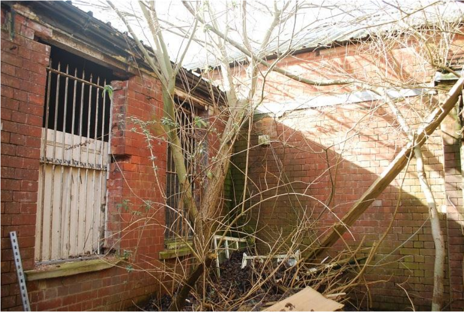
Plate 43 Exterior elevation of the armoury, looking south west
