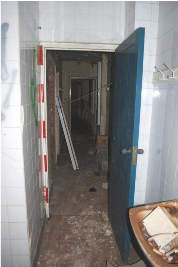
Plate 47 Interior of phase 2 structures, looking north east
