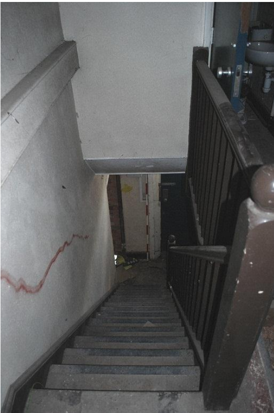
Plate 24 Stairs in the drill sergeants' house, looking south west
