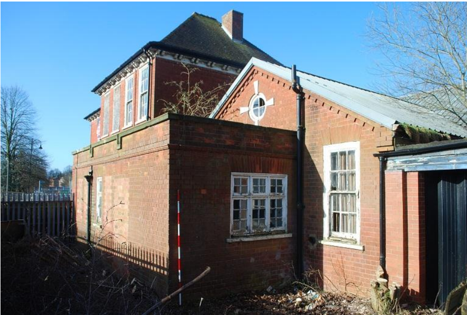
Plate 40 Exterior elevation of the toilet block and armoury, looking south west
