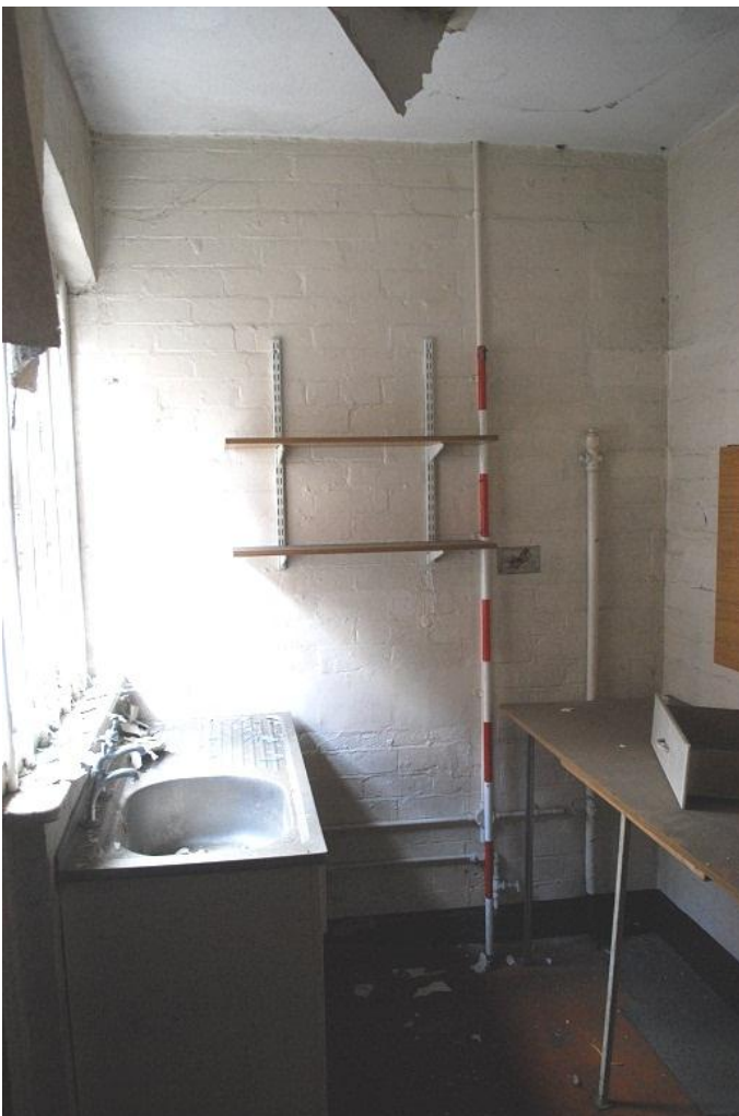
Plate 18 Kitchen of the drill sergeants' house, looking north east
