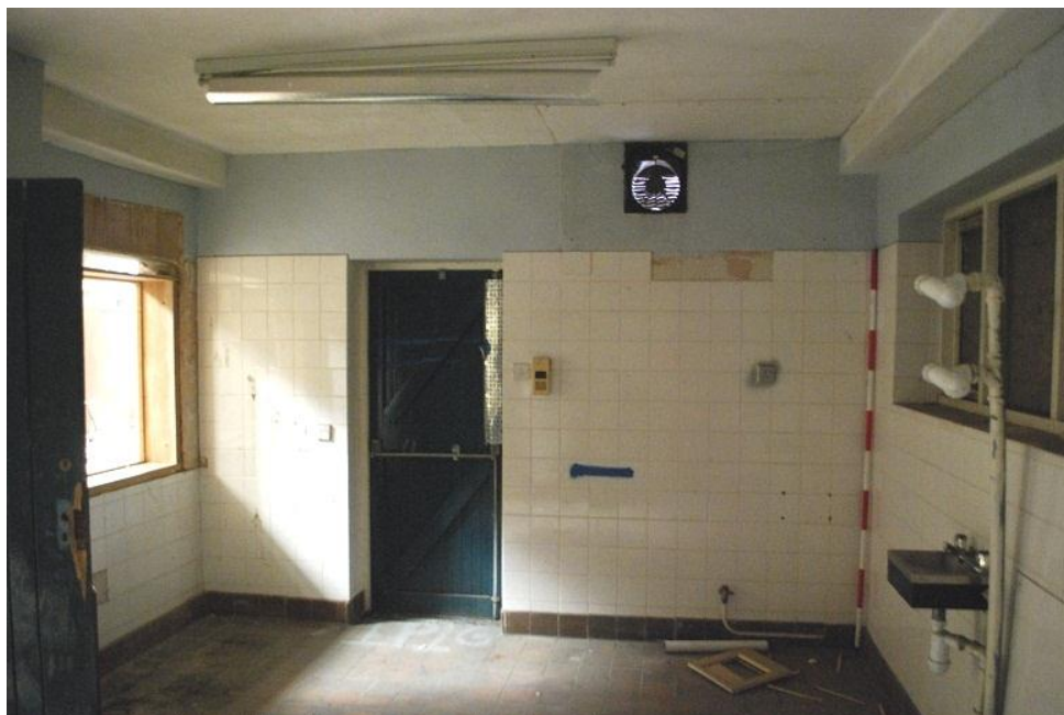
Plate 57 Interior of phase 3 structure, looking south west
