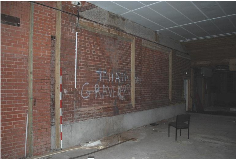
Plate 6 The gable end of the hall, looking west
