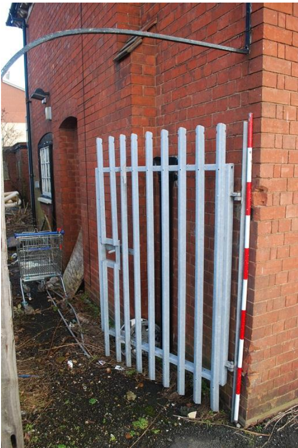
Plate 10 Exterior elevation of the drill sergeants' house, looking north east
