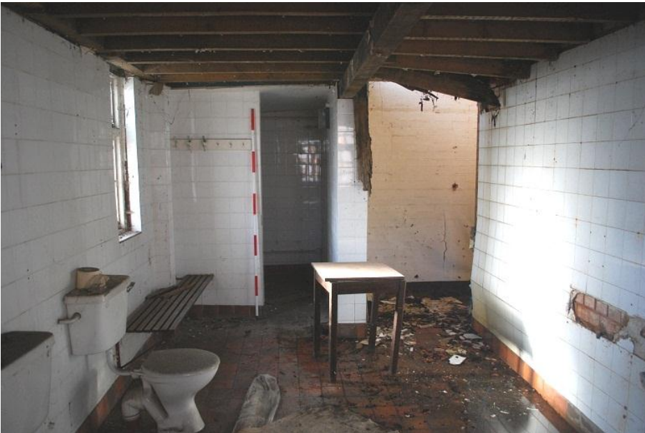
Plate 42 Interior of the toilet block and armoury, looking south west
