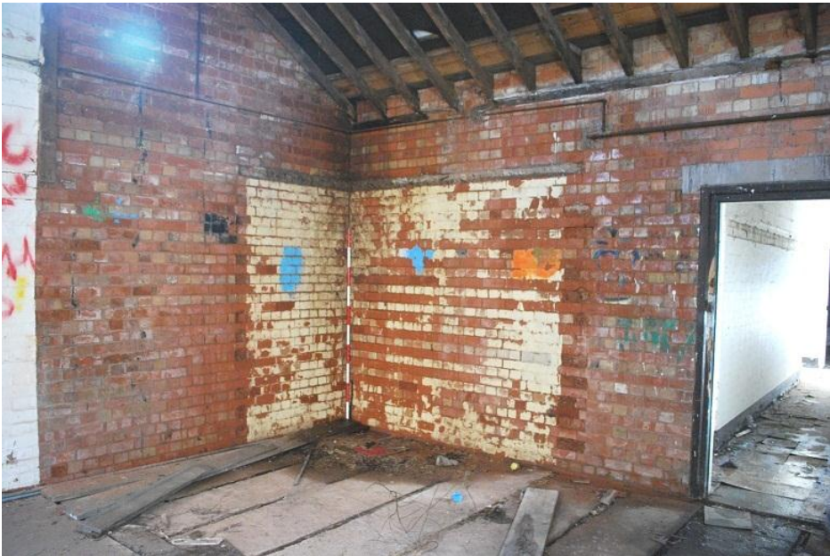
Plate 45 Interior of the armoury, looking south east
