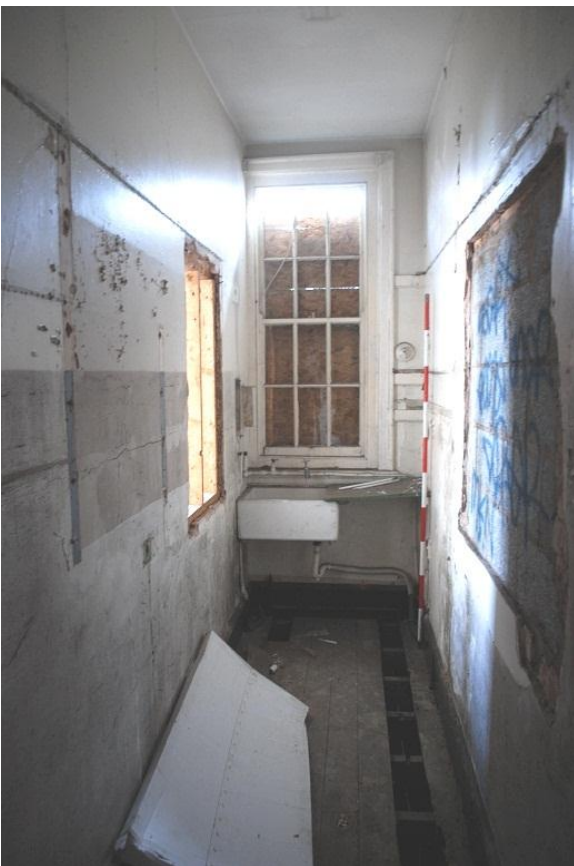
Plate 36 First floor of the social rooms, looking south east
