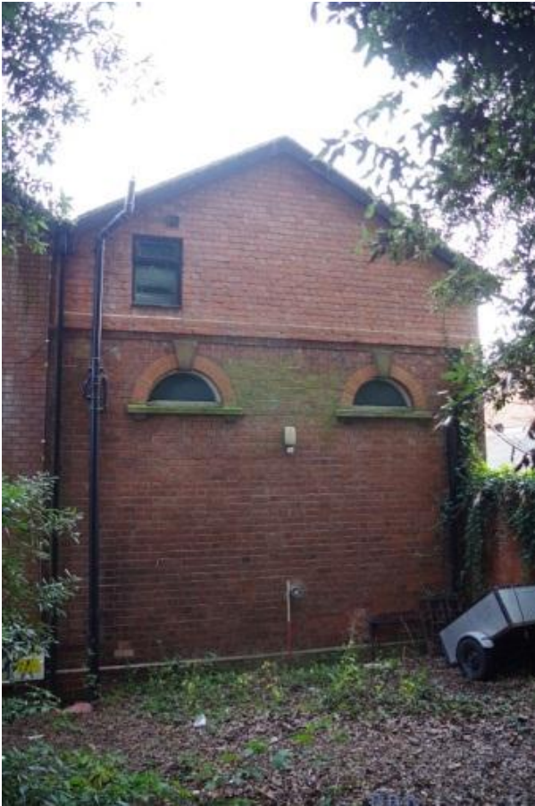
Plate 58 Western gable of the coach house, looking east
