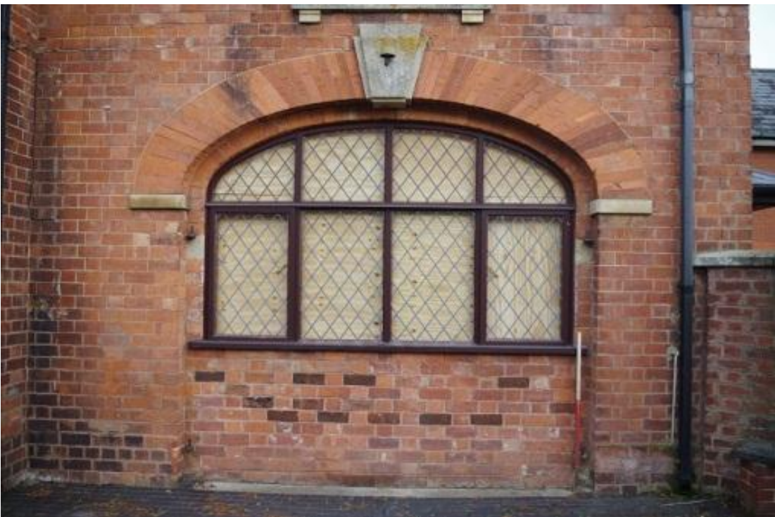
Plate 56 Former coach entrance, looking north west
