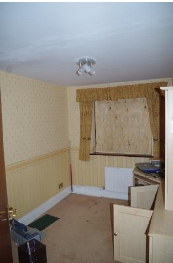
Plate 82 Late 20th century extension to the coach house ground floor, looking north west
