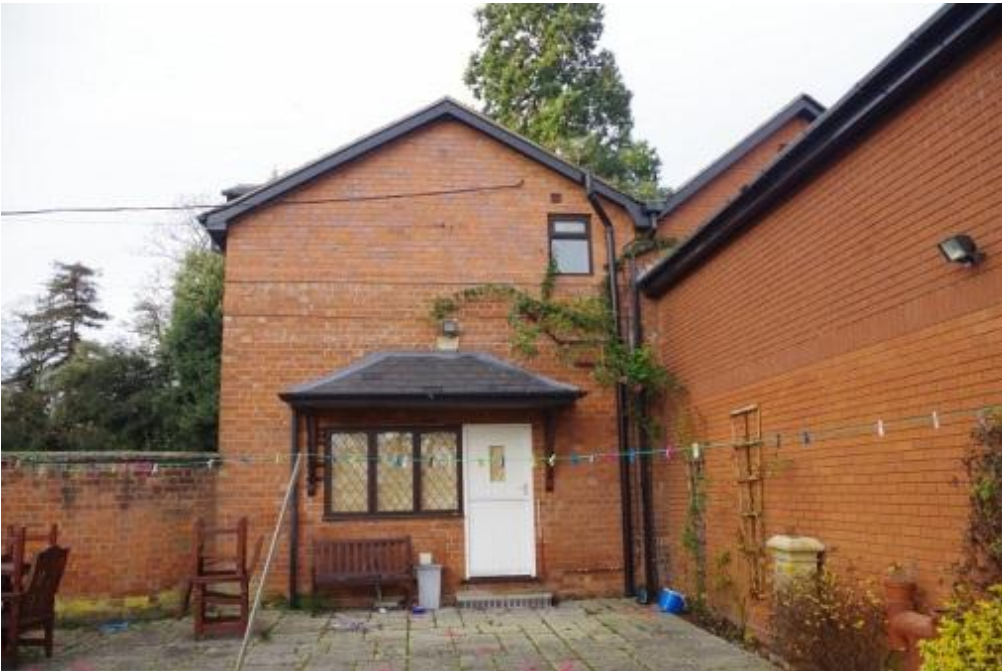
Plate 63 Eastern gable of coach house, looking west
