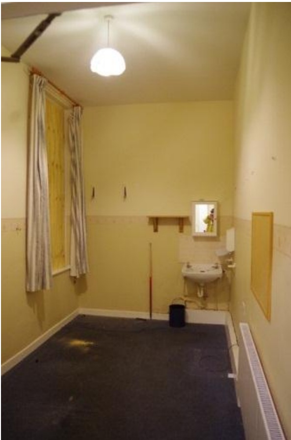
Plate 68 20 th century extension ground floor, looking north east
