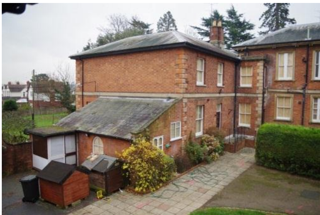
Plate 41 The service wing, looking south west
