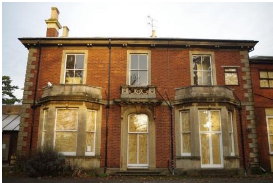
Plate 6 South east facing Italianate elevation of the house, looking north west
