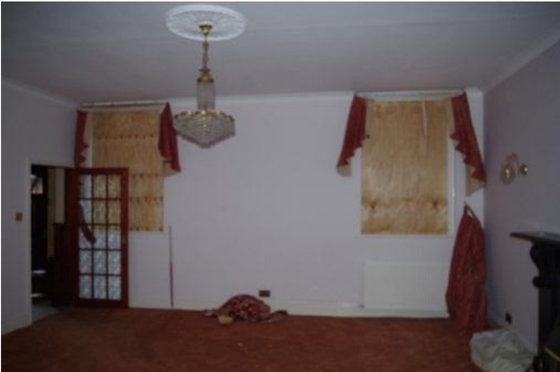
Plate 57 Western ground floor room of the coach house, looking south east
