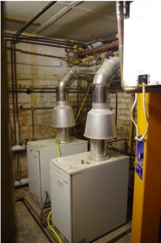
Plate 32 Former storage room, looking south west
