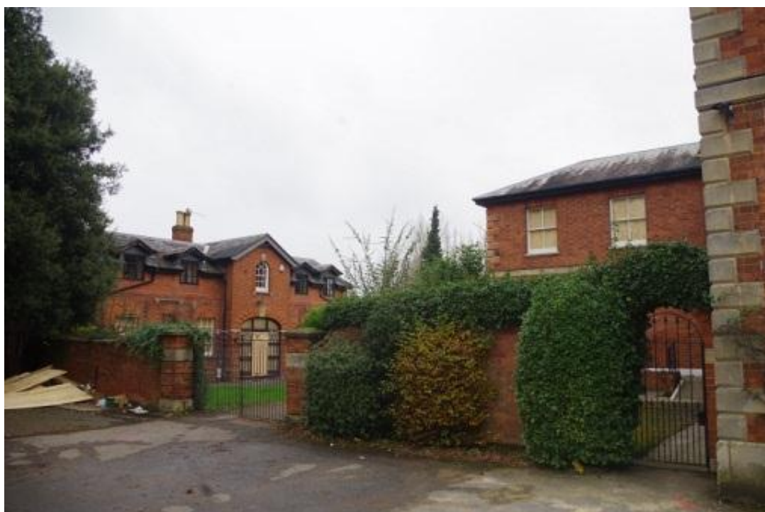
Plate 53 The yard area, looking north east
