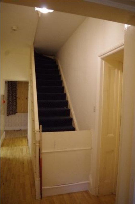
Plate 51 Service wing stairs, looking north east
