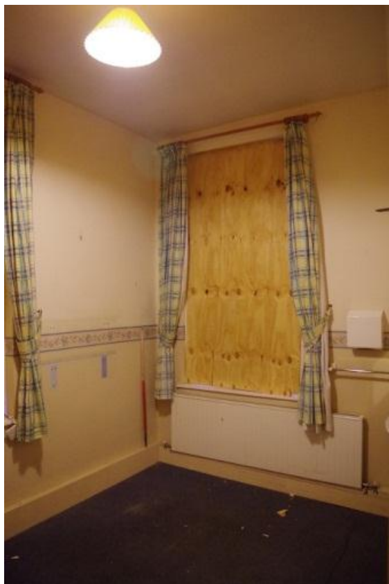
Plate 69 20th century extension ground floor, looking south east
