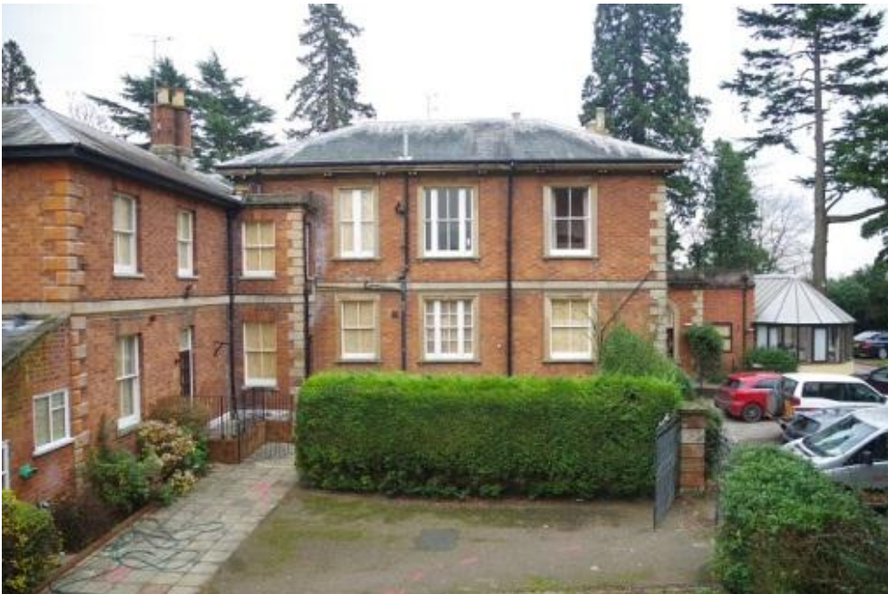
Plate 4 View of the house looking south west with the service wing to its left
