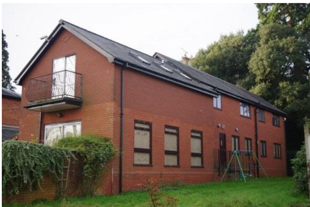
Plate 77 Late 20th century extension to the coach house, looking south west
