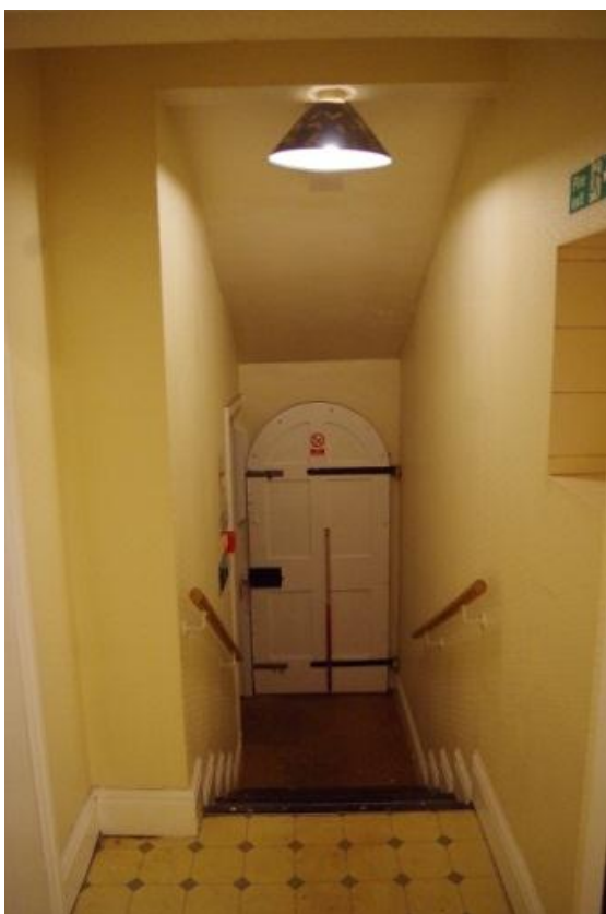
Plate 50 Single storey element of the service wing, looking north west
