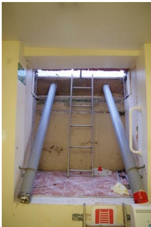
Plate 29 Former coal shoot in the cellar, looking north west
