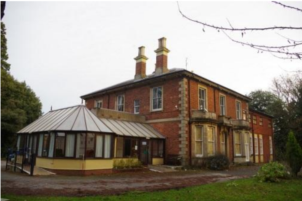
Plate 2 View of the house looking north east
