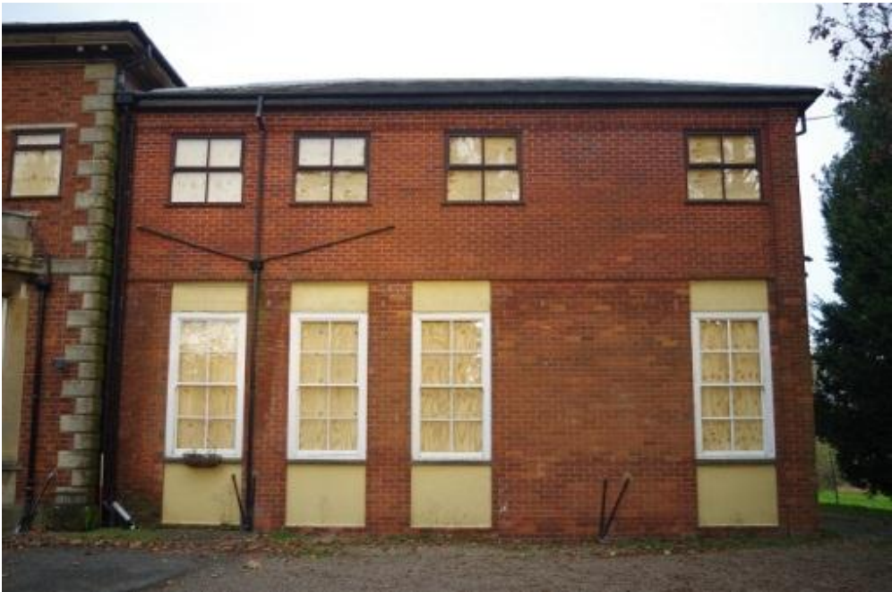
Plate 65 Mid 20 th extension, looking north west
