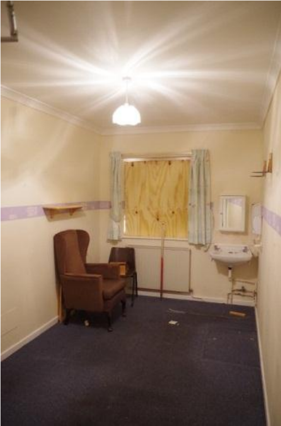
Plate 71 20th century extension first floor, looking south east
