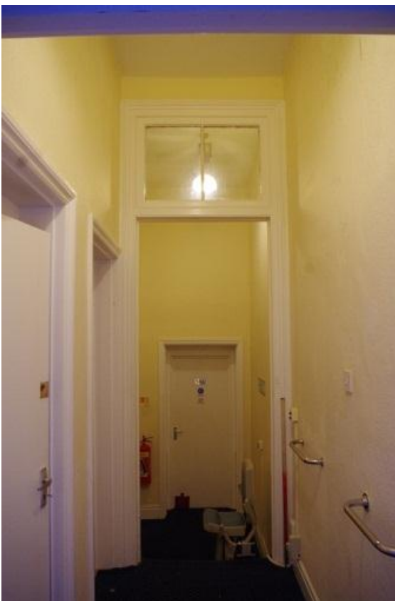
Plate 40 Passage into the first floor service wing
