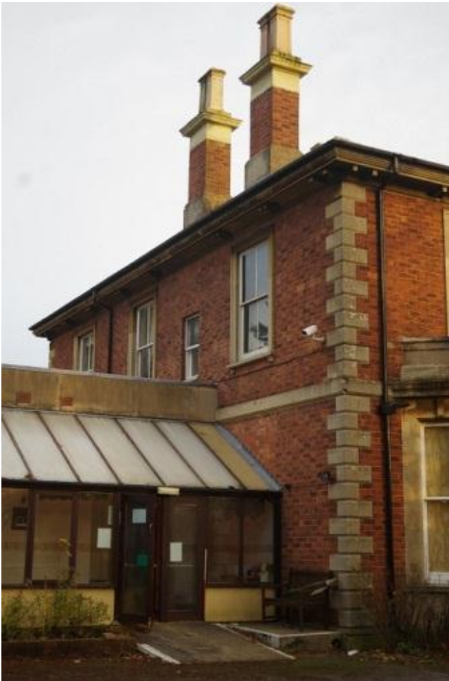
Plate 3 View of the house looking north east
