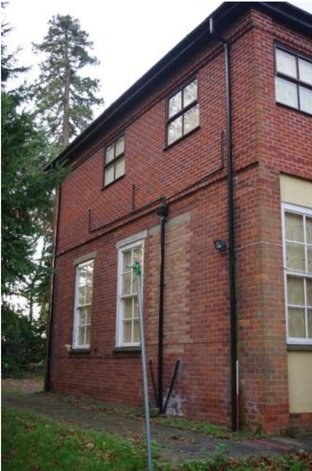
Plate 66 Mid 20 th extension, looking south east
