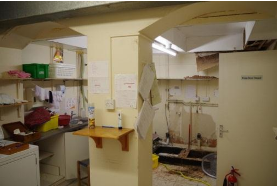
Plate 28 Former coal cellar, looking north east
