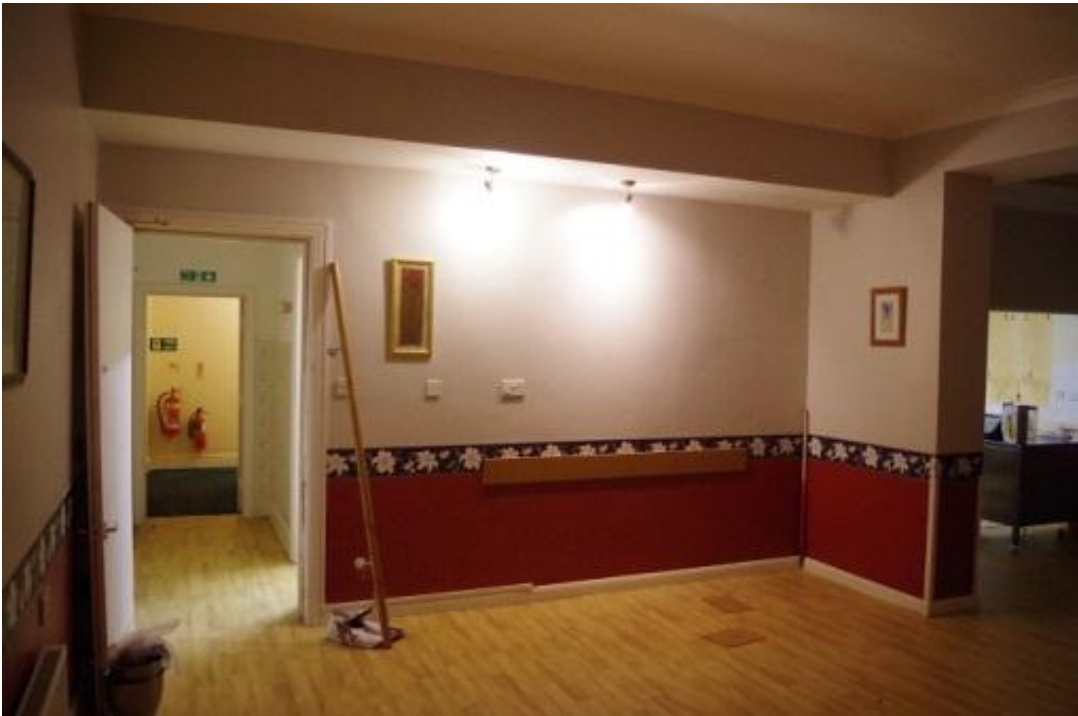
Plate 45 Former kitchen, looking north
