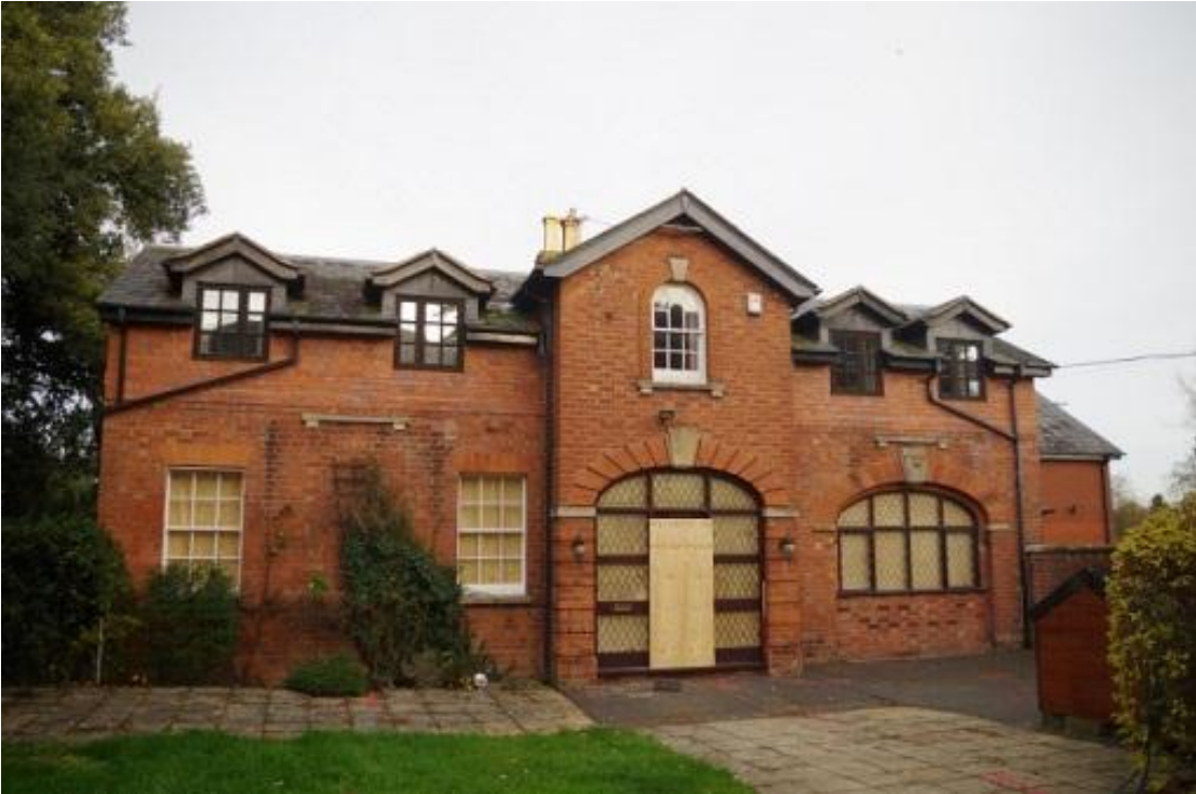
Plate 55 Former coach house, looking north
