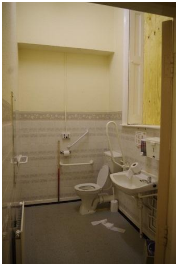
Plate 25 Former ground floor service room, looking west
