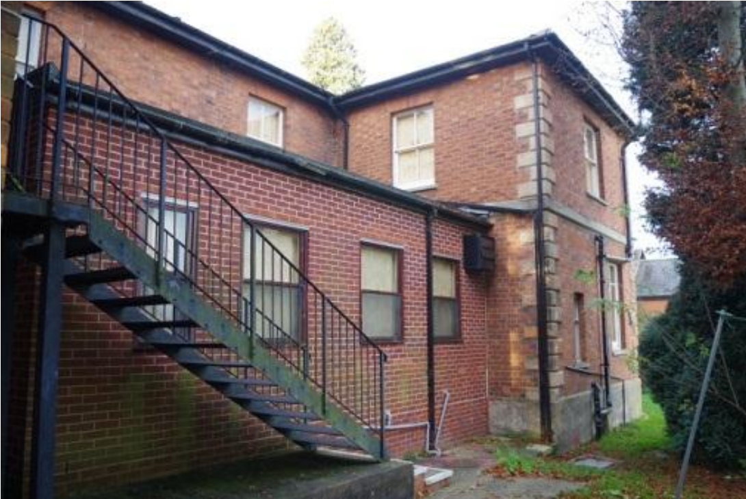
Plate 43 Service wing with 20 th century addition, looking north west
