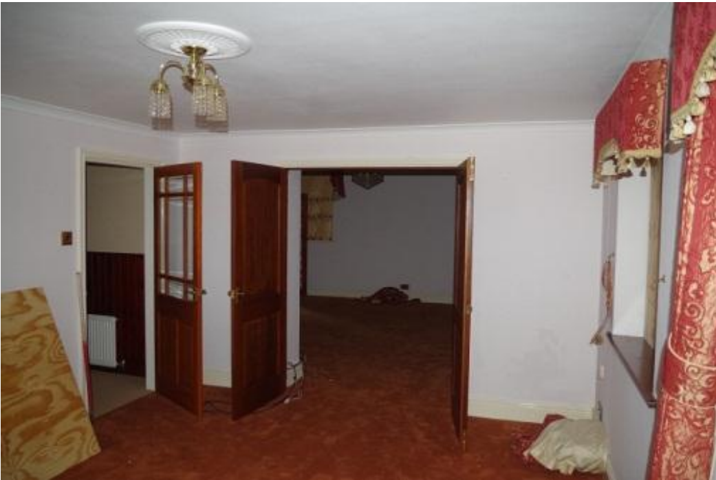
Plate 79 Late 20th century extension to the coach house ground floor, looking south east
