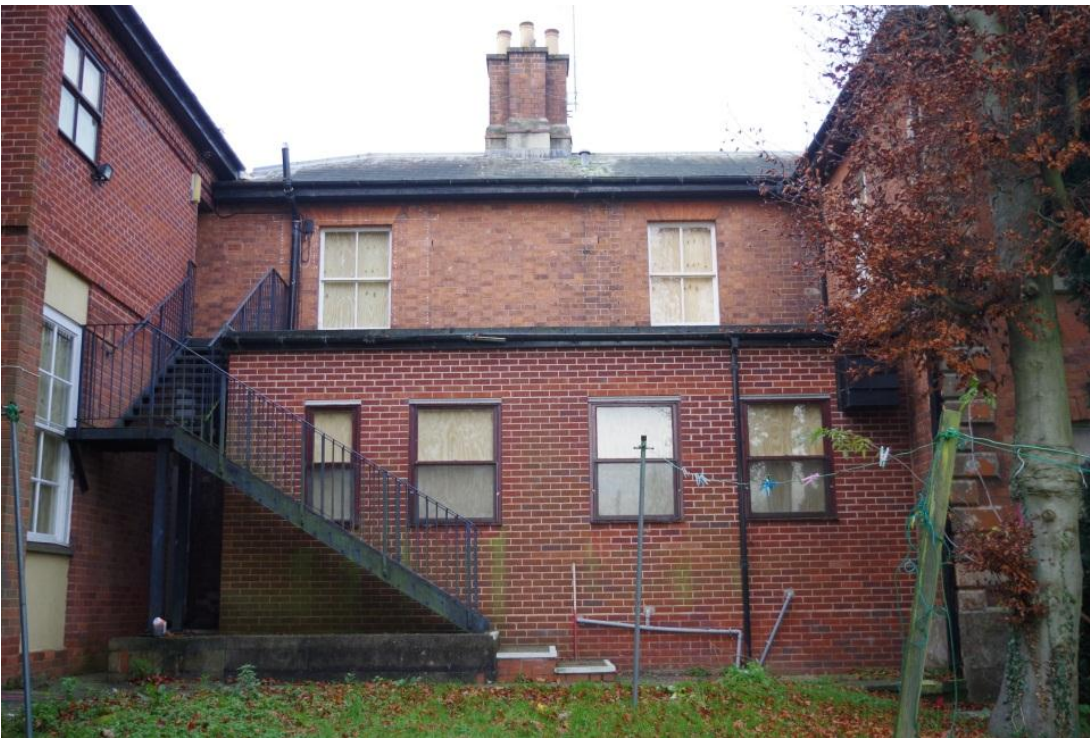
Plate 44 Service wing with 20 th century addition, looking west
