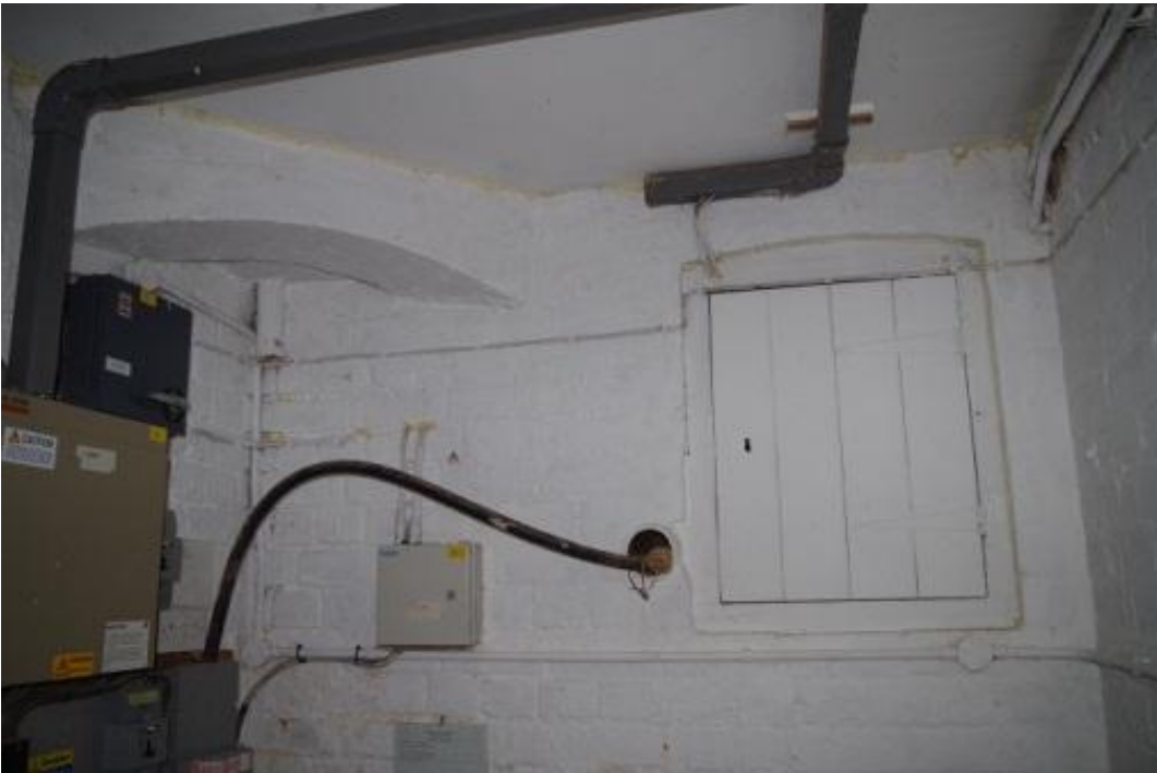
Plate 35 Possible flue in cellar, looking south east
