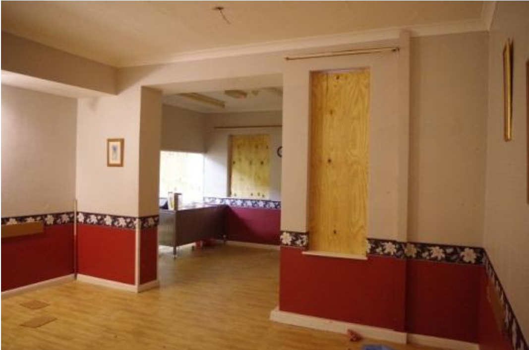
Plate 46 Former kitchen looking north west
