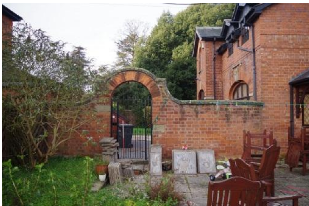
Plate 54 Pedestrian access to the yard, looking south west
