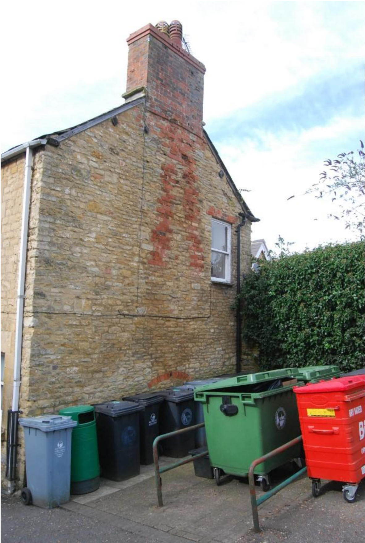
Plate 11 Gable end of No 7 High Street, looking northwest
