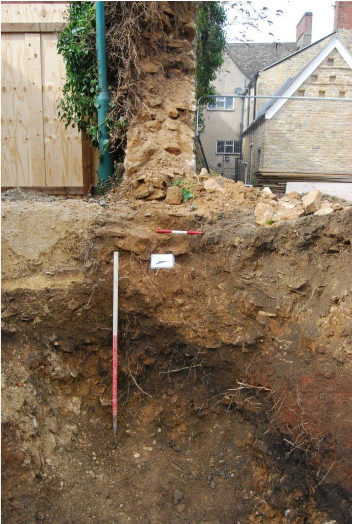
Plate 6 Boundary wall between 7 and 8 High Street
