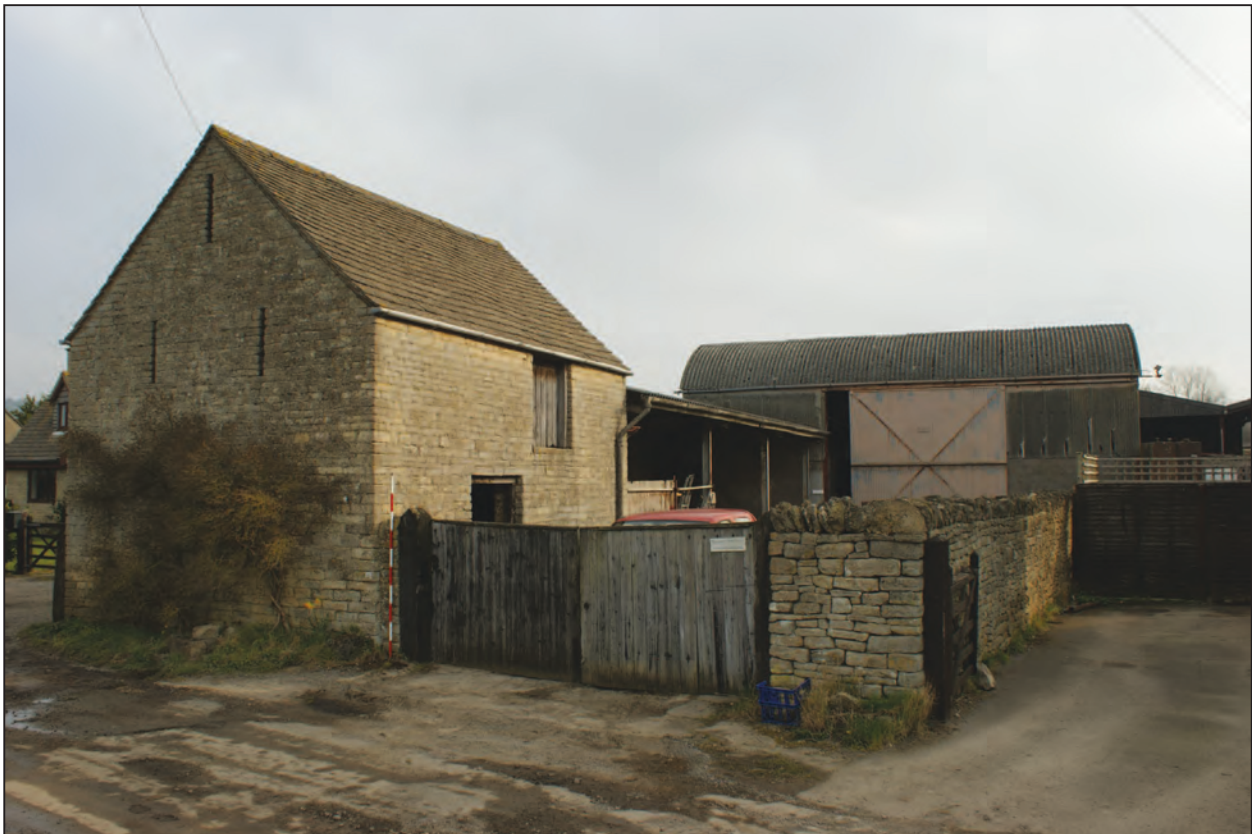
Stable facing north-east
