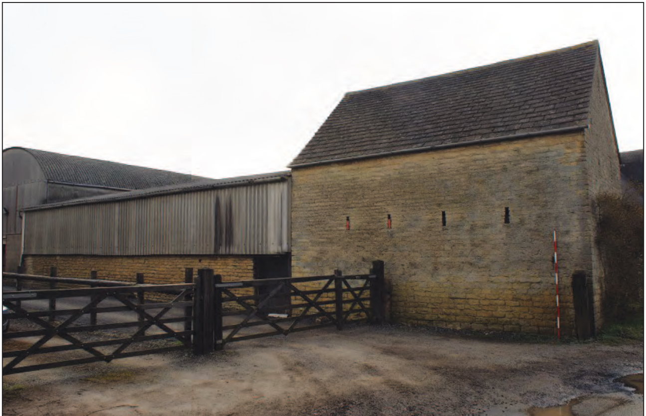
Stable and shelter shed facing south-east
