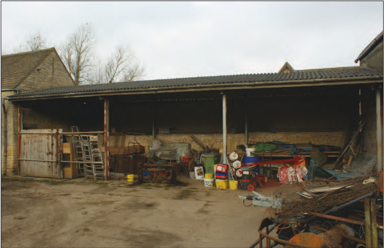
Shelter shed facing north-west
