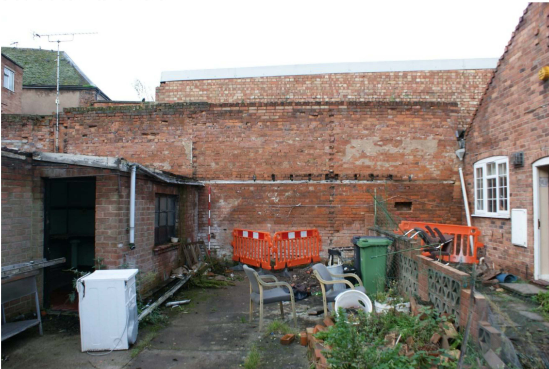
Plate 22: The wall to the south of the bungalow showing evidence of a former terrace.
