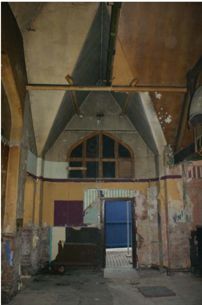
Plate 12: Later doorway inserted through a former window.
