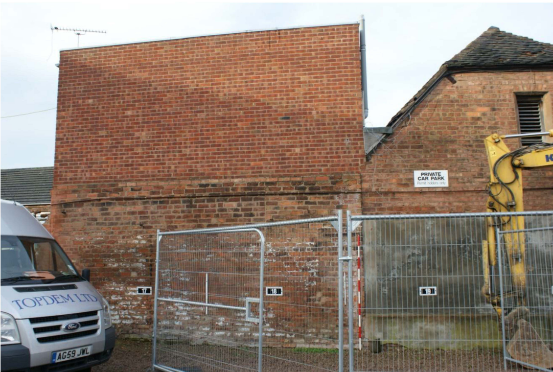
Plate 24: Exterior of the building containing the skittle alley.
