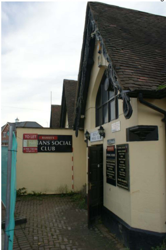
Plate 8: The entrance to the former social club, inserted through the position of a former window.
