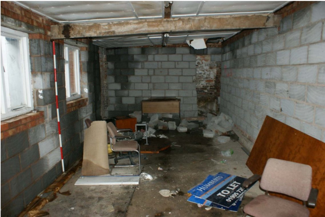
Plate 29: Interior of the building at the southern end of the plot.
