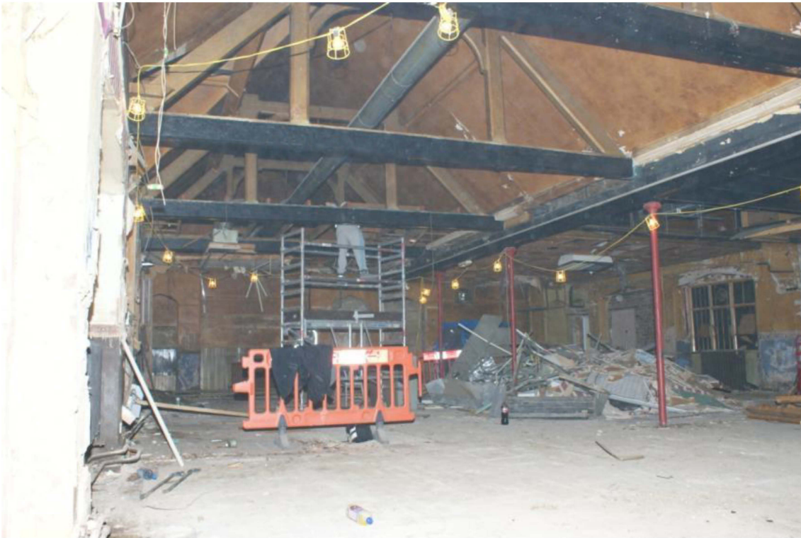
Plate 11: Interior of the former school building after the removal of a later ceiling relating to its use as a social club.
