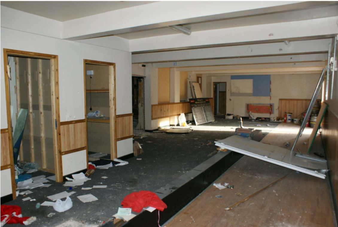
Plate 25: Ground floor interior showing the skittle alley.
