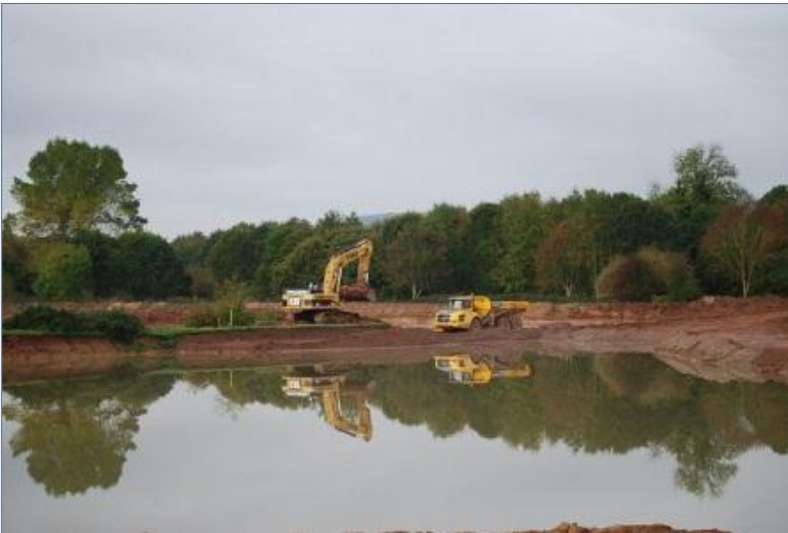
Plate 12: Excavations in progress along the hedgerow dividing Phase 1A and 1B
