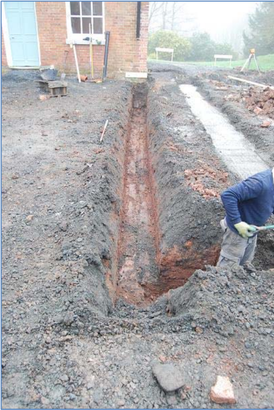
Plate 10 Location of South-west single storey extension foundation trench
