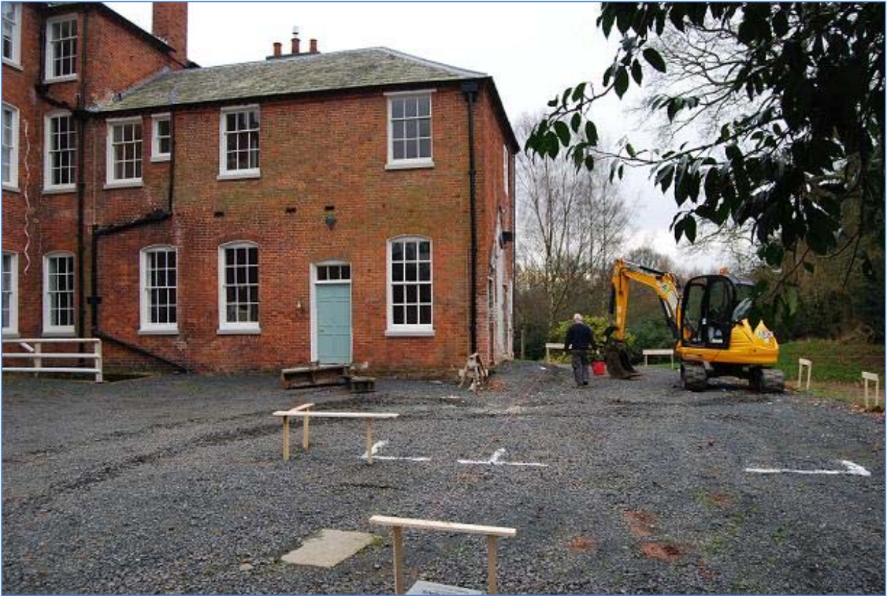
Plate 8 Location of South-west single storey extension
