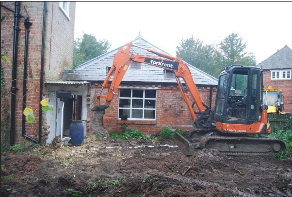
Plate 5 Location of Trench 2 before excavation
