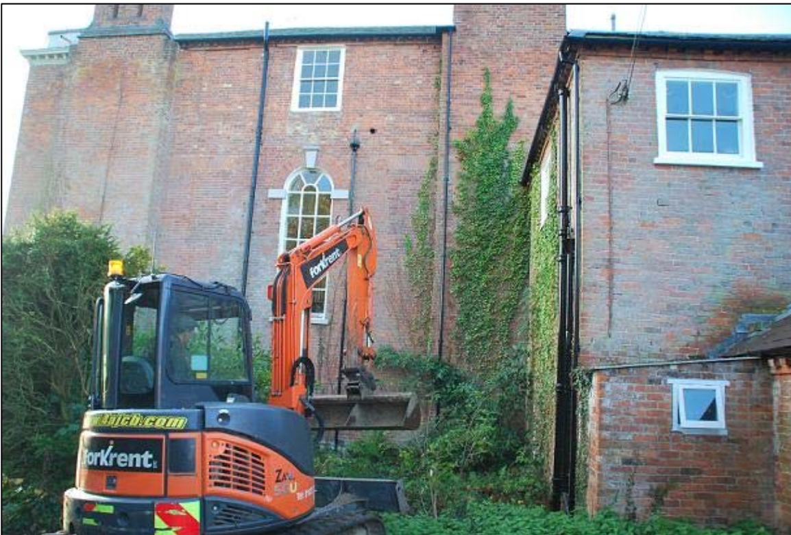
Plate 2 Location of trench 1
