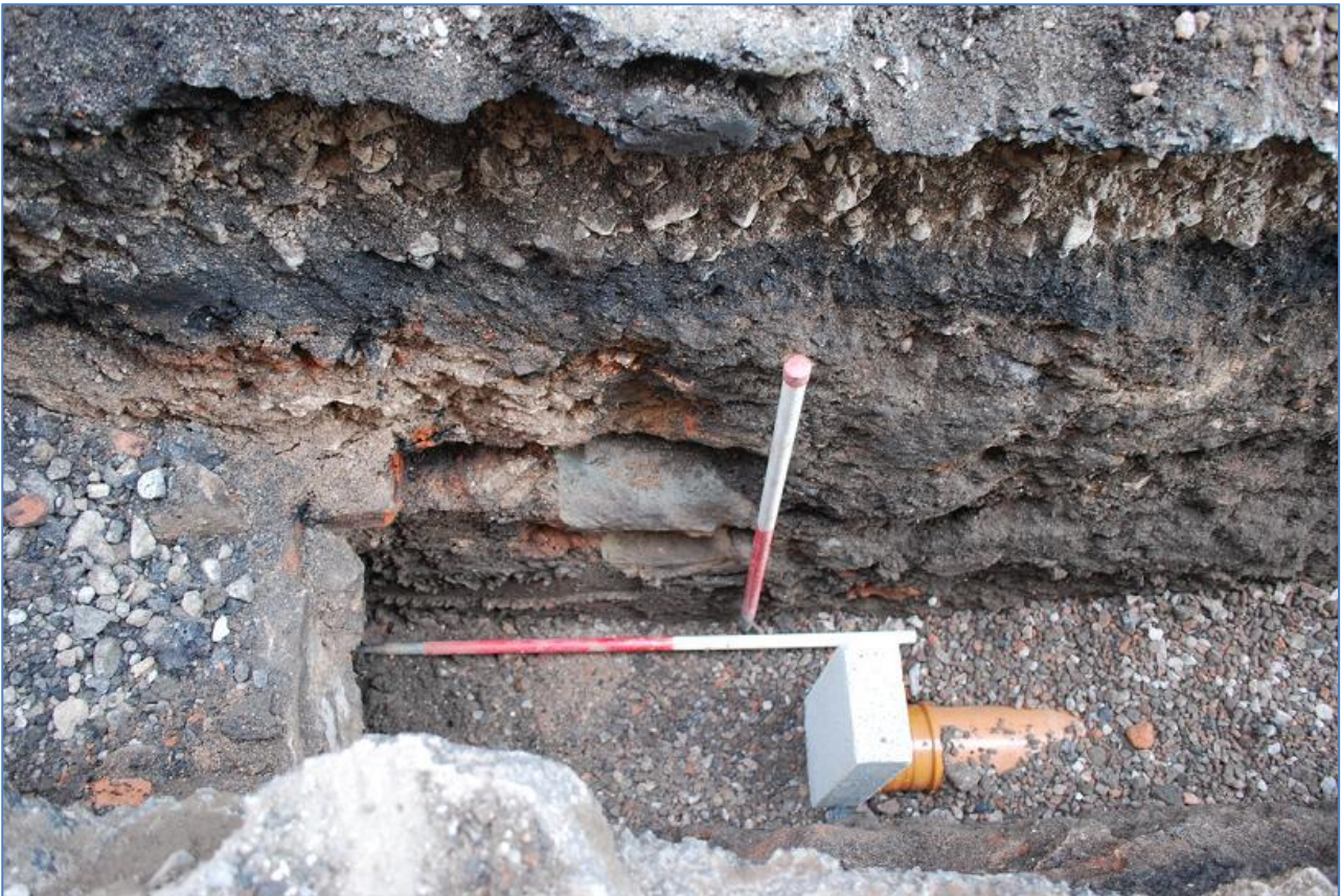
Plate 6 Ashlar masonry from city wall; reused in modern concrete foundations.
