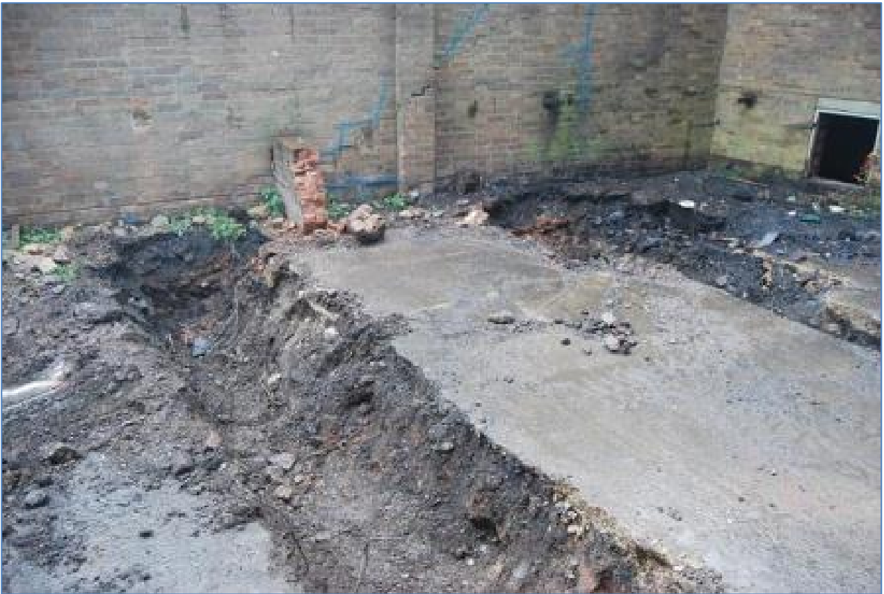
Plate 3 Trenches 3 and 4, entrance foundations on west side of building, view north-west.
