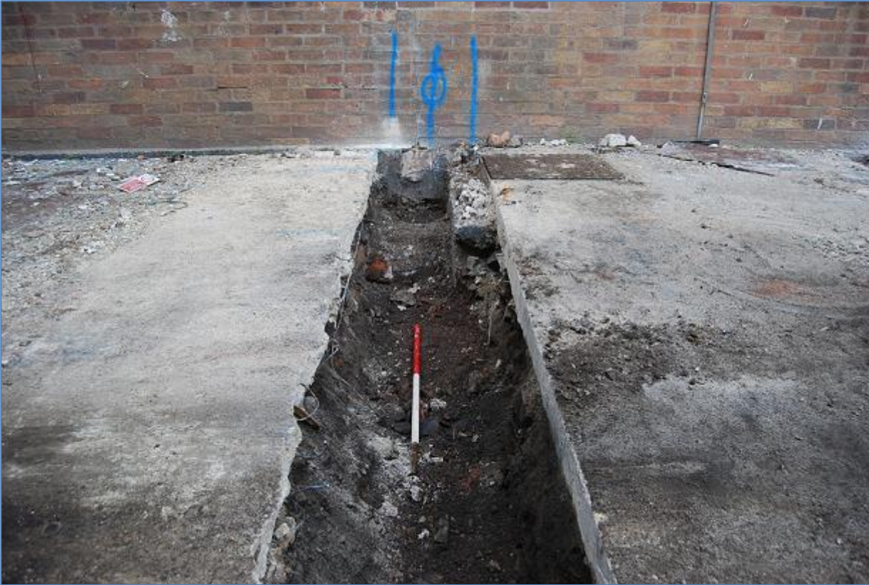
Plate 1 Trench 3 entrance foundations, view east.
