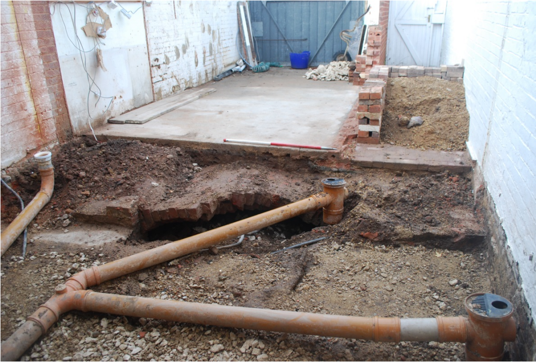
Plate 1 The brick vaulted cellar looking west (1m scale)
