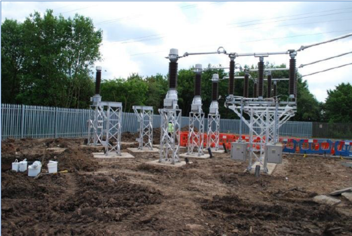
Plate 1 The location of trench between the new substation structures; facing south-east
