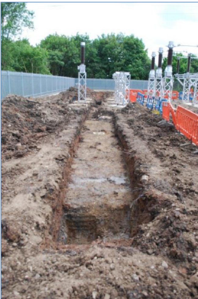
Plate 8 General shot of trench; facing south
