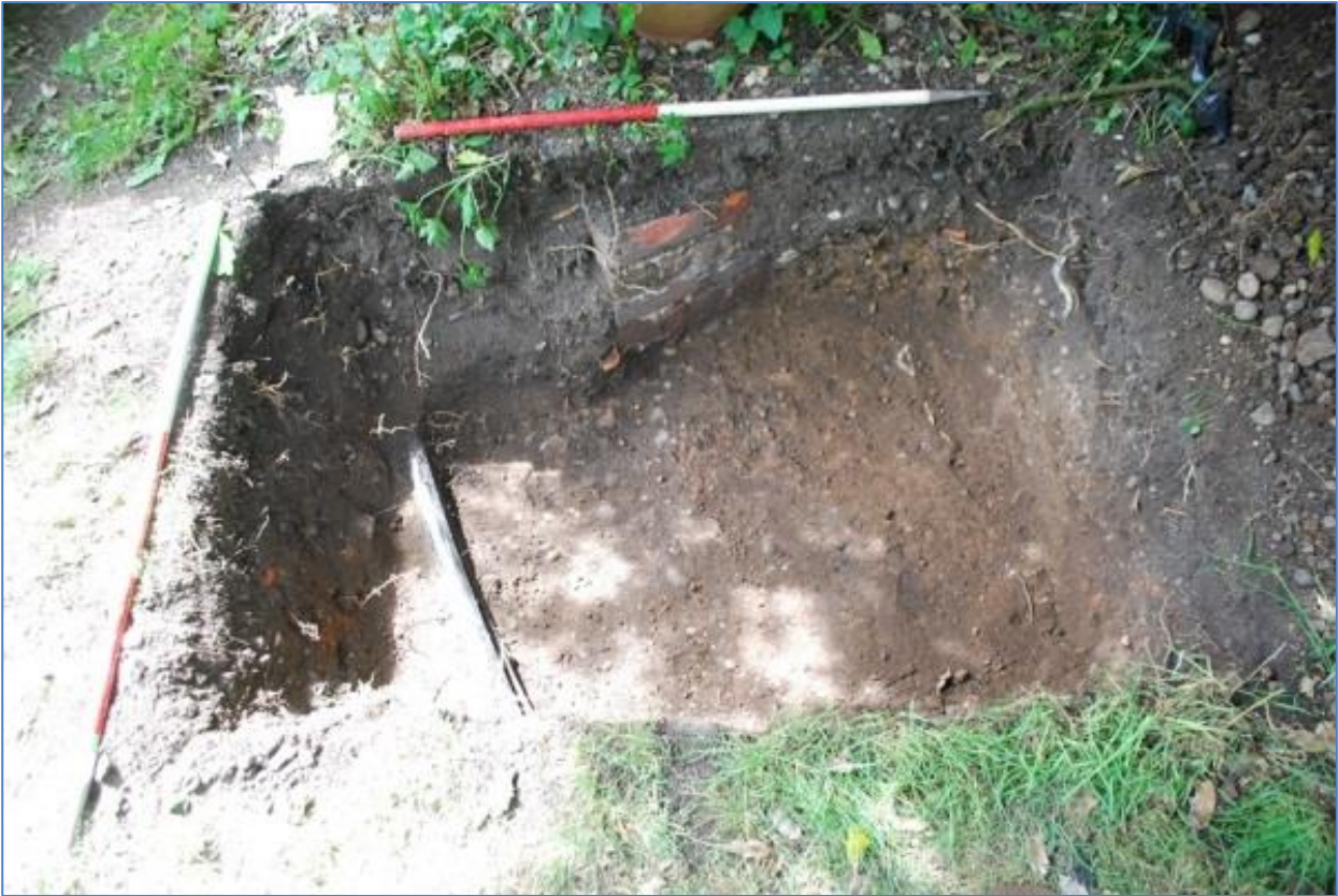
Plate 3 Trench 4 at full depth showing the electric cable and brick manhole; view west
