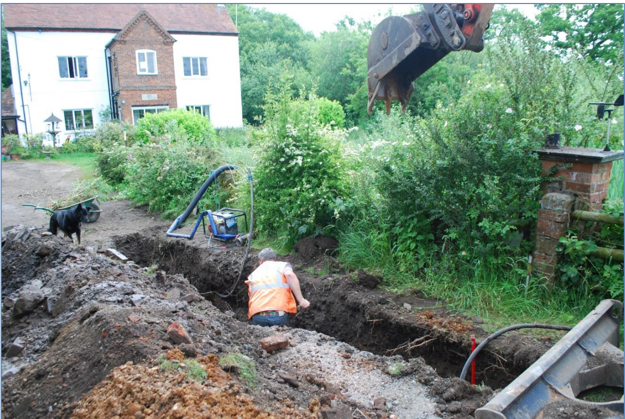
Plate 8 The location of Trench 7 during works; view east
