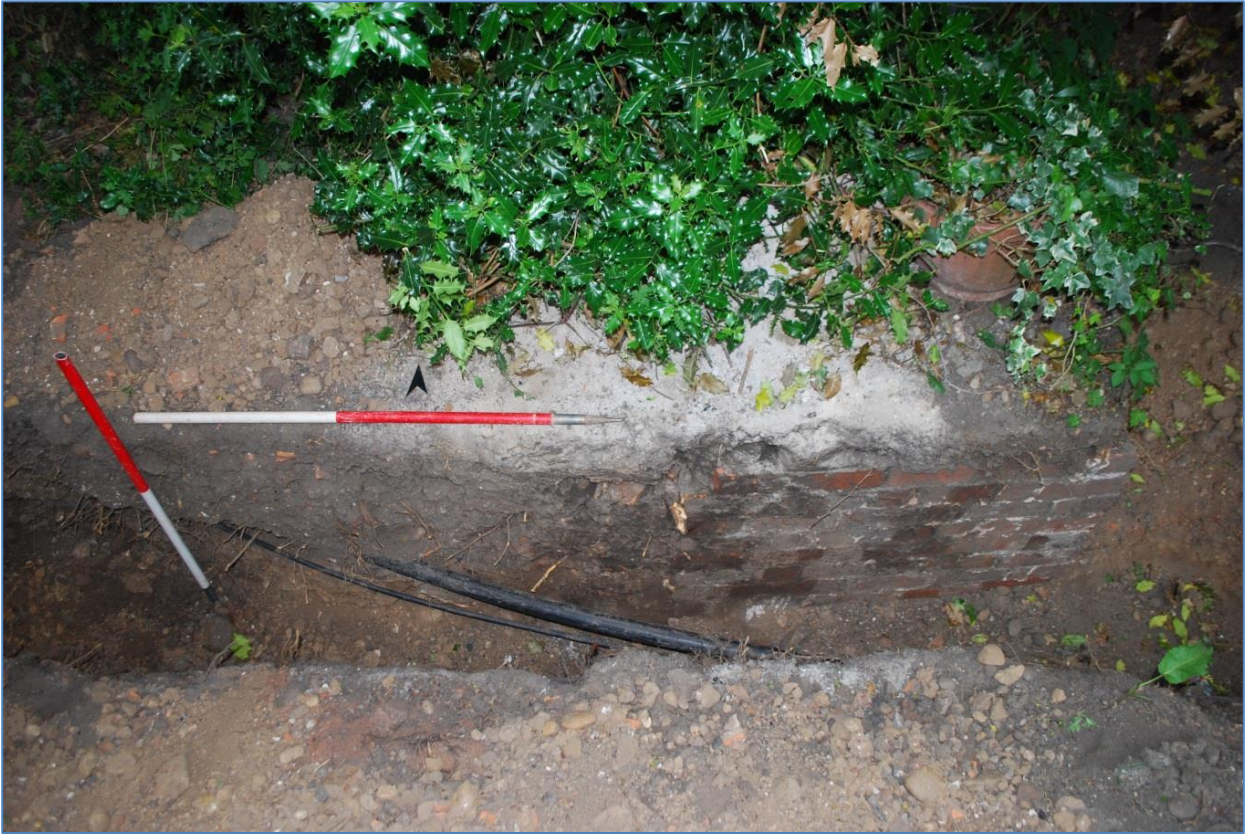
Plate 9 Sample section of Trench 8 showing modern manhole uncovered in Trench 4
