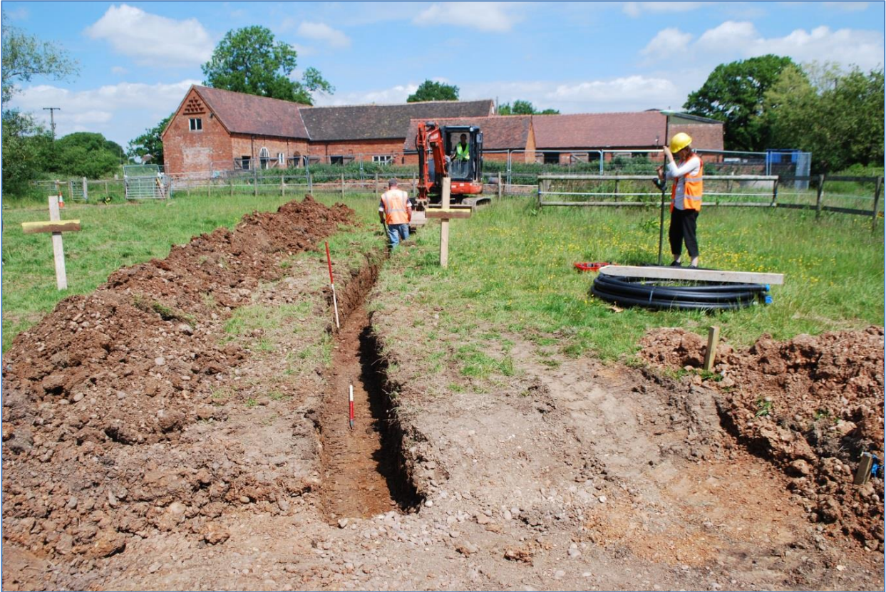
Plate 5 Trench 6 during works; view north-west
