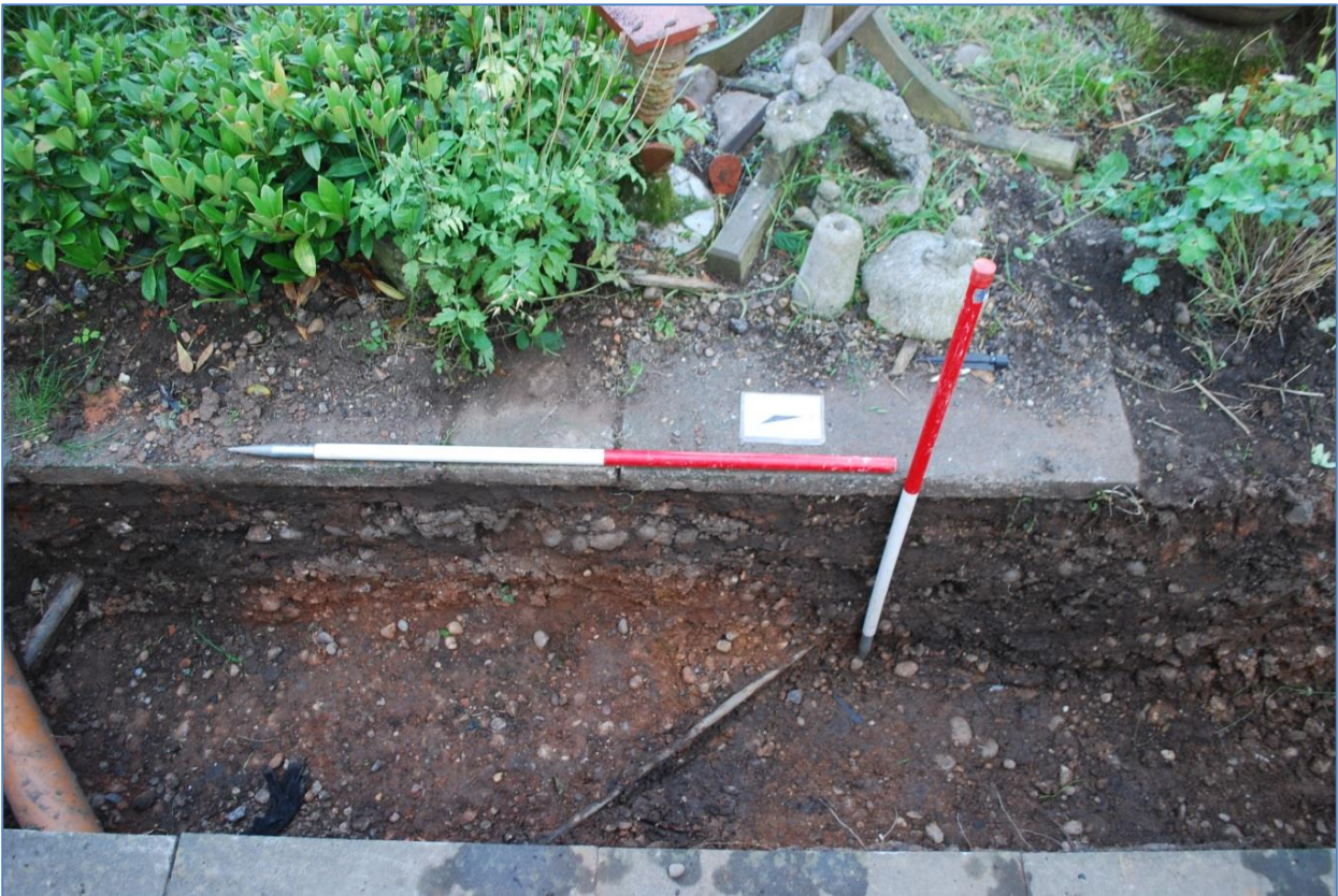
Plate 11 Trench 9 sample section showing services running into the house
