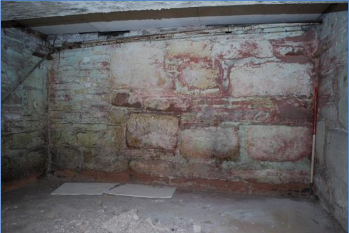
Plate 7 The north-eastern wall of cellar constructed of sandstone blocks.
