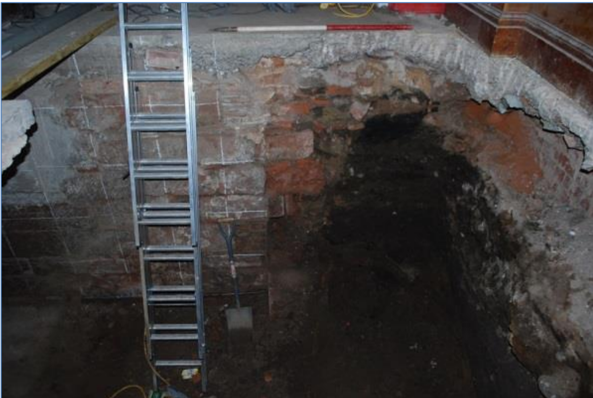
Plate 4 The western wall after full excavation, down to the base. Showing the dark backfill (112) of the wall cut and existing building foundations.
