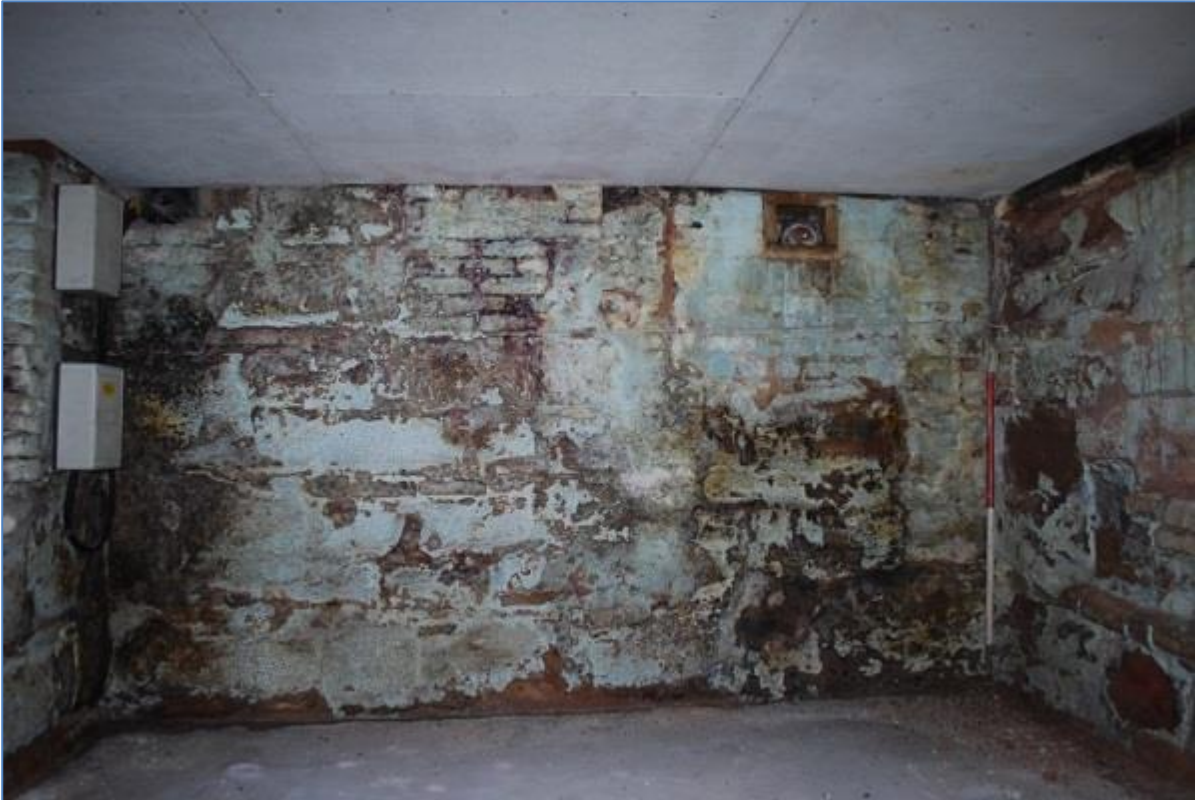
Plate 9 The southeastern wall of the cellar.
