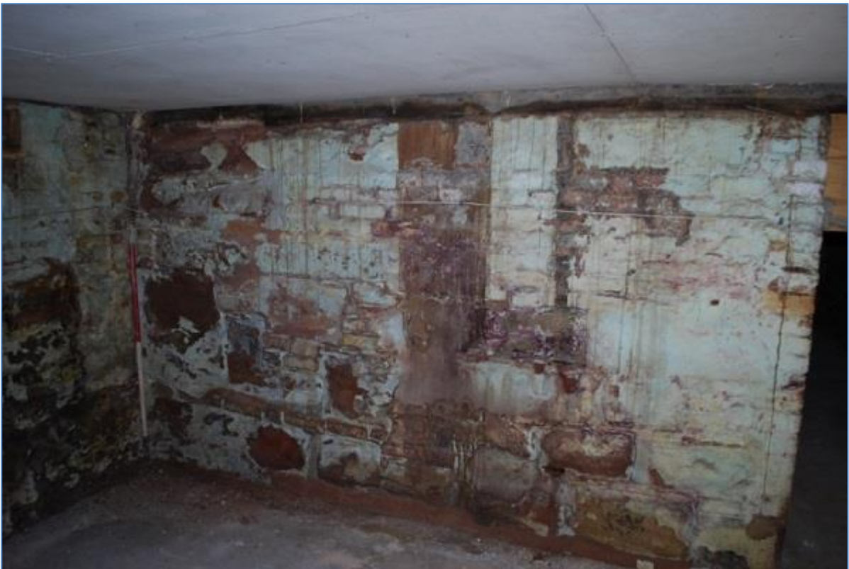
Plate 8 Wall of eastern room of cellar, view southwest.
