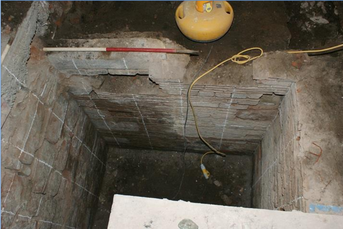
Plate 3 The cellar walls uncovered by the lift shaft works. View north.
