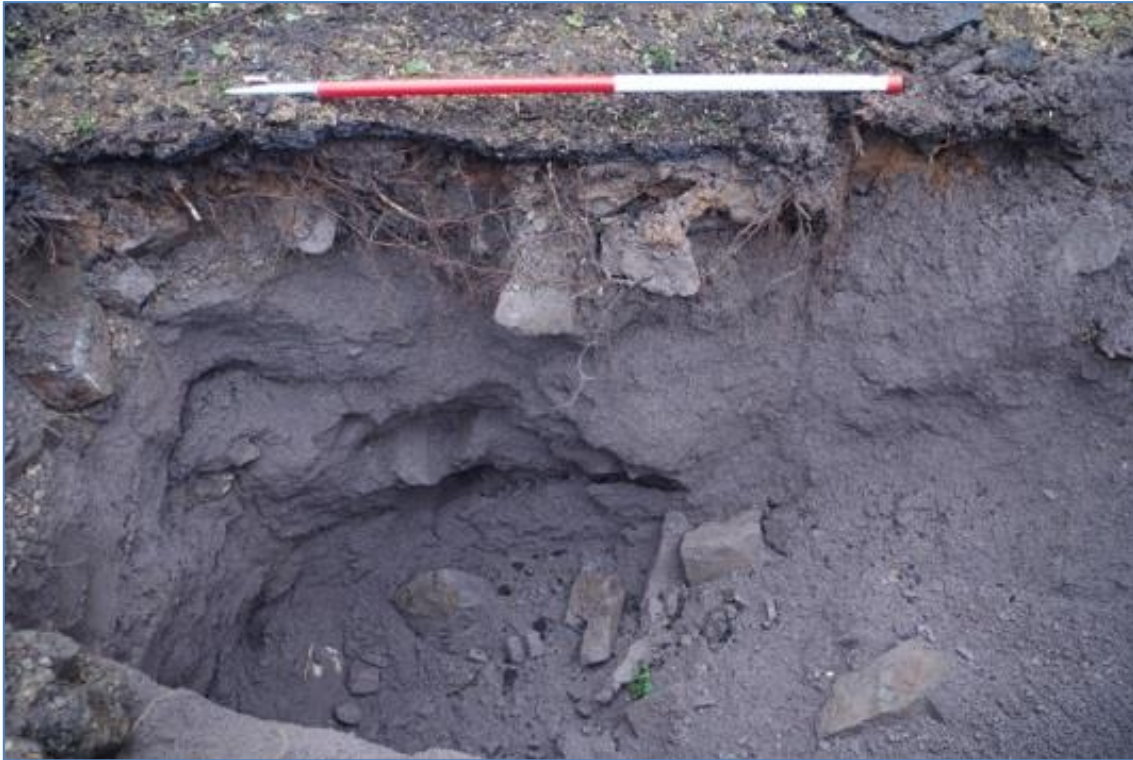
Plate 7 Geotechnical pit 15 showing unstable made ground
