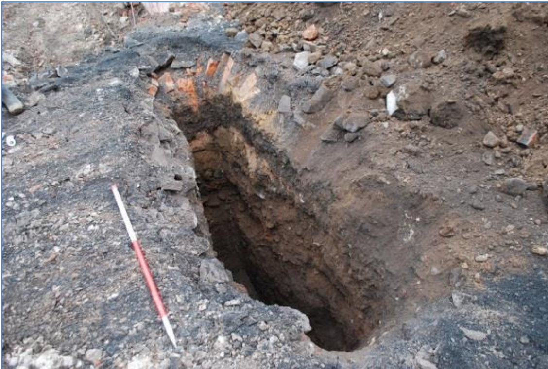
Plate 8 Geotechnical pit 16 (TP101) showing made ground
