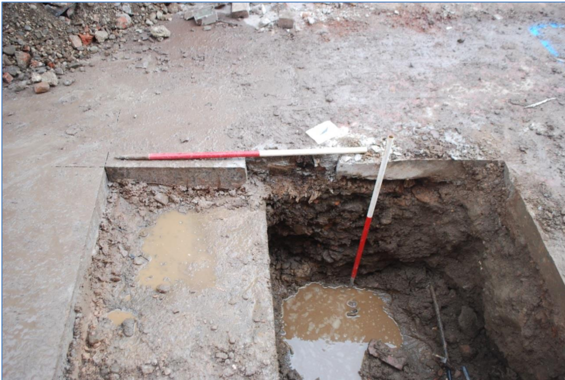
Plate 12 Trench 21 showing made ground and ring beams
