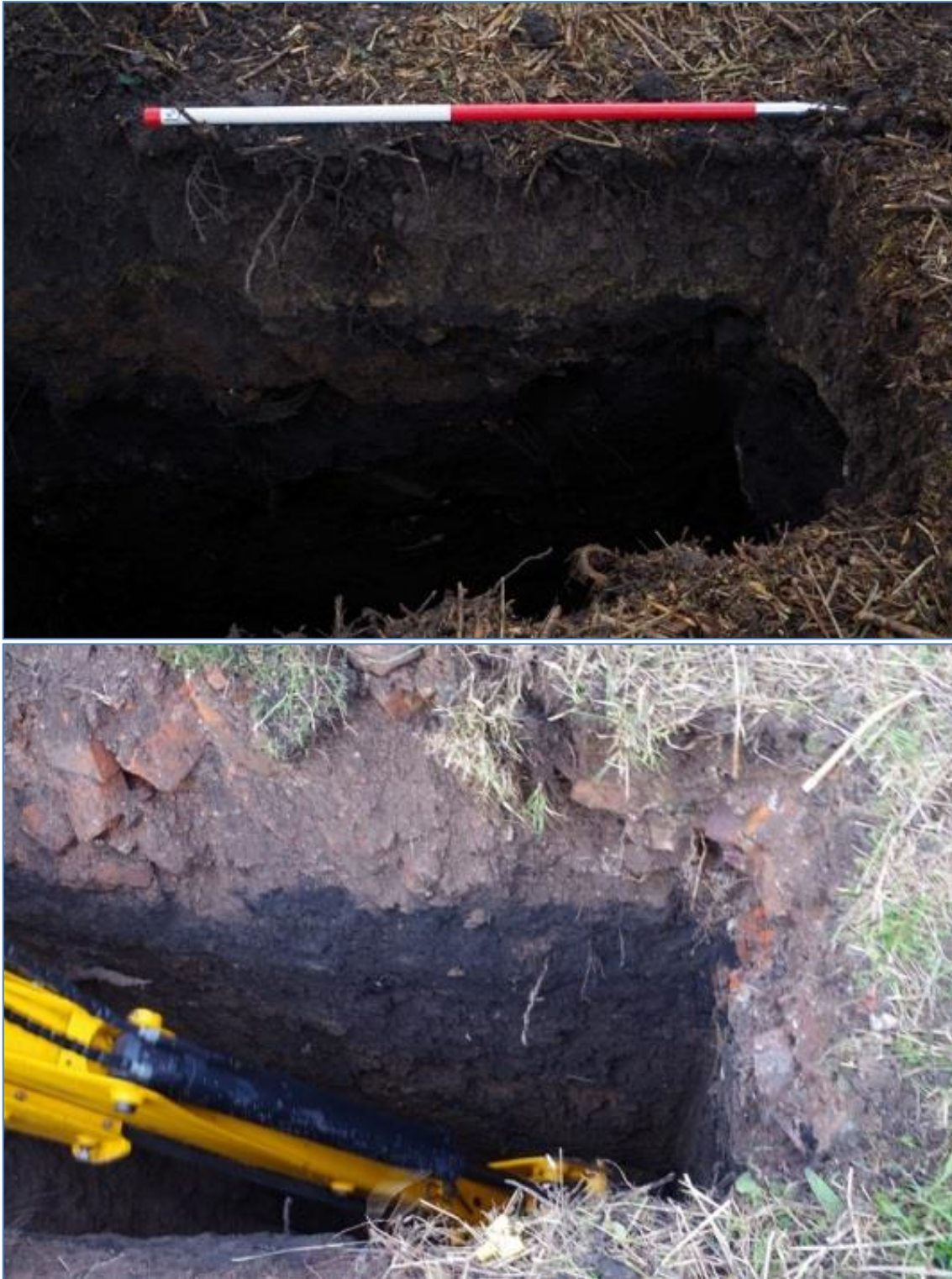
Plate 4 Geotechnical pit 12 showing made ground
