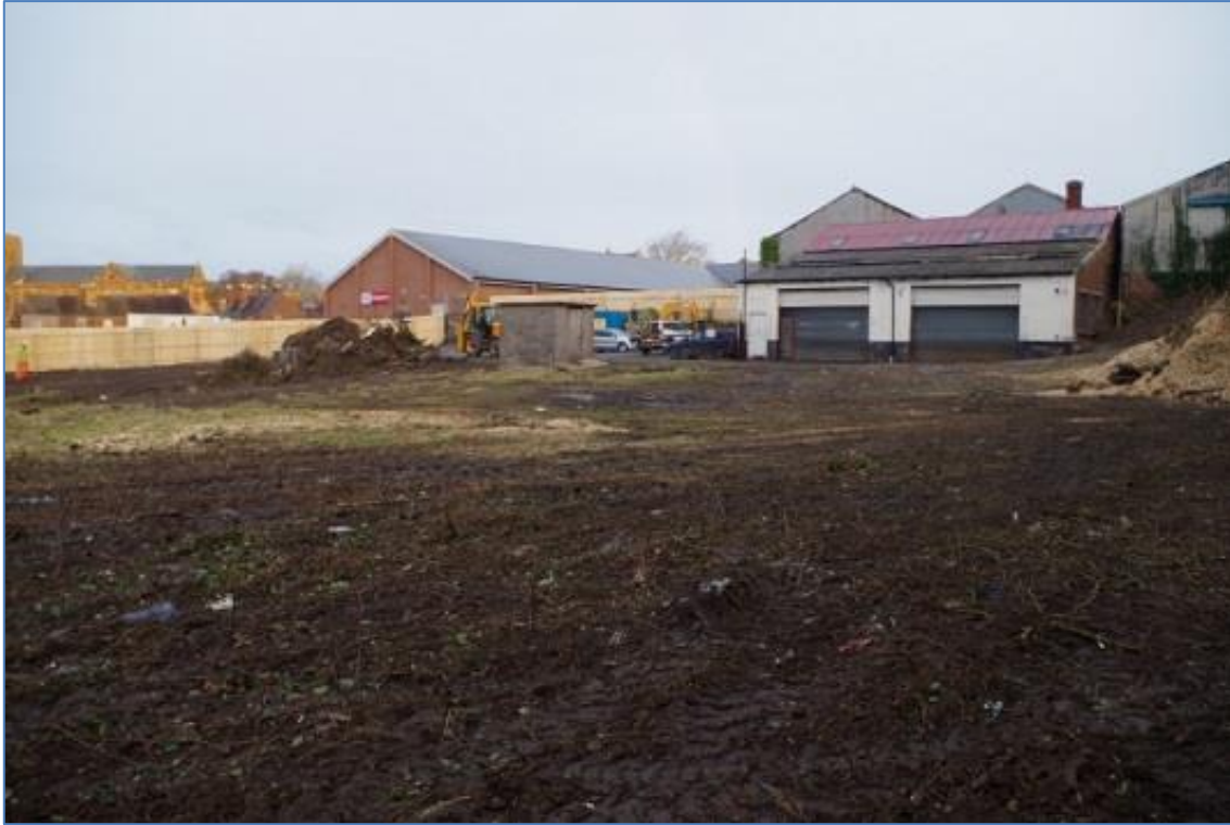
Plate 1 The site prior to excavation from the southeast
