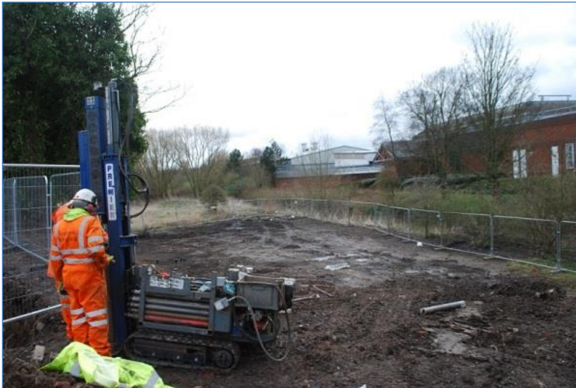
Plate 14 Drilling rig undertaking WS 104, looking towards location of WS105. View southeast
