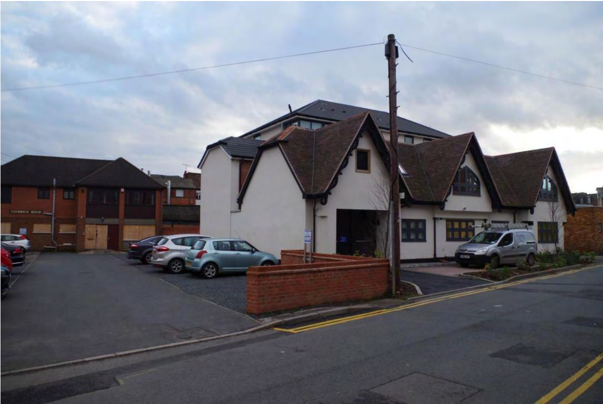
Plate 7 Former Holy Trinity School-Heenan and Froude Club, with Goodrich House in background, looking south-west
