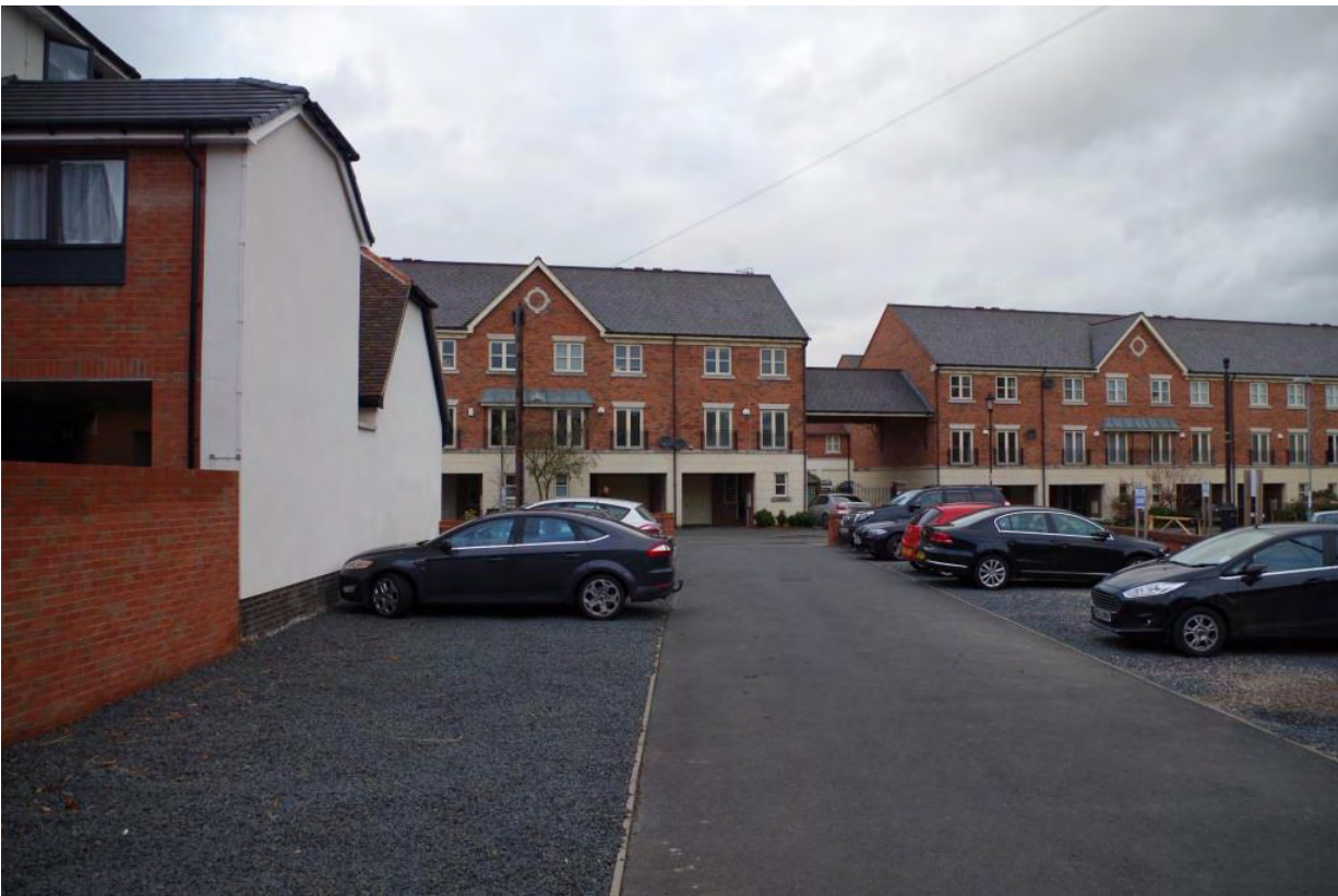
Plate 8 Proposed development area, with former Holy Trinity School house to left, looking north
