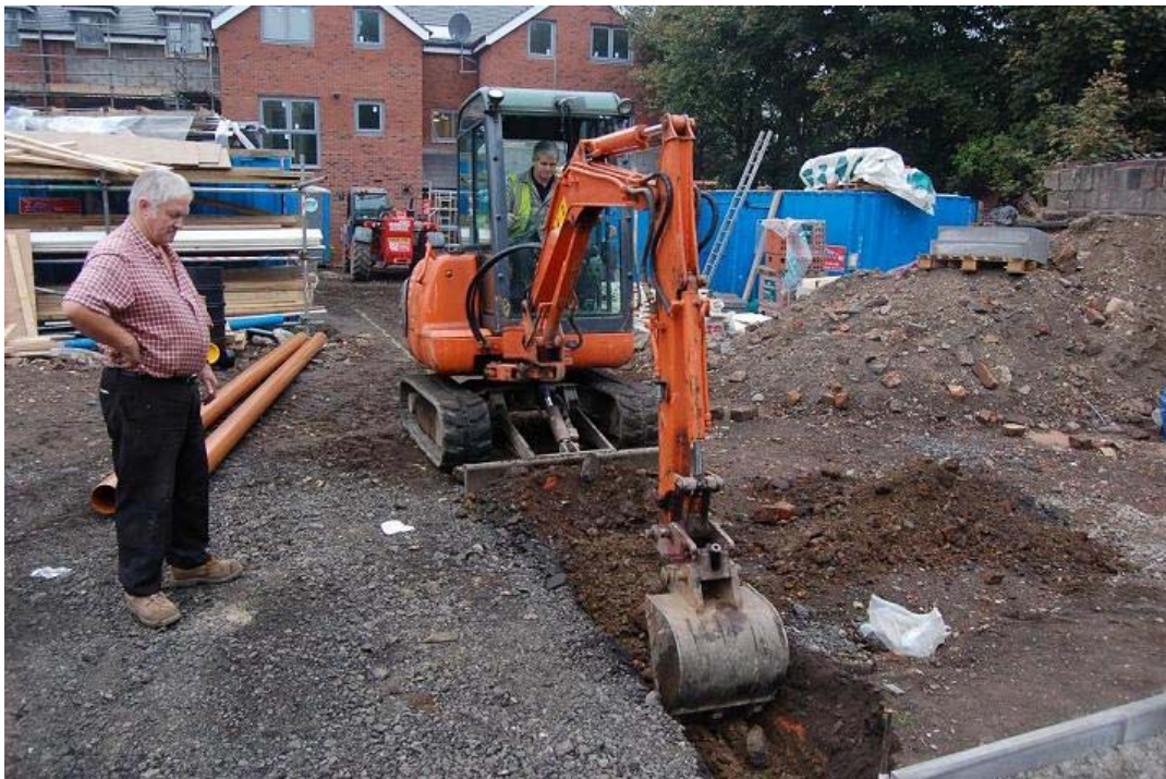
Plate 3: General view from east end of site, view west.
