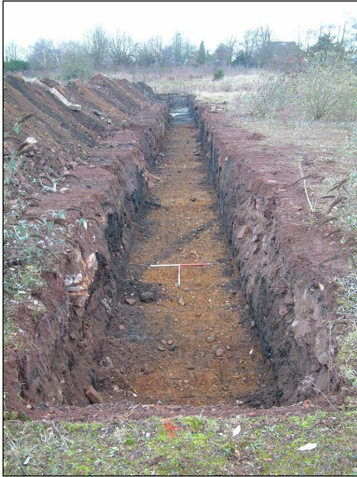
Plate 25 Trench 10 - general shot facing north-west
