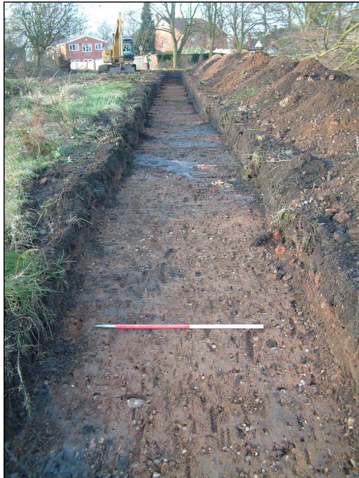
Plate 5: Trench 2 – general shot facing north-west
